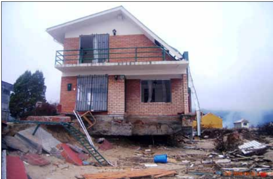
Figure 11. This concrete frame and confined masonry building in Dichato survived the hydrodynamic loads, but suffered substantial foundation scour (photo: G. Chock).
