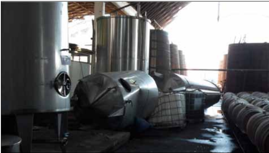
Figure 28. Typical damage to storage tanks in wineries (photo: R. Leon).
