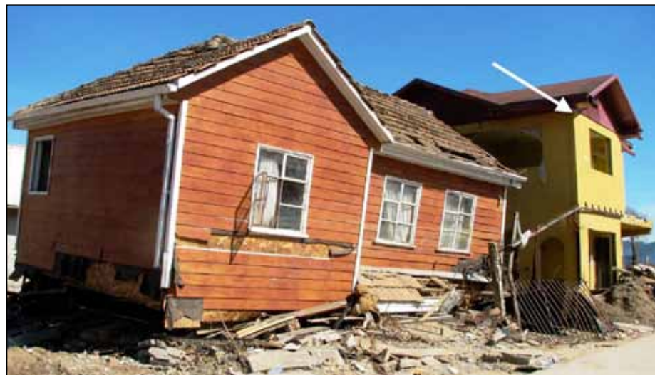
Figure 9. Wood building on left in Dichato was transported from across street and collided with the concrete frame building on the right. Arrow shows water height (photo: L. Dengler).
