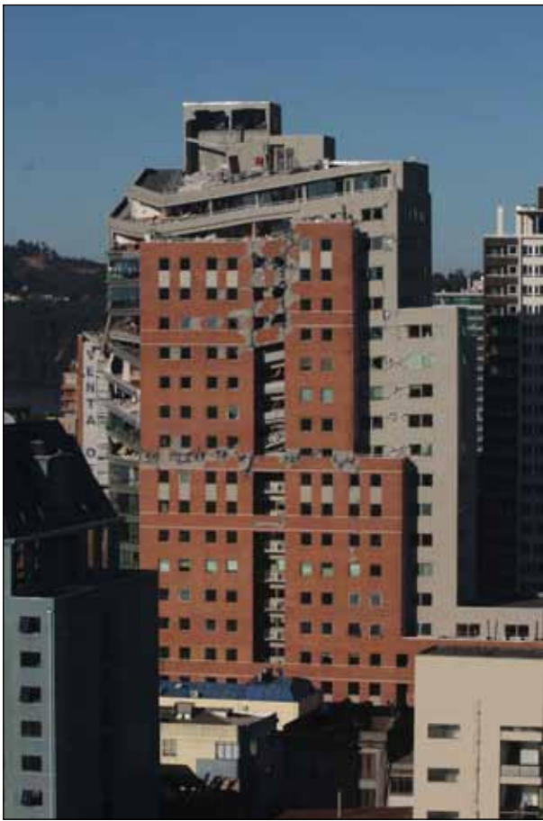
Figure 18. O'Higgins 241 office tower (photo: E. Miranda).
