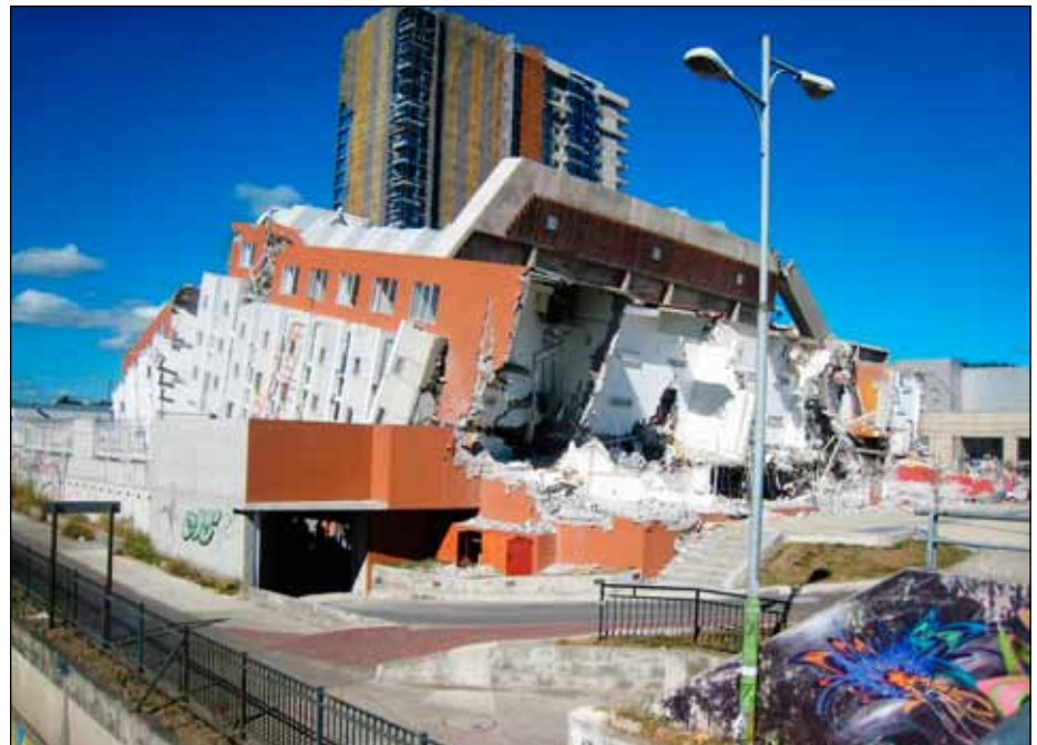
Figure 17. Collapsed Alto Río tower showing underside (photo: J. Maffei).
