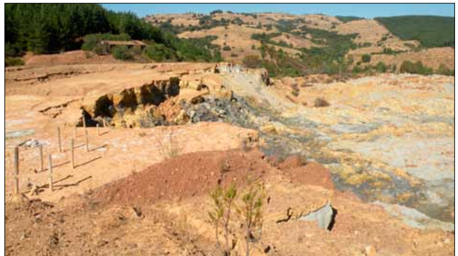
Figure 8. Upper scarp of Failed Tailings Impoundment (photo: GEER 2010).
