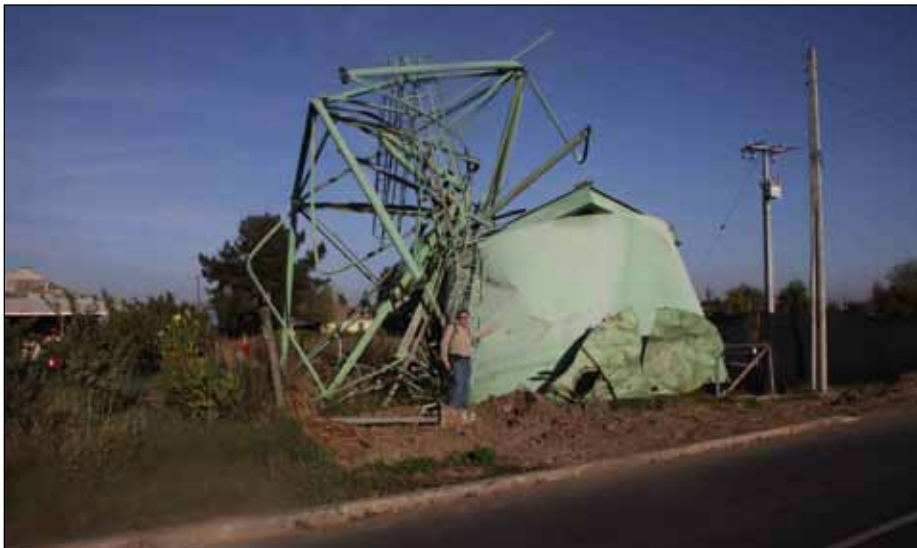
Figure 23. Typical collapsed elevated small steel tank (constructed in 1999) (photo: TCLEE).
