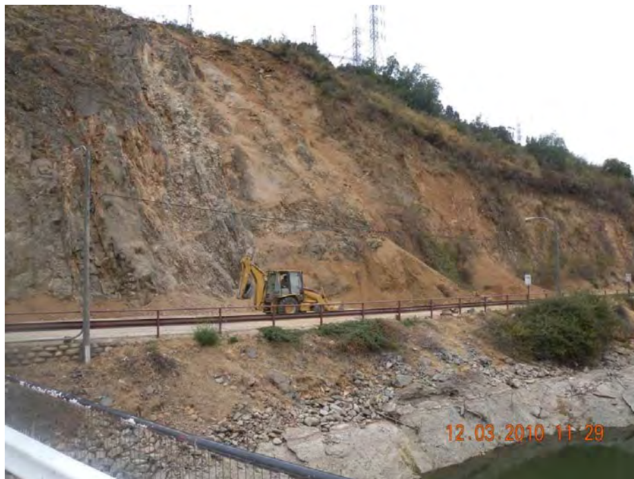
Figure 10.3. Shallow raveling failure of a road cut in weathered and heavily jointed granitic rock at Rapel Dam (34.0407421°S, 71.587153°W).
