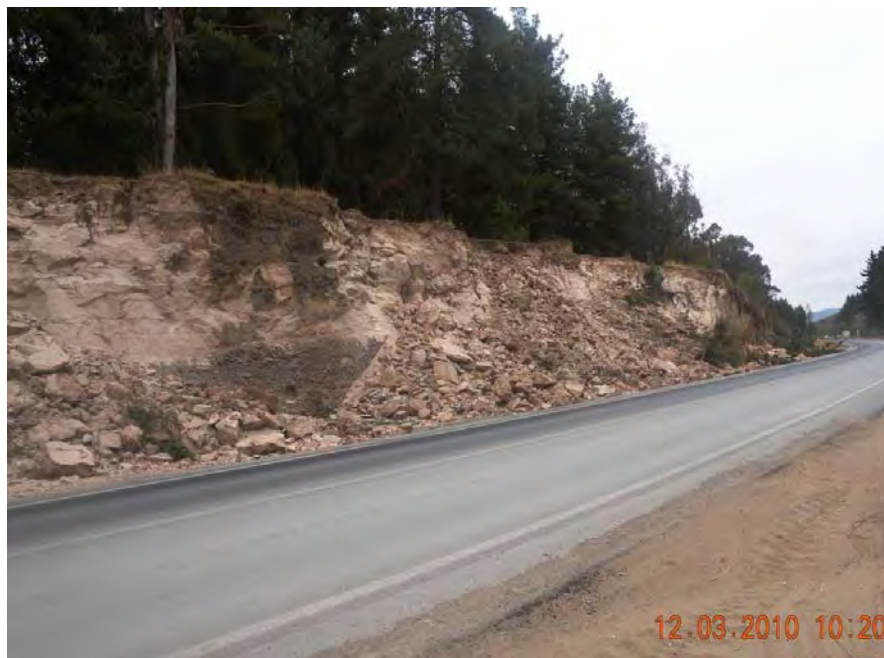
Figure 10.4. Road cut failure in jointed welded tuff north of El Manzano. The height of the cut is about 6 m (20 feet). Picture looking NE (34.144076°S, 71.38000°W).
