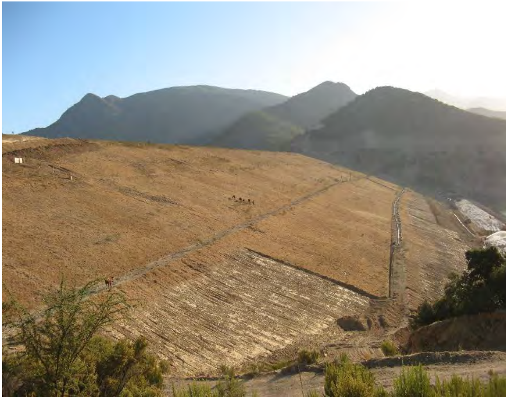
Figure 11.20. March 10, 2010 View of the Downstream Face of the Caren Tailings Dam Showing Progress of Dam Raise Construction (S34.092422°, W71.173250°)
