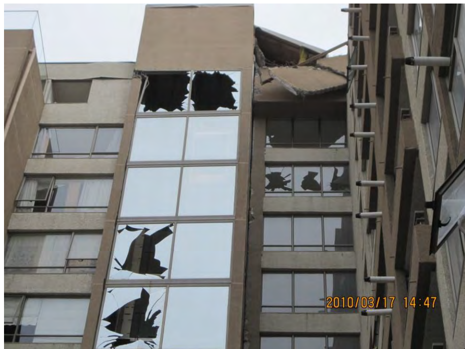
Figure 7.39. Interface between the north and south wings at the upper floors (north wing on right of photograph) showing evidence of minor pounding (view of east side, looking west) (S36.8205°, W73.0619°; 03/17/10).
