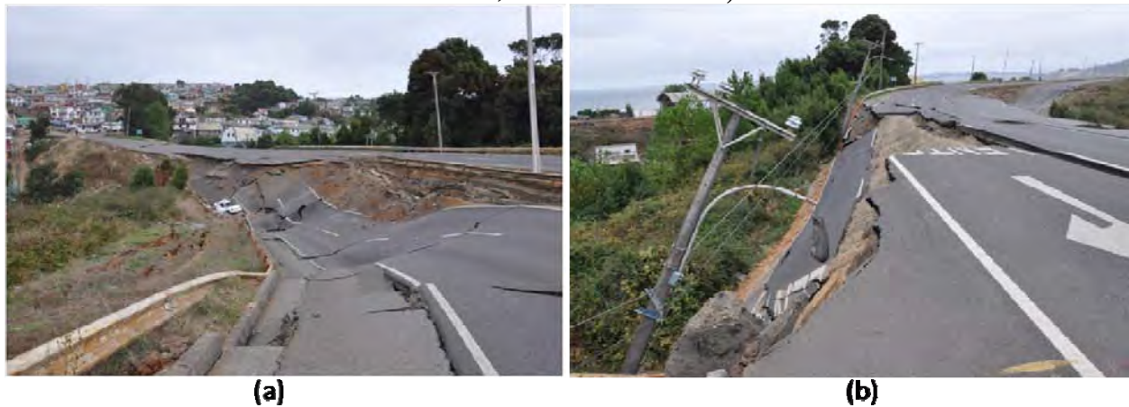
Figure 9.55. Lota (a)View looking south on route 160 showing north bound failure area (S37.0730°,W73.1475°; 1145 hrs on 3/16/2010) (b)View looking north on route 160 showing south bound failure area (S37.0746°, W73.1479°; 1215 hrs on 3/16/2010).
