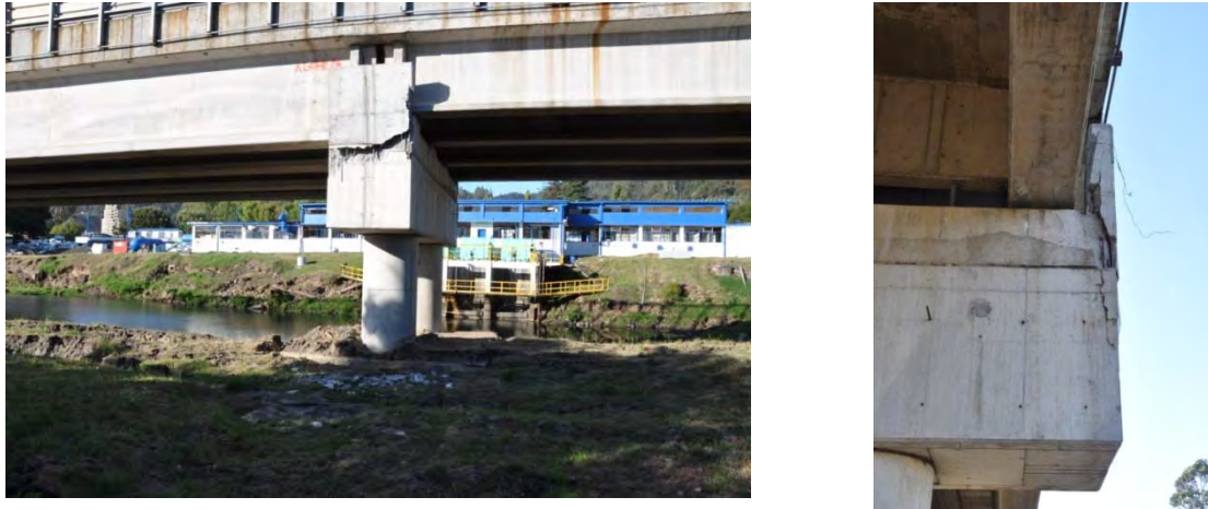
Figure 9.22. Damage to transverse shear keys at bent #3 due to movement of the La Mochita bridge (S36.847405°, W73.055084°; 1830 hrs on 3/15/2010).
