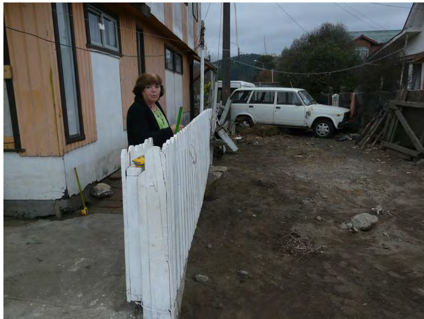
Figure 13.2. Beach-front homes in Laraquete were inundated by the tsunami. At this woman's home, tsunami flow depths reached at least 0.55 m, which transported the white car from the street to the backyard. The tape measure left of the woman indicates the flow depth measured from a water stain on the building (S37.165650° W73.188136, 1915 hrs on 03/16/2010).
