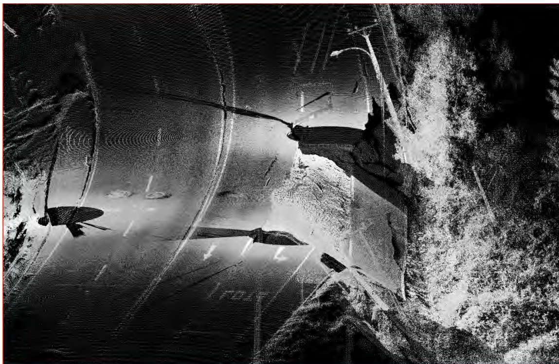
Figure 15.40. Oblique view of route 160 embankment failure along the west side of the merged highways.
