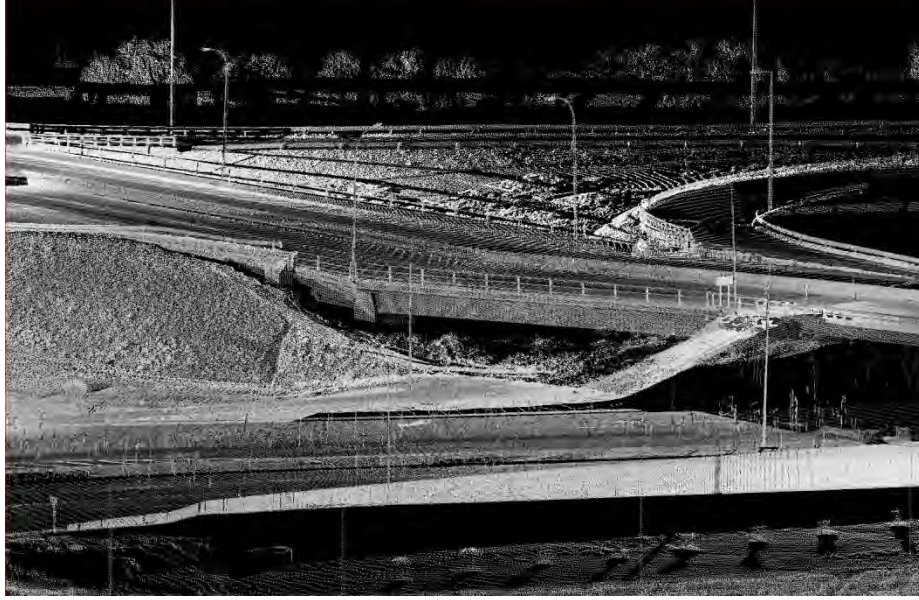
Figure 15.23. Settled bridge pier at the approach embankment of the Juan Pablo II Bridge (S36.815864°; W73.083674°).
