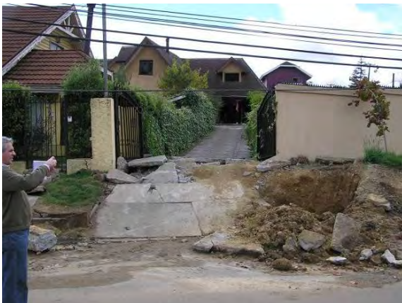
Figure 7.32. View of toe of translation slide in foreground of left photo (also note that the driveway behind the toe is not damaged(S 36.79134°, W 73.05762°; 1150 hrs on 03/17/10), and view of the head scarp of the translation slide at back of driveway in the right photo (S36.79126°, W73.05719°; 1130 hrs on 03/17/10).
