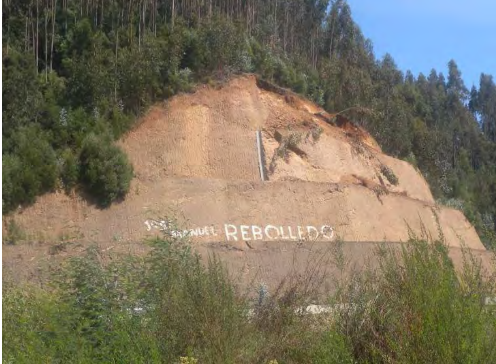
Figure 10.7. Bench failure along a daylighting joint in a road cut in deeply weathered rock south of Lota (37.1213°S, 73.1550°W).
