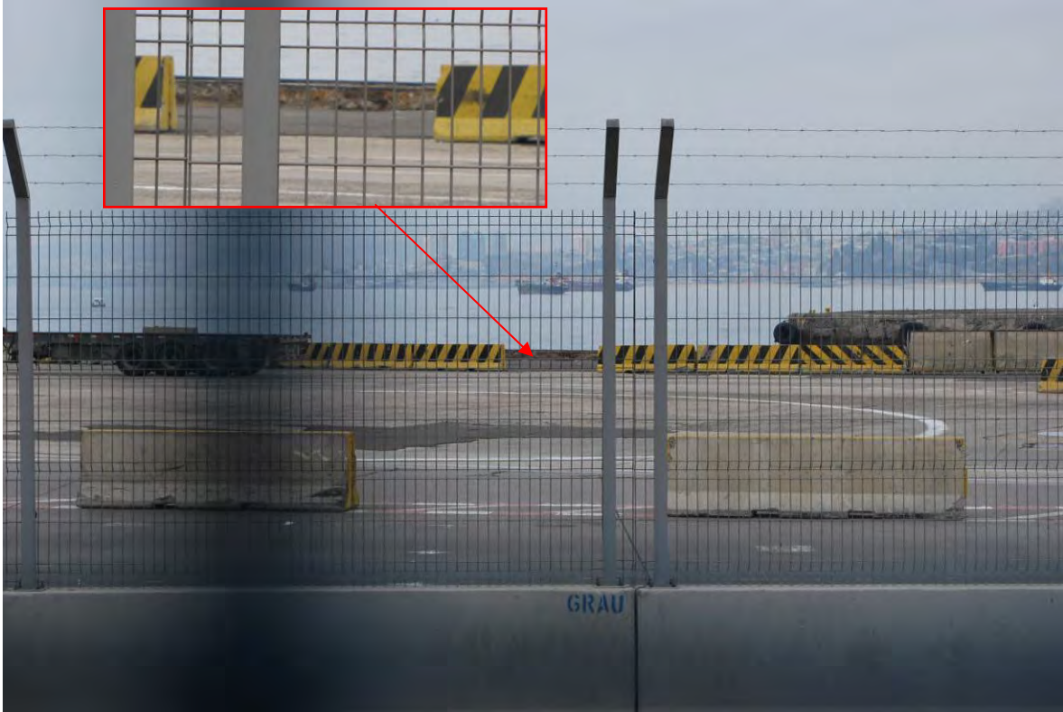
Figure 8.19. Settlement in backfill behind the quay wall at commercial dock of Valparaíso port (S33.034°, W71.627°; 1620 hrs, 03/15/2010).
