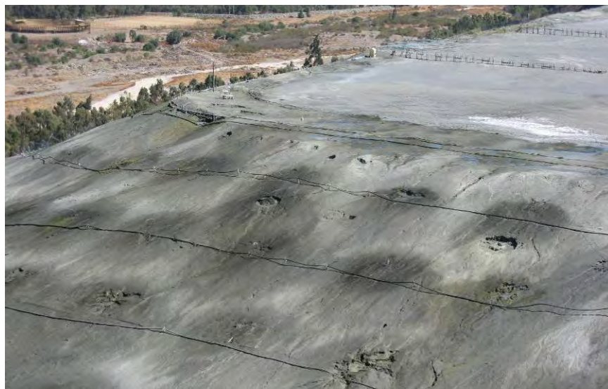
Figure 11.16. March 10, 2010 View of Cabildo Tailings Dam from Helicopter Showing Sprinkler System on Downstream Face (S32.422414°, W71.077165°)
