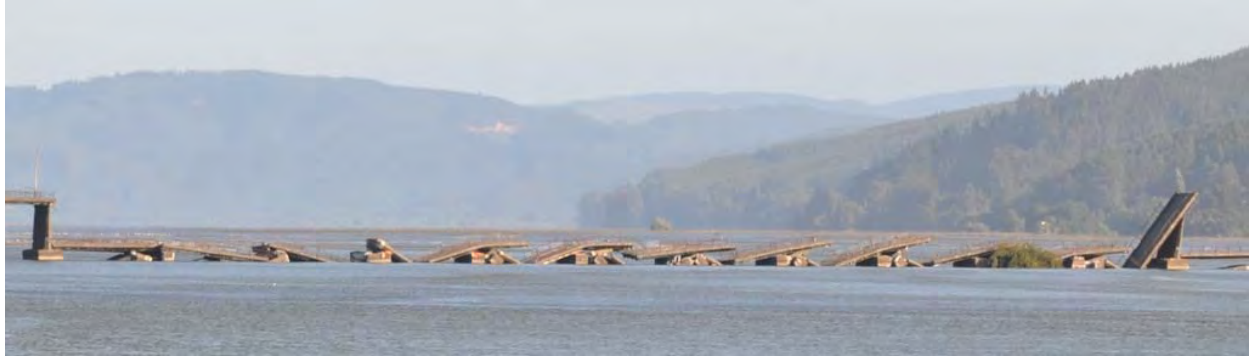
Figure 9.25. Puente Bi-Bio's collapsed slab sections and bridge bents (S36.837968° W73.062896° on 3/15/2010).
