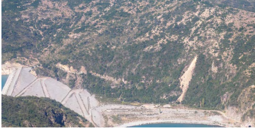
Figure 10.16. Typical shallow disaggregated slide, Colbun Dam (35.668°S, 71.351°W) .
