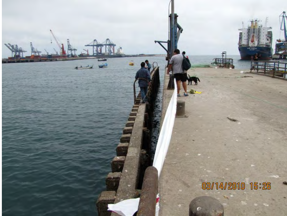
Figure 8.35. Separation from lateral pile screen of wharf structure in San Antonio Port (S33.5817°, W71.6154°; 1526 hrs, 03/14/2010).
