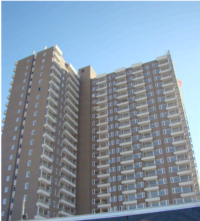
Figure 5.35. 20-story structure adjacent to collapsed (S 36.828083° W 73.060600°, 1910 hrs on 03/16/2010) designed using Soil Type III conditions, and suffering only minor damage.
