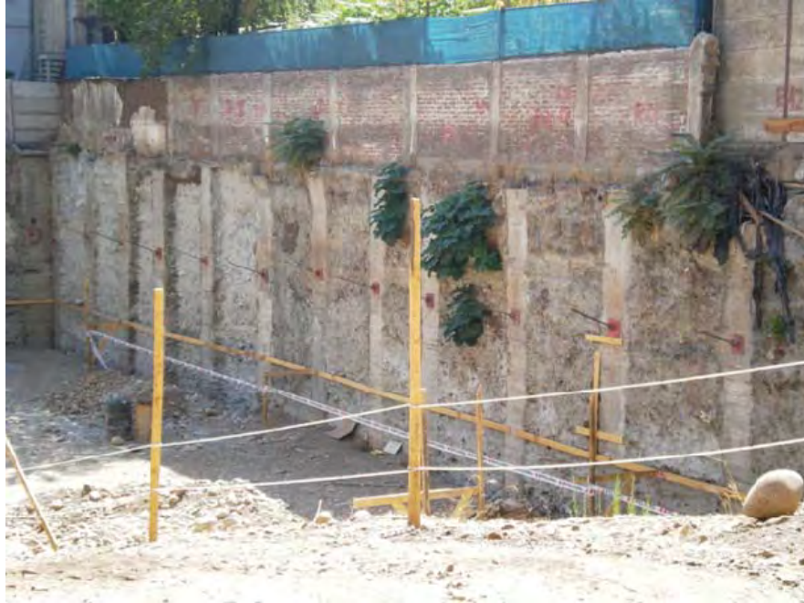
Figure 12.11. Undamaged temporary retaining structure in Santiago.
