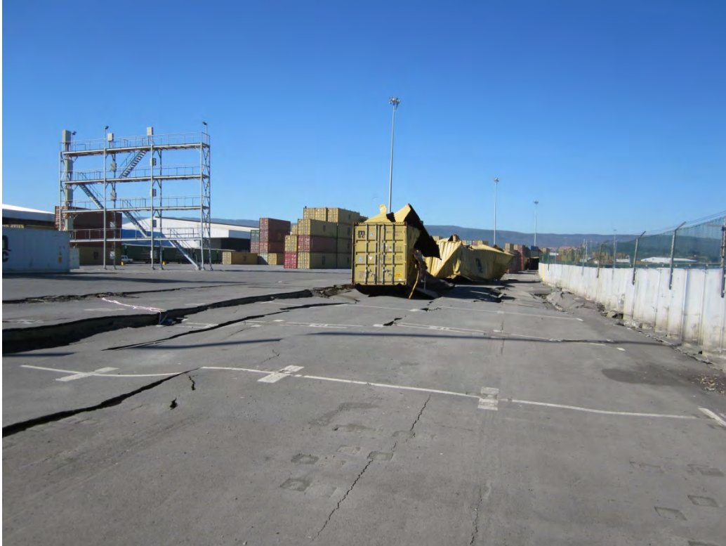
Figure 15.76 Lateral spreading looking south, Port Coronel, April 14, 2010 (37.028874°S, 73.149768°W).
