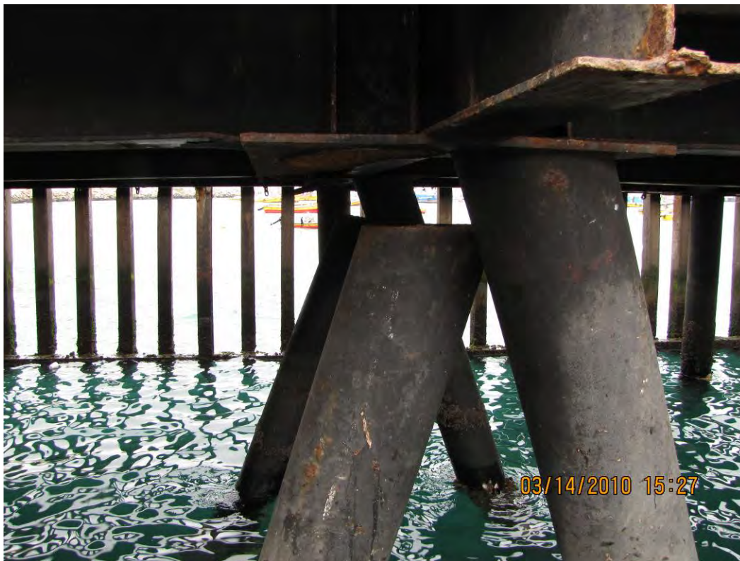
Figure 8.36. Failure of head connection between wharf and raked piles in San Antonio Port (S33.5817°, W71.6154°; 1527 hrs, 03/14/2010).
