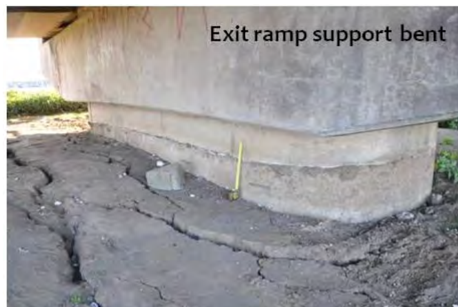
Figure 9.7. Ground settlement surrounding an exit ramp support bent at the Llacolén bridge in Concepción (S36.830380°, W73.067541°, 1901 hrs. on 3/14/2010).
