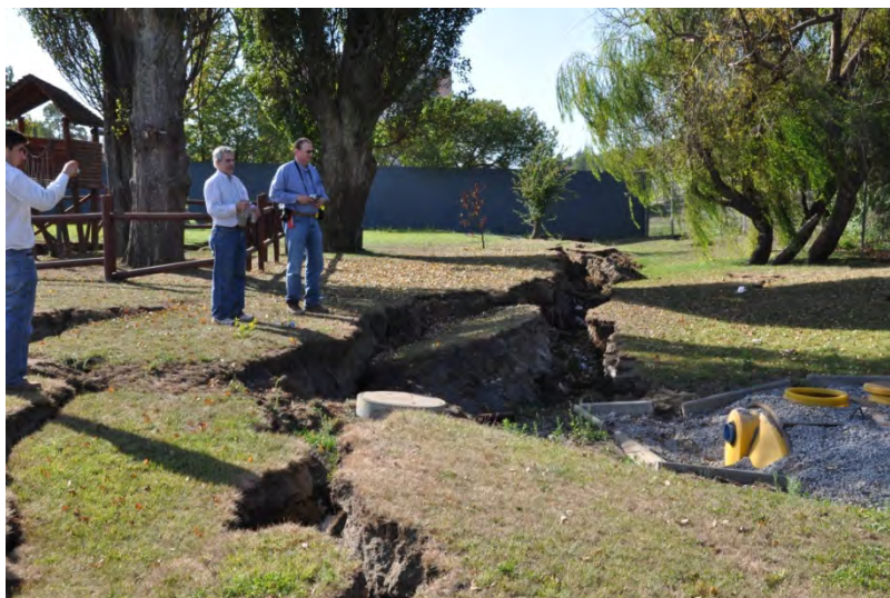
Figure 6.9. Tank uplift in park along west shore of Tres Pasquales lagoon in Concepcion (S36.8152°, W73.0460°; 3/14/2010)
