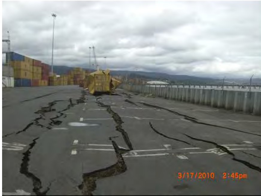
Figure 8.2. Photograph of lateral spread displacements at the Port of Coronel (S37.028680°, W73.150054°; 1445 hrs, 03/17/2010).
