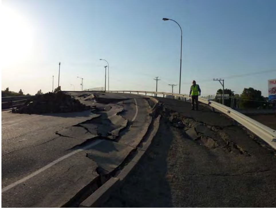
Figure 15.83 Damage to over padded embankment, Ruta 5 Sur overpass embankment, to Retiro at Tucapel Mill, April 15, 2010 (36.051209°S, 71.768005°W).
