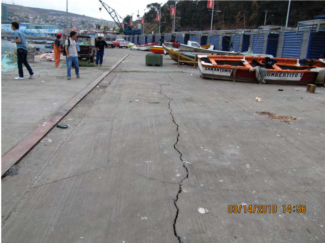
Figure 8.31. Cracks on asphalt pavement behind quay wall in San Antonio Port (S33.5870°, W71.6132°; 1456 hrs, 03/14/2010).
