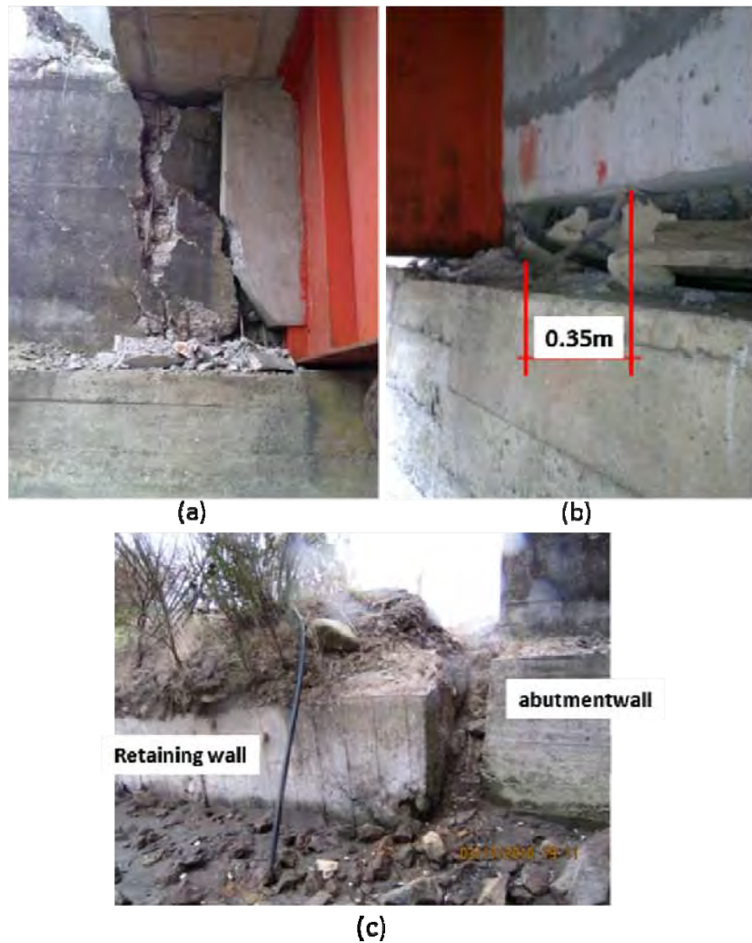
Figure 9.51. Damage to bridge abutment due to lateral spreading of soil around bridge abutment. (a) abutment wall movement relative to beams, (b) deformation of vertical restraining bar due to abutment movement relative to beams, (c) movement of retaining wall relative to abutment. (S37.254345°, W73.437021°; 1911 hrs on 3/17/2010)
