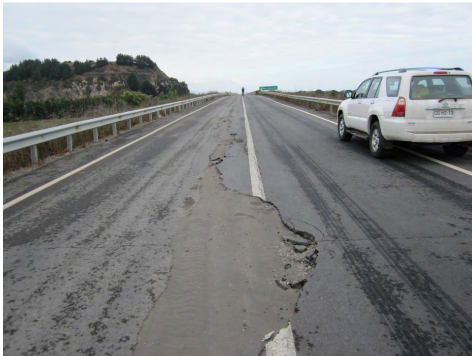
Figure 15.67 Cracking and transverse movement (60 cm on each side) of embankment due to liquefaction of underlying soil, north abutment of the bridge, Puente Mataquito, 35.050712°S, 72.162258°W, April 16, 2010.
