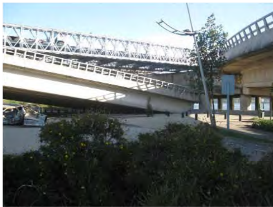
Figure 9.5. Deck unseating at Llacolén bridge in Concepción. (note the temporary deck supporting approach traffic). View South ( S36.829707^\circ , W73.068220^\circ , 1809 hrs on 3/14/2010) and (b) view north ( S36.830380^\circ , W73.067541^\circ , 1911 hrs on 3/14/2010).
