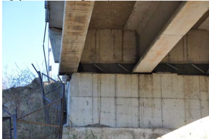
Figure 9.20. Transverse shift of deck relative to south abutment at the La Mochita bridge (S36.847547°, W73.054876°; 1834 hrs on 3/15/2010).
