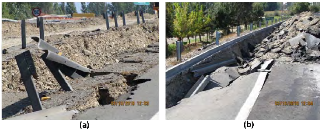
Figure 9.60. Highway 5 failure near Paine; (a)shoulder settlement due to poorly compacted soil (S33.864897° W70.742222° 1203 hrs on 3/16/2010), and (b) road failure due to poorly compacted soil (S33.864897° W70.742222°; 1204 hrs on 03/16/2010)
