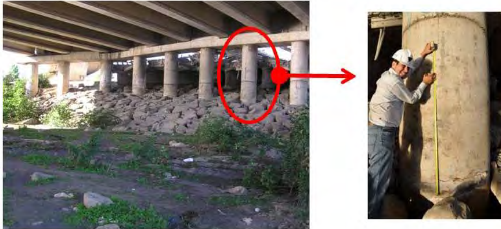
Figure 9.6. Substructure of the north approach at the damaged Llacolén bridge in Concepción showing the unseated deck in the foreground. Flexural cracking of the column supports was observed at ground level and extending to the construction joint (2-2.5m above ground)
