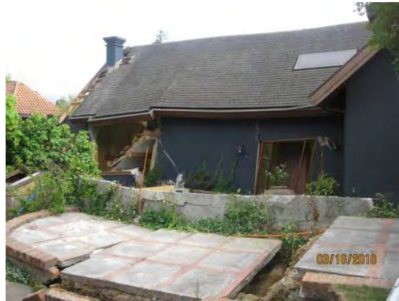
Figure 7.31. View of extension zone in open field behind apartment building (left photo(S36.79126°, W 73.05714°; 1120 hrs on 03/17/10), and view of damage to a home due to ground extension across its foundation (right photo, S36.79108°, W73.05728°; 1200 hrs on 3/17/2010).
