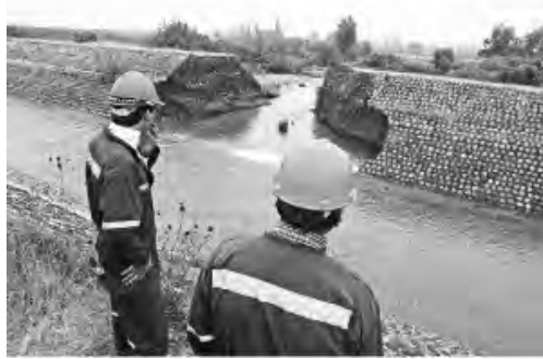
Figure 11.35. Earthen levee breach west of Colbun ( S35.698672^\circ , W71.487294^\circ ; photograph taken by Mr. Juan Carlos Romo of the El Mercurio on March 12, 2010; http://diario.elmercurio.cl ).
