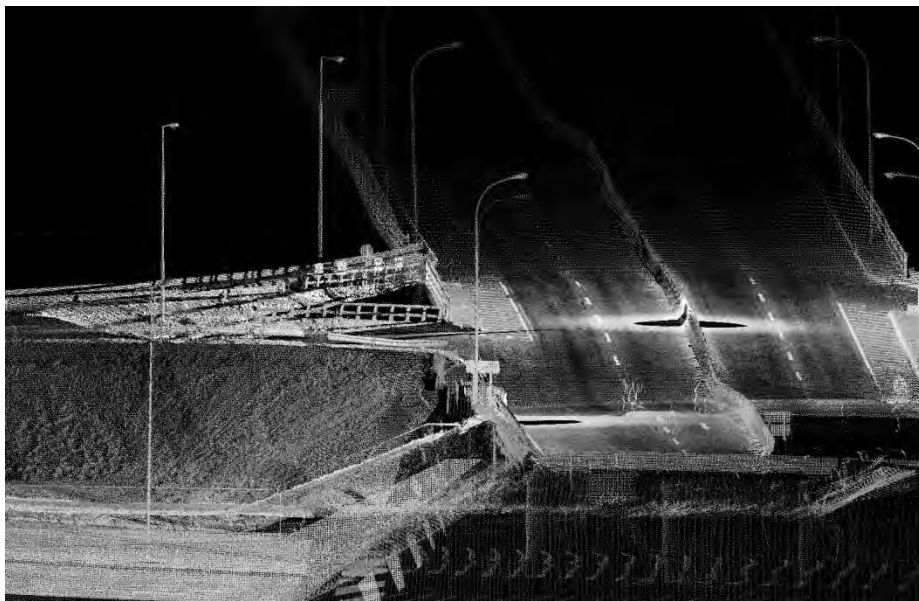
Figure 15.24. Distorted bridge centerline guard wall and settle deck above the north east approach embankment.
