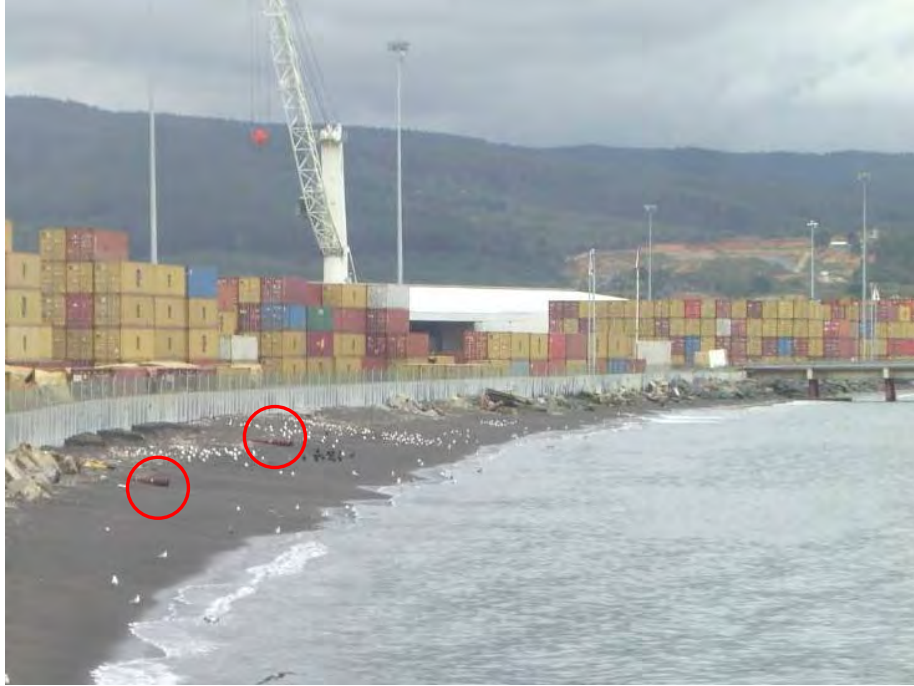
Figure 8.6. Pipelines running transverse to sheet-pile wall which were subjected to longitudinal strain due to lateral spreading (S37.028680°, W73.150054°; 1520 hrs, 03/17/2010).
