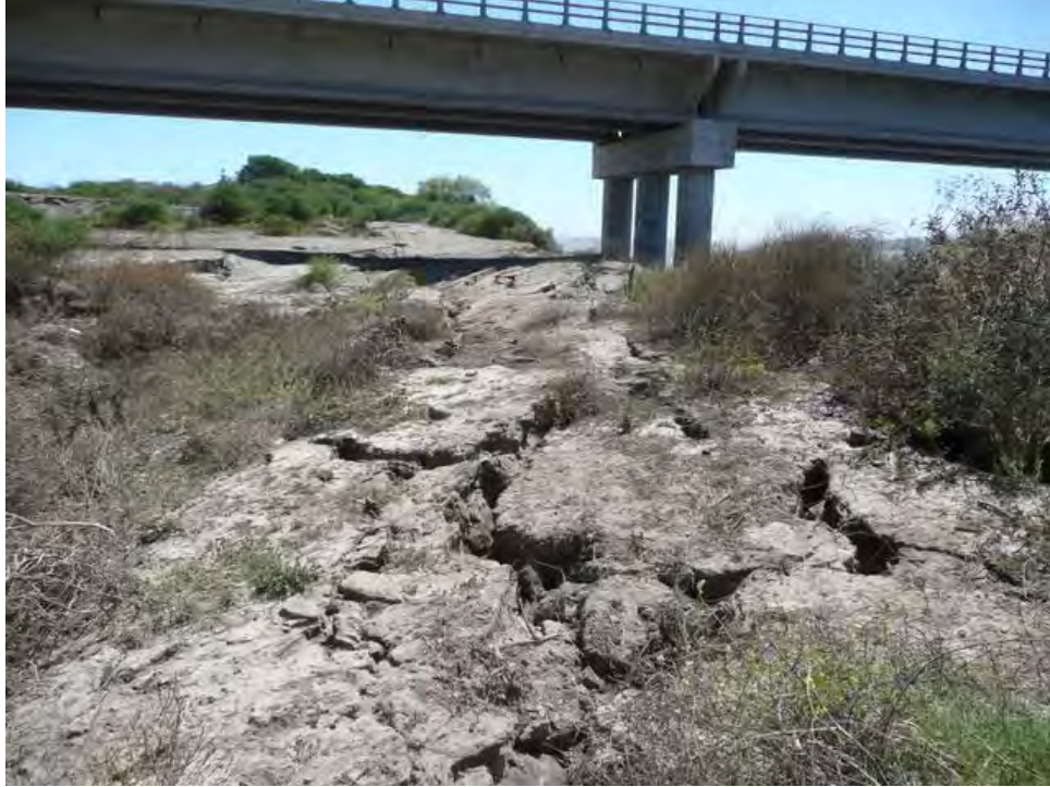
Figure 6.13. Lateral spreading at the south landing of the Mataquito bridge along the coastal highway (S3505078°, W72.16240°, 11:00, 3/8/2010).
