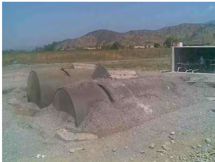
Figure 6.19. Tanks buoyed above the ground surface when the higher unit weight soil fluidized due to excess pore pressure generation. This occurred near San Fernando (~S34.5898°, ~W70.9890°)
