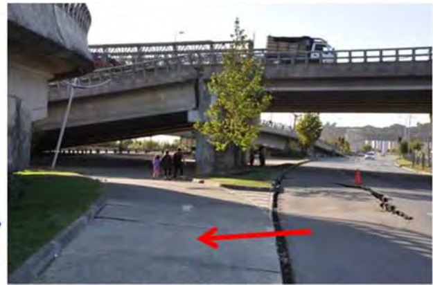
Figure 9.5. Deck unseating at Llacolén bridge in Concepción. (note the temporary deck supporting approach traffic). View South ( S36.829707^\circ , W73.068220^\circ , 1809 hrs on 3/14/2010) and (b) view north ( S36.830380^\circ , W73.067541^\circ , 1911 hrs on 3/14/2010).
