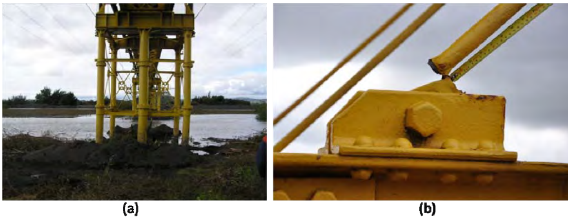
Figure 9.26. Bio Bio Railroad crossing (a) Pillars move and rotated during earthquake (b) Detail of broken crossbar, (S36.836075° W73.086969°; 1717 hrs on 3/17/2010)
