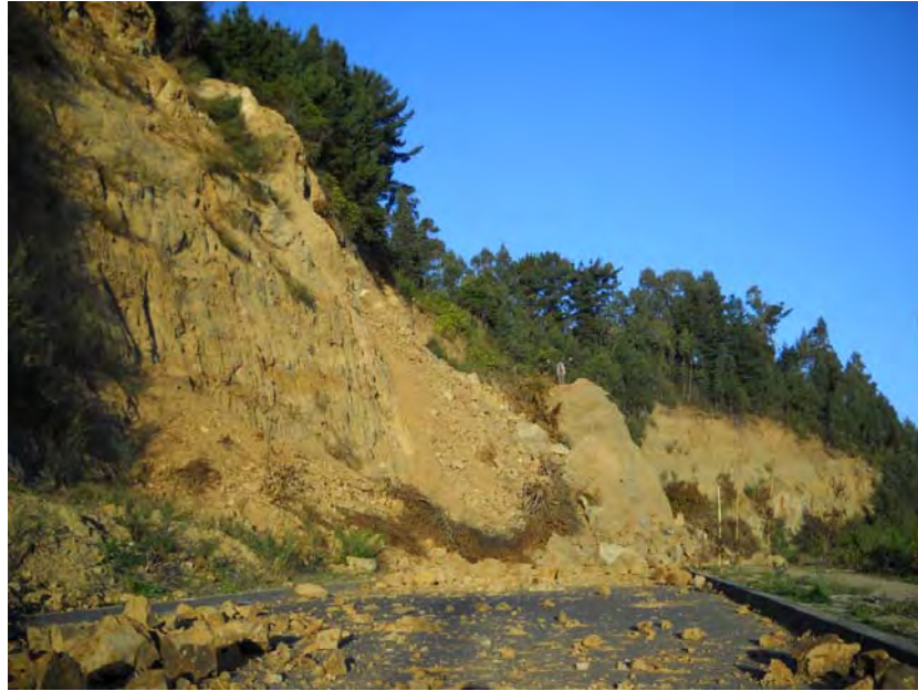
Figure 10.14. Landslide in a road cut in Cocholgue, north of Tome (36.595 S, 72.974 W). Photo and details courtesy of J.M. Lopez.
