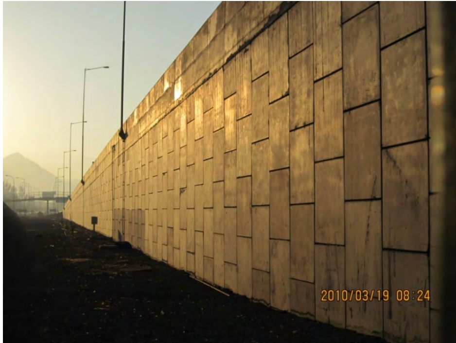
Figure 9.37. Retaining walls and mechanically-stabilized-embankment (MSE) walls appeared to perform well in the Quilicura area of Santiago (S33.366137, W70.688913; 824 hrs on 3/19/2010)
