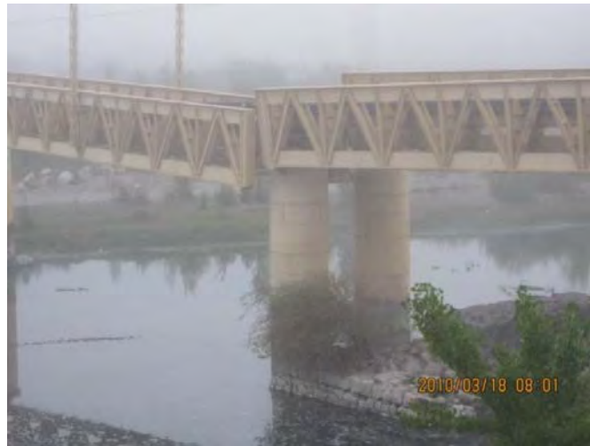
Figure 9.63. Unseated railway bridge span near Longavi from excessive transverse movement (S36.004136, W71.726193, 0801 hrs on 3/18/2010)
