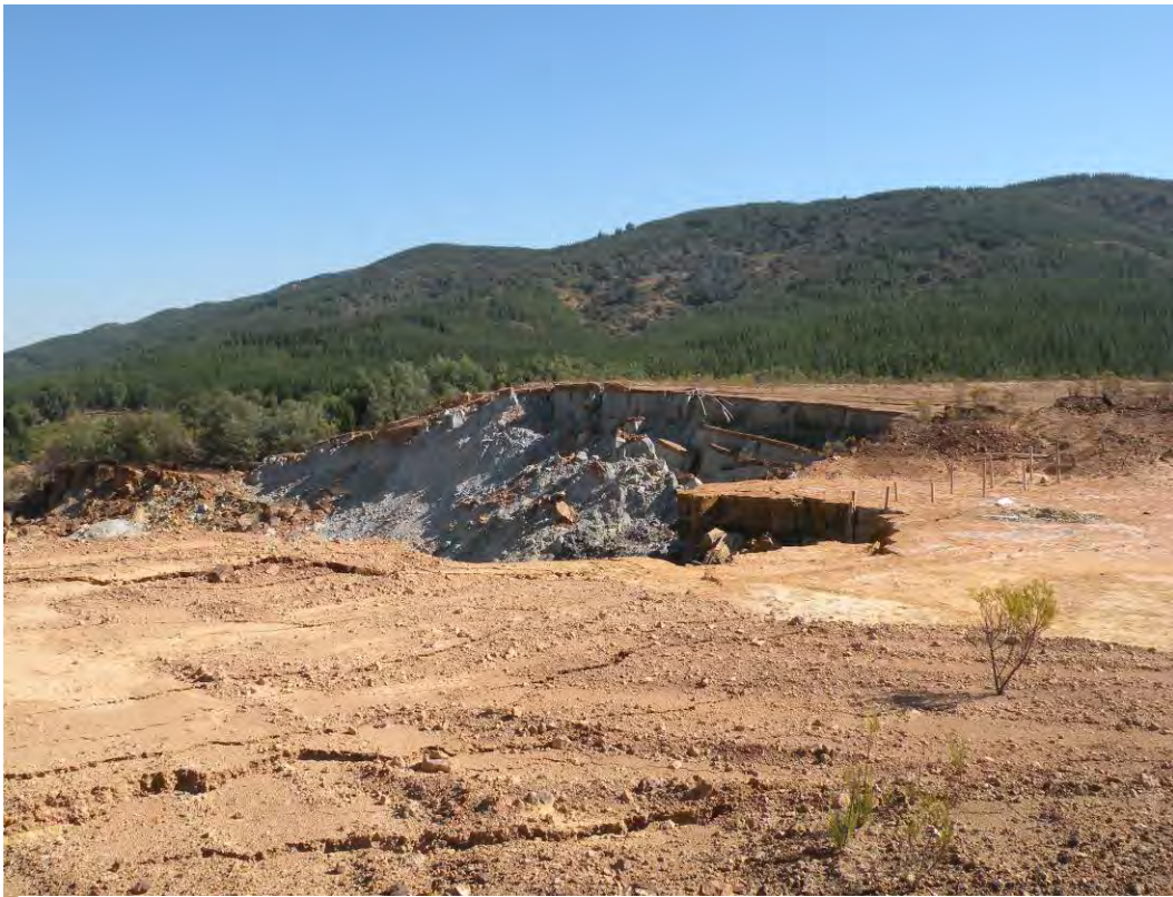
Figure 11.23. March 11, 2010. Upper Scarp of Failed Tailings Impoundment Looking Southwest ( 35.184679^{\circ} S, 71.759410^{\circ} W)
