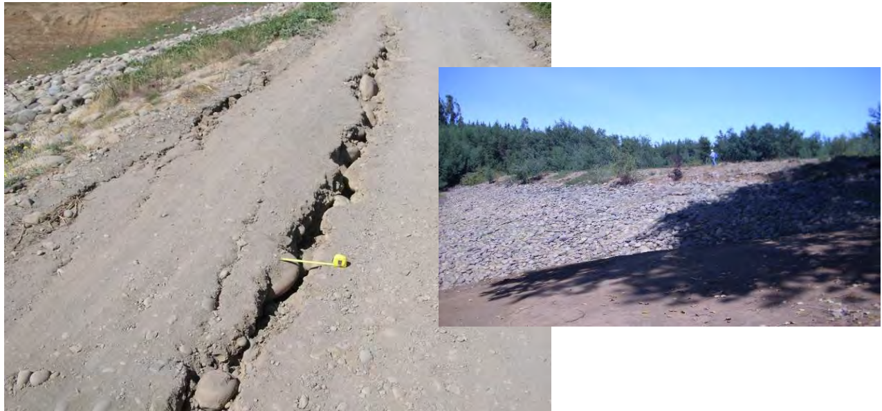
Figure 11.5. March 10, 2010. Cracking of Crest of Small Dam South of Main Coihueuco Dam (S36.645411°, W71.800212°).
