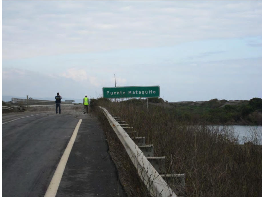
Figure 15.66 Settlement of the north abutment of the bridge, 70 cm offset at the bridge deck, Puente Mataquito, 35.050712°S, 72.162258°W, April 16, 2010.
