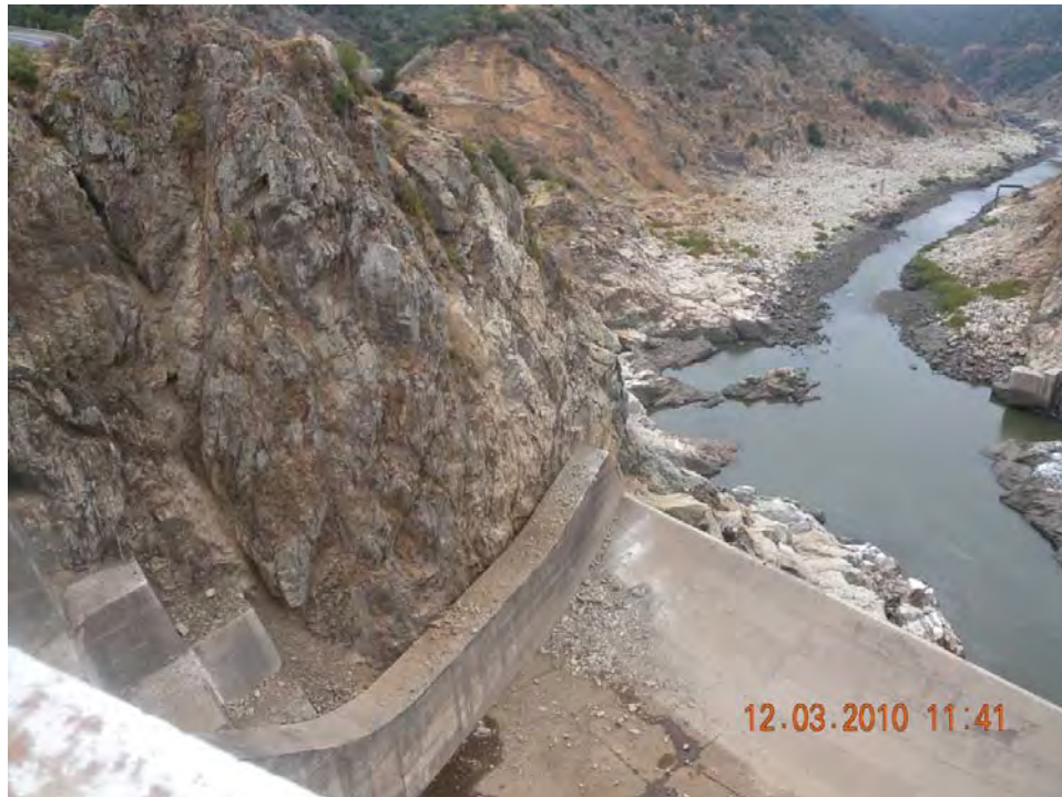
Figure 10.2. Rock fall from the downstream left abutment of Rapel Dam (34.04167°S, 71.59263°W).
