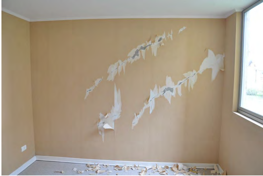
Figure 7.25 Damage to ground floor shear walls of the Montt building (S36.790737°, W73.080901°; 1545 hrs on 3/17/2010)
