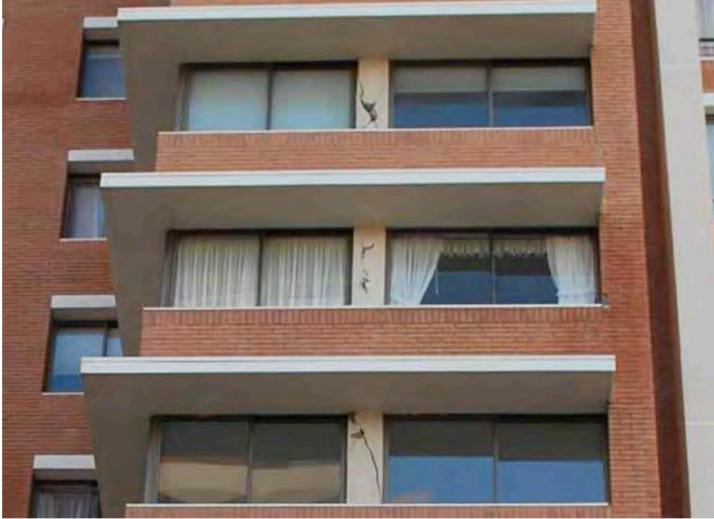
Figure 5.25. Site DA020 (S 33.018678° W 71.556288°, 1953 hrs on 03/14/2010). Diagonal cracks of columns in all the floors of 19-story building.
