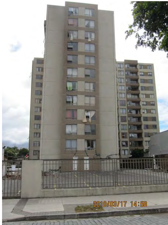
Figure 7.36. Elevation view of 1343 Salas, looking north. North wing is in the background, while the south wing is in the foreground. Note shear and horizontal cracks in the wall on first floor of south wing. (S36.8205°, W73.0619°; 1458 hrs on 03/17/10).
