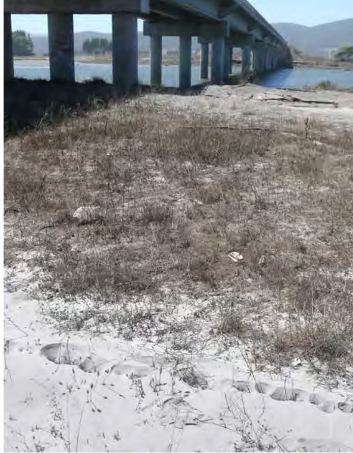
Figure 6.15. Ejecta in the foreground and lateral spreading cracks in the back ground along the south landing of the Mataquito bridge (S3505078°, W72.16240°, 11:00, 3/8/2010).
