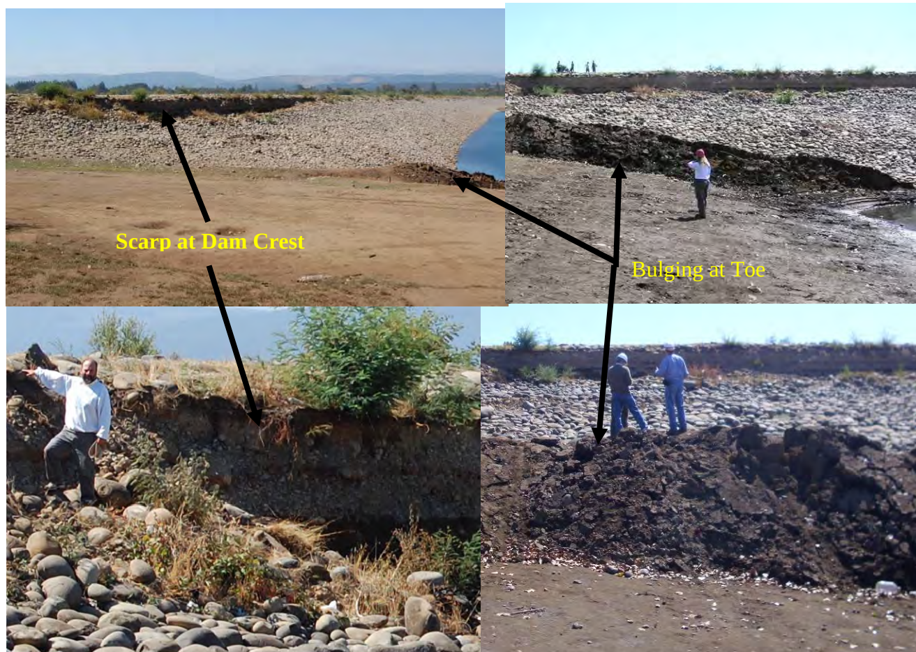
Figure 11.2. March 10, 2010. Slump of the upstream face of Coihueco Dam near the left abutment (S36.637166°, W71.797530°)
