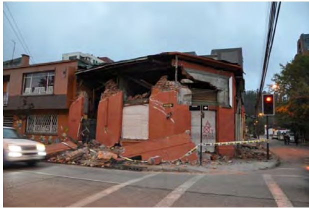
Figure 9.28. Typical construction type and observed damage within the city of Talca (S36.832375,W73.055439; 2016 hrs on 3/17/2010).
