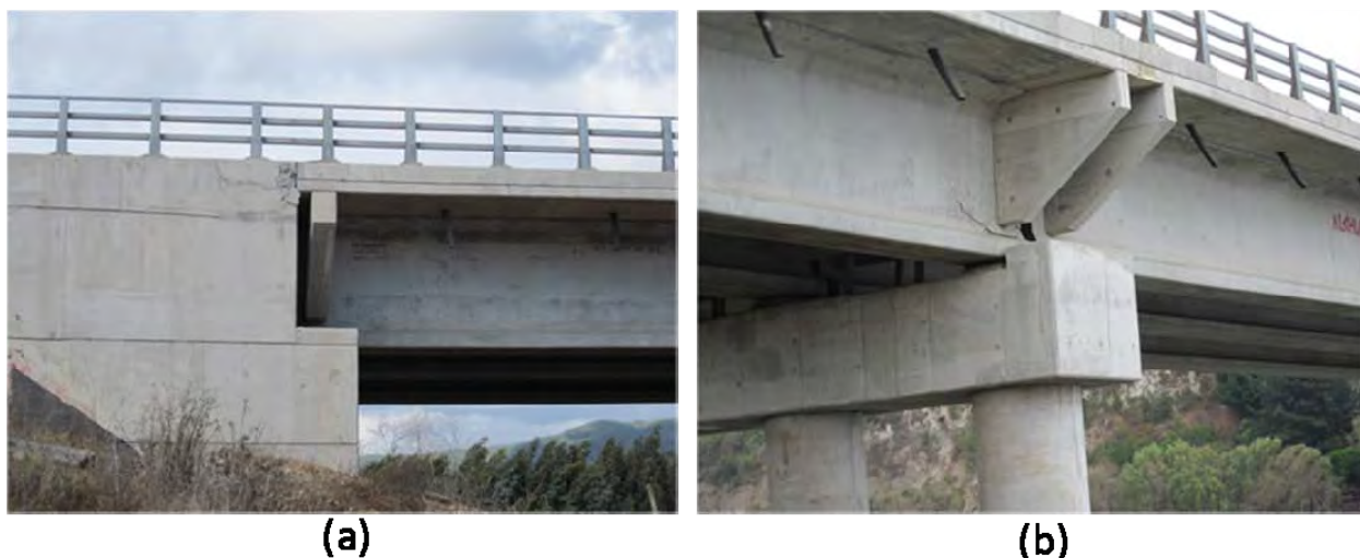
Figure 9.43 (a) North abutment shoved into bridge deck due to lateral spreading, Puente Mataquito, S35.050712°,W72.162258°, April 16, 2010, (b) Shearing of bridge girder, North abutment of bridge, Puente Mataquito, S35.050712°,W72.162258°, April 16, 2010.
