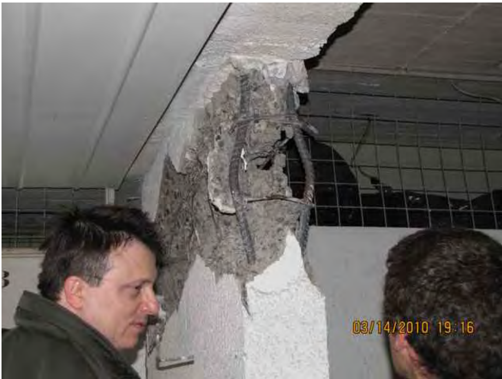
Figure 5.24. Site DA019 ( S33.016045^{\circ} W 71.551990^{\circ} , 1916 hrs on 03/14/2010). Damaged 10-story building. Lack of confinement beam-column joints and low quality concrete.
