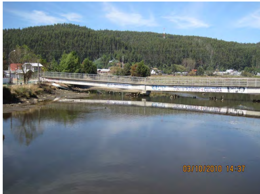
Figure 9.47. Pedestrian Laraquete Bridge showing large settlement of middle pier (S37.166742° W73.184384°; 1437 hrs on 3/10/2010).
