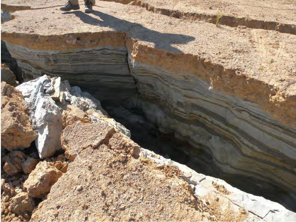
Figure 11.29. March 11, 2010. Gravelly Cover Layer Over Oxidized and Unsaturated Tailings (35.184679° S, 71.759410° W)
