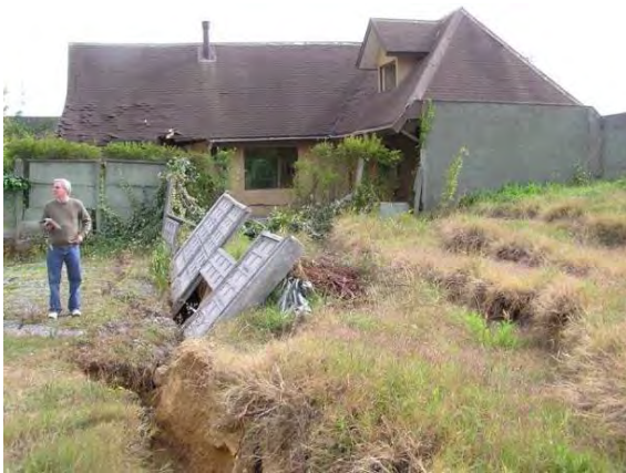
Figure 7.31. View of extension zone in open field behind apartment building (left photo(S36.79126°, W 73.05714°; 1120 hrs on 03/17/10), and view of damage to a home due to ground extension across its foundation (right photo, S36.79108°, W73.05728°; 1200 hrs on 3/17/2010).
