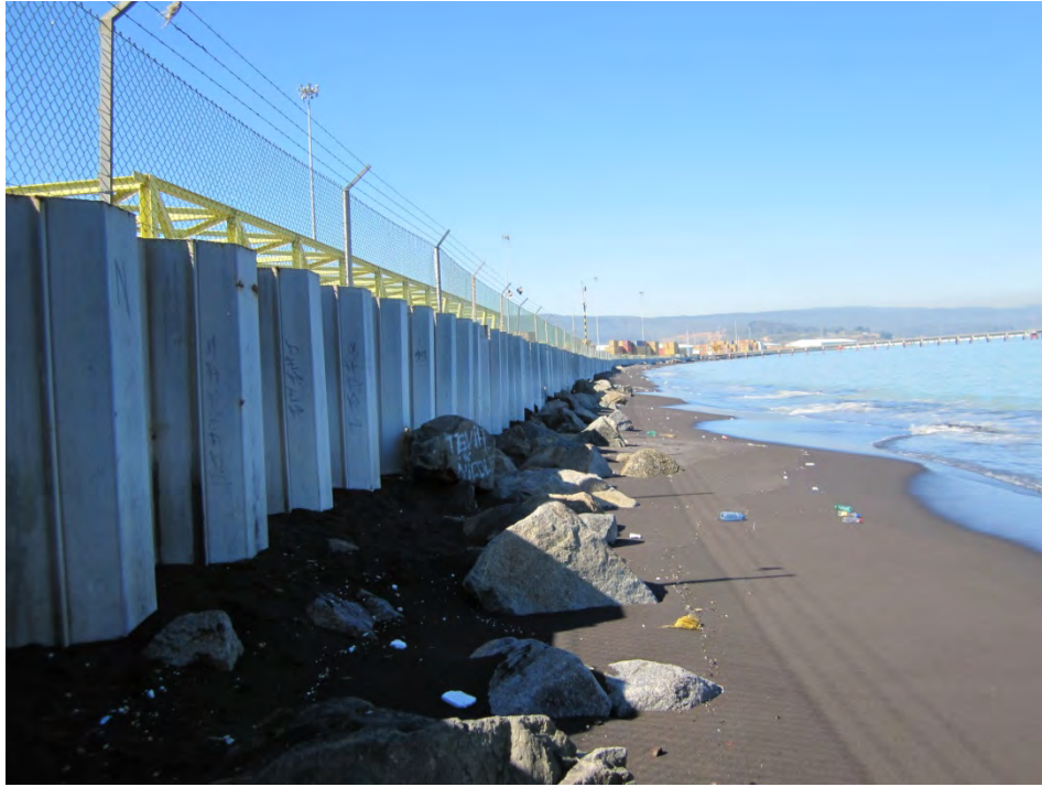
Figure 15.78 Seaside view of the sheet pile wall that experienced lateral spreading, Port Coronel, April 14, 2010 (37.028874°S, 73.149768°W).
