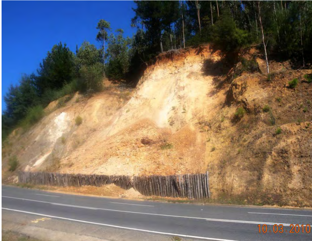
Figure 10.5. Shallow failure in a road cut in highly weathered bedrock (37.256493°S, 72.96018°W, looking SW).
