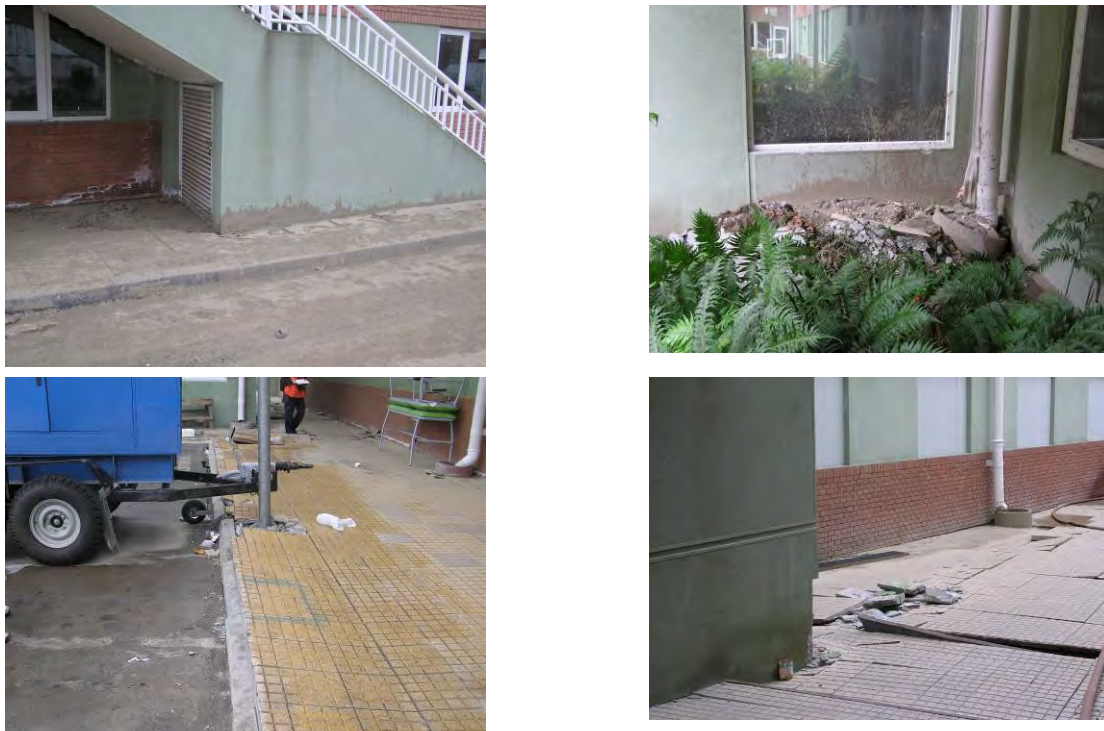
Figure 7.7. Sediment ejecta observed around hospital wings; (a) ejecta observed along exterior staircase of Wing 1D (S37.47358°, W73.34890°), (b) ejecta observed along exterior of Wing 1C (S37.47342°, W73.34829°), (c) ejecta observed along south side of Wing 1D(S37.47375°, W73.34851°), and ejecta observed along east side of Wing 2G (S37.47343°, W73.34788°).
