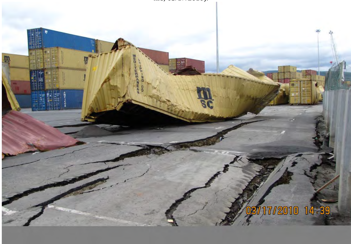
Figure 8.2. Photograph of lateral spread displacements at the Port of Coronel (S37.028680°, W73.150054°; 1445 hrs, 03/17/2010).
