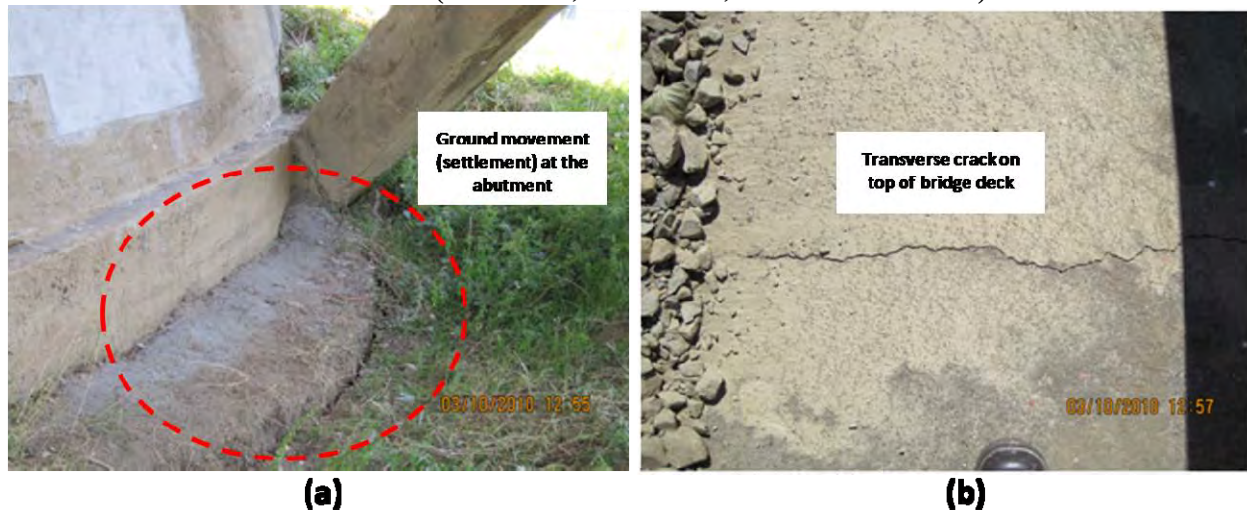
Figure 9.45. Patagual Bridge-(a) Ground movement at the abutment (b) Sidewalk crack in the transverse direction on the top of the bridge deck(S37.111325, W72.987583, 1257 hrs on 3/10/2010).
