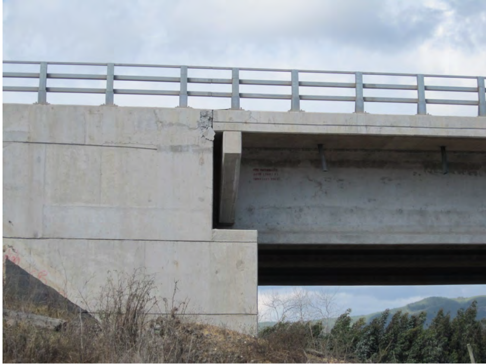
Figure 15.70 North abutment shoved into bridge deck due to lateral spreading, Puente Mataquito, 35.050712°S, 72.162258°W, April 16, 2010.
