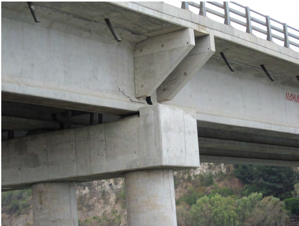
Figure 15.71 Shearing of bridge girder, North abutment of bridge, Puente Mataquito, 35.050712°S, 72.162258°W , April 16, 2010.
