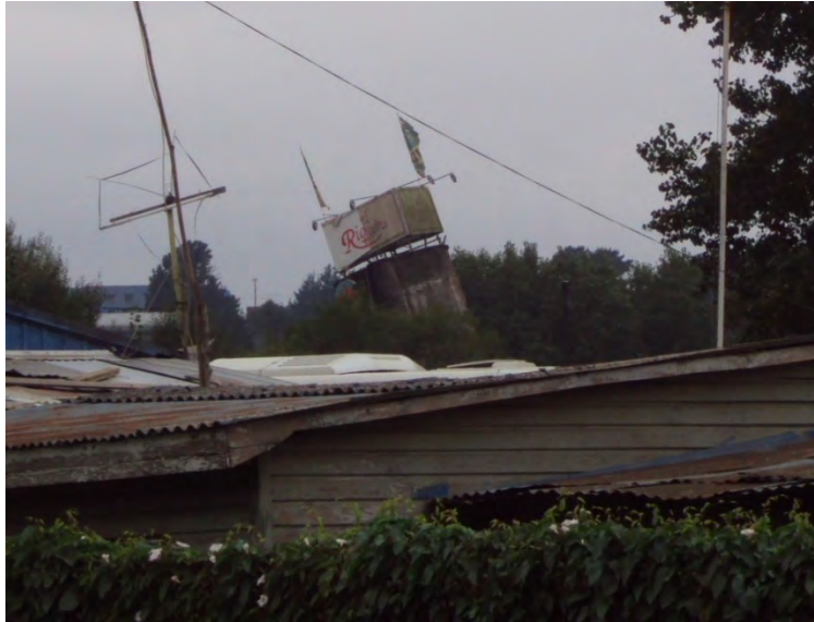
Figure 6.18. Leaning tank due to liquefaction of the foundation soil, near Arauco (S37.2458°, W73.3197°).
