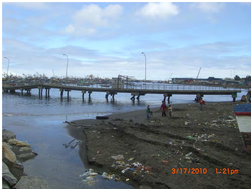
Figure 8.12. Damage to pile supported pier at small fishermen's Port of Coronel due to lateral spreading (S37.024319°, W73.156210°; 1321 hrs, 03/17/2010).
