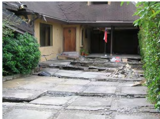
Figure 7.32. View of toe of translation slide in foreground of left photo (also note that the driveway behind the toe is not damaged(S 36.79134°, W 73.05762°; 1150 hrs on 03/17/10), and view of the head scarp of the translation slide at back of driveway in the right photo (S36.79126°, W73.05719°; 1130 hrs on 03/17/10).
