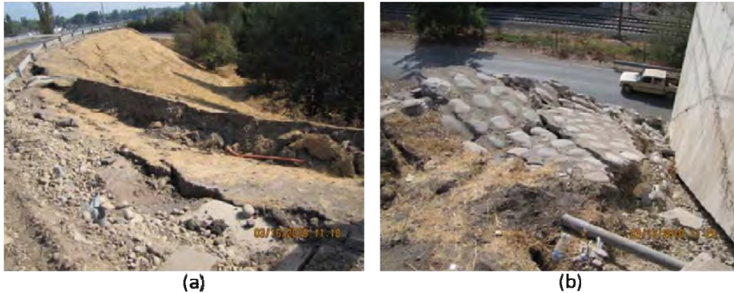
Figure 9.59. Highway 5 crossing near Paine; (a)View of bridge approach from East (S33.854592° W70.747687°; 1118 hrs on 3/16/2010); (b) View of damaged bridge abutment (S33.854211° W70.747784°; 1120 hrs on 3/16/2010)
