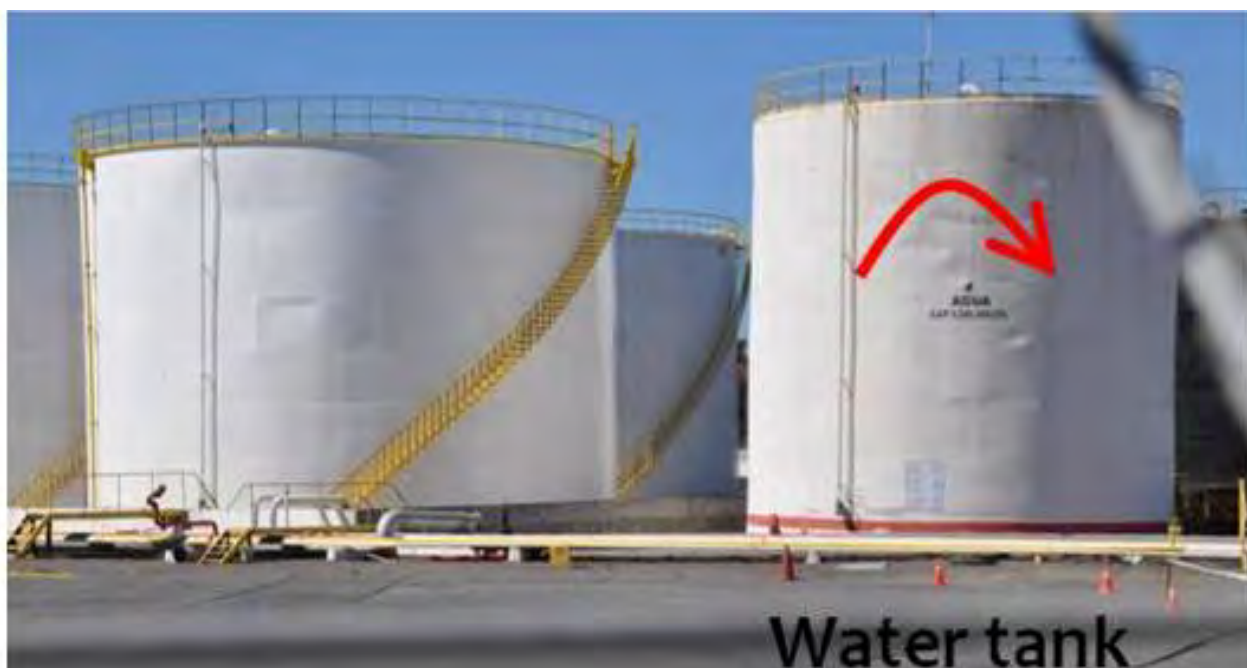
Figure 8.30. Tilted water tank at Petrobras gas facility (S36.7270°, W73.1272°; 1250 hrs, 03/15/2010).
