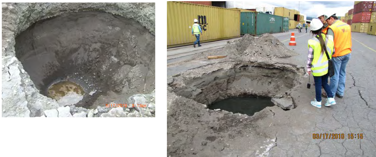
Figure 8.5. Development of sinkholes (2.2 m deep, 3.5 m diameter) as a result of crack (gap) in pipe (S37.0339°, W73.1467°; 1513 hrs, 03/17/2010).
