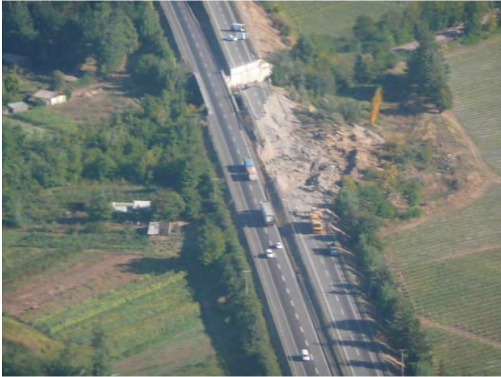
Figure 6.16. Typical road base failure along Pan American highway. Line of trees show where the water crossing intersects the highway. These type of road failures were observed at regular intervals corresponding to the minor water crossings. This picture is from near the town of Curico ( \sim S34.7794^\circ , \sim W71.1599^\circ , 17:30, 3/6/2010).
