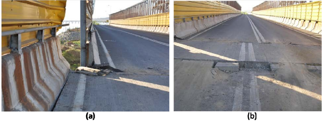
Figure 9.21. La Mochita bridge (a) Transverse gap developed between deck and south abutment. View looking north. (-36.847798°, -73.054797°; 1856 hrs on 3/15/2010), (b) Damage at the south abutment-road-deck interface due to transverse shift of the deck. View looking north. (S36.847761°, W73.054777°; 1856 hrs on 3/15/2010).
