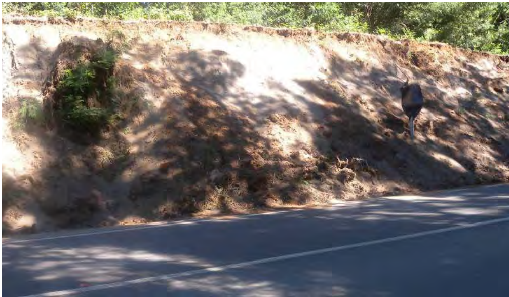
Figure 10.6. Sloughing of unconsolidated fluvial sand in a road cut North of Santa Juana (37.1111°S, 72.9876°W).
