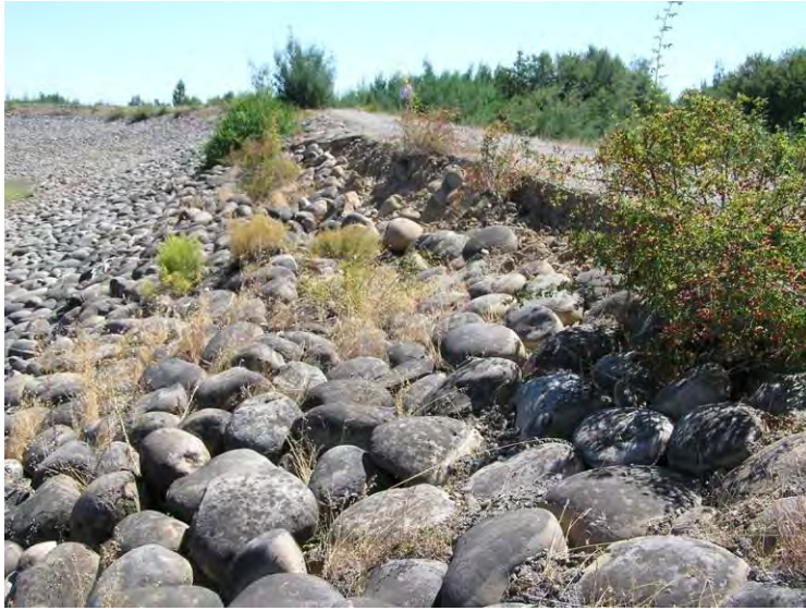
Figure 11.4. March 10, 2010. Small Area of Upstream Crest Slumping on Coihueuco Dam (S36.636902°, W71.788897°)
