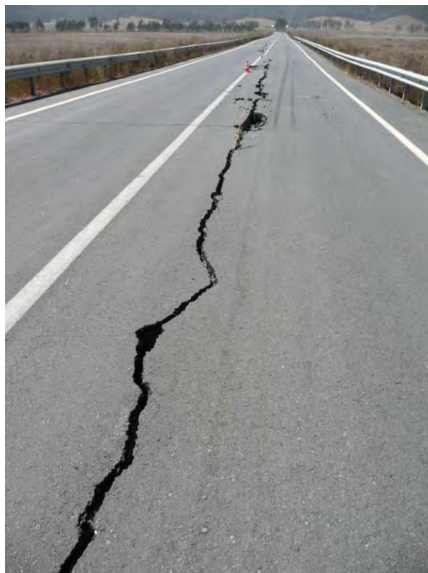
Figure 6.12. Impact of liquefaction and lateral spreading on the north approach fill of Mataquito Bridge (S3505078°, W72.16240°, 11:00, 3/8./2010).
