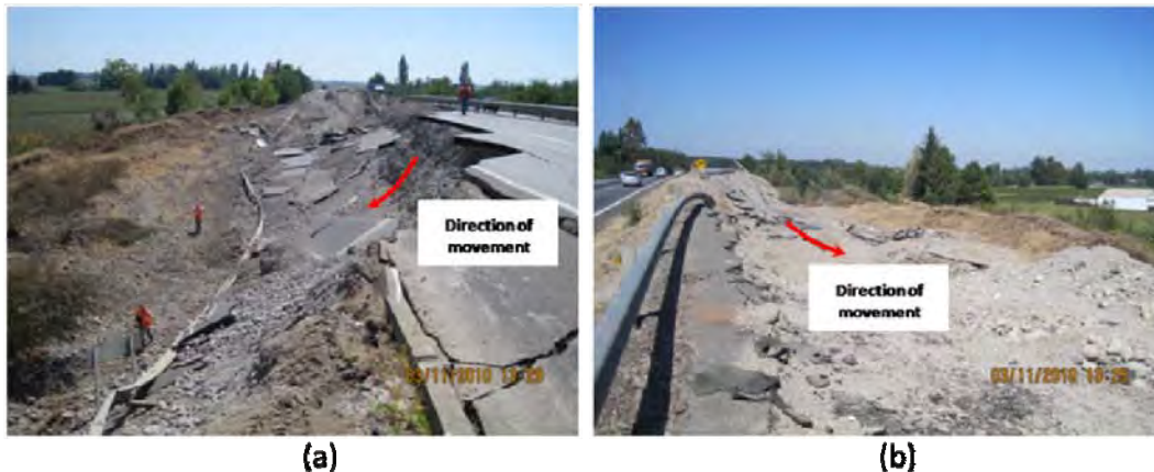
Figure 9.57. This embankment fill collapsed together with an overhead near Copihue, north of Parral, closing the South bound of Route 5 (a) View from the South, (b) View from the North (S36.087891, W71.791513, 1325 hrs on 3/11/2010)
