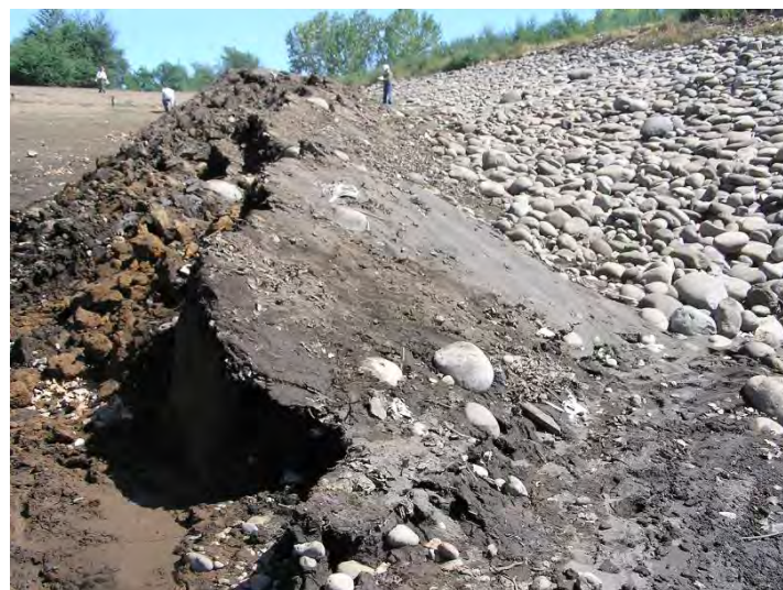
Figure 11.1c View of toe bulge area near left abutment of main dam, showing fine sand at the ground surface; due to the foot traffic it was not possible to see evidence that would allow one to classify these features as sand ejecta from soil liquefaction.
