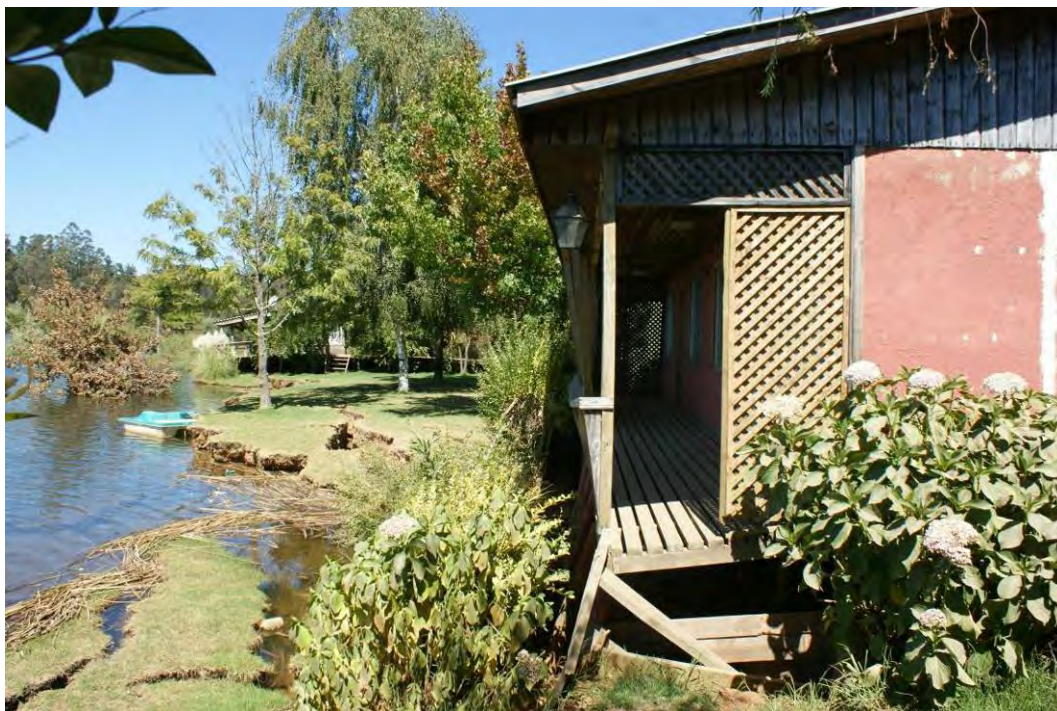
Figure 14.13. Lago Vichuquen. Lateral spreading has affected much of the ground underlying a small lakeside cabana hotel. Some shore side piers of the cabanas were submerged and there was evidence of structural damage as well. (S34.796345°, W72.07885°; 12:58 hours on 3/15/2010)
