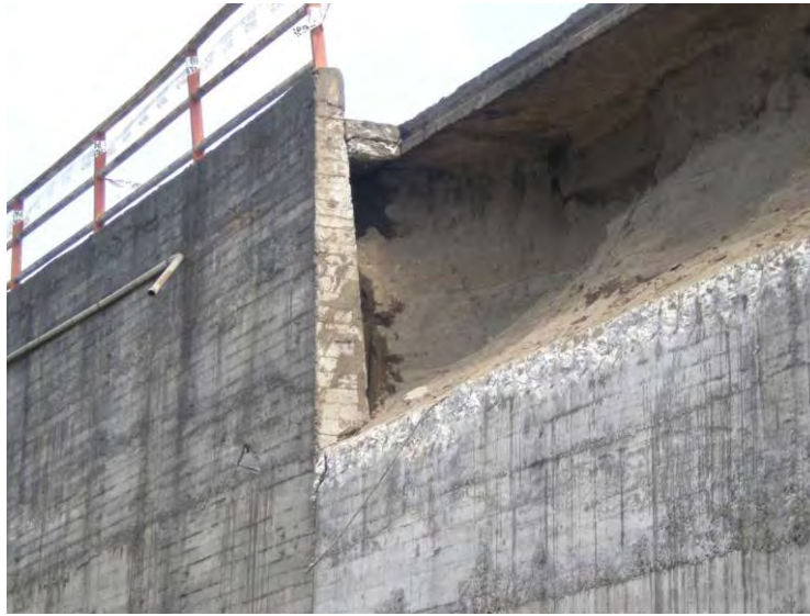
Figure 12.9. Granular fill soils and water seepage evident behind failed portion of wall.
