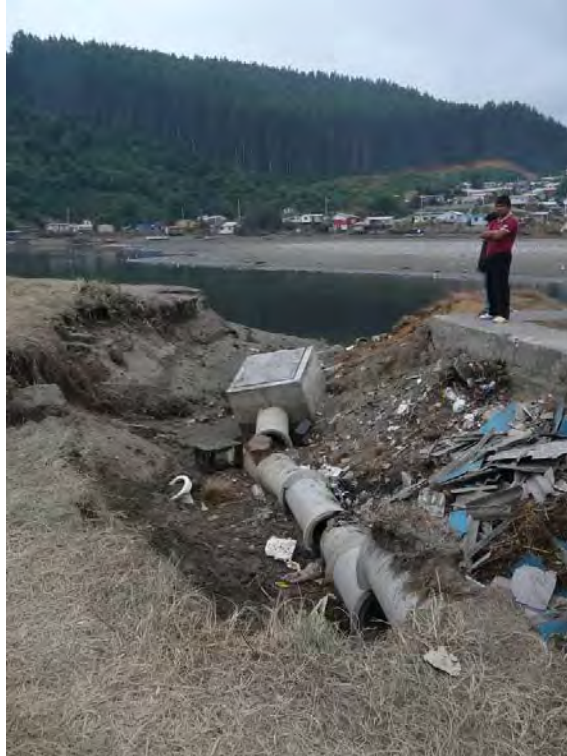
Figure 13.1. Tsunami scoured out the foundation of this storm sewer outfall at Laraquete (S37.165352° W73.188051, 1907 hrs on 03/16/2010).
