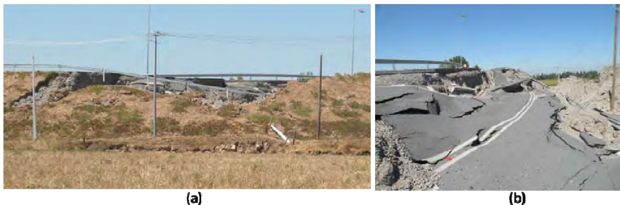
Figure 9.58. Curved overpass embankment failure 13 km North of Parral (a) Translational 3-D slide failure, (S36.0343 W71.7568; 1405 hrs on 3/11/2010) and (b) Failed outside of the curved embankment (S36.0347 W71.7558; 1409 hrs on 3/11/2010)
