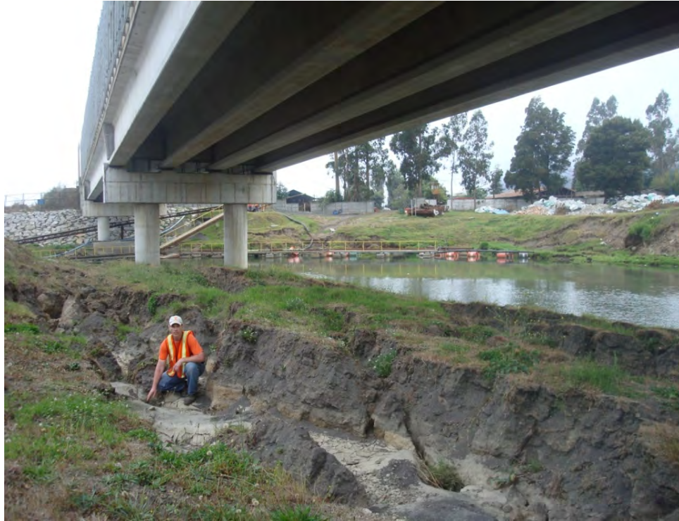
Figure 15.27. Liquefaction-induced lateral spread at Concepcion bridge parallel to the Bio Bio River. (36.84722°S, 73.05530°W; 27 March 2010; 09:25)
