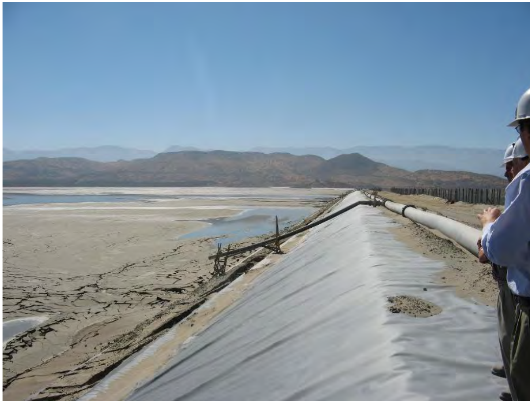
Figure 11.10. March 9, 2010 View along the Upstream Face of the Ovejeria Tailings Dam. There is no damage to the liner and no signs of slumping of the sand beneath the liner (S33.052911°, W70.807067°)
