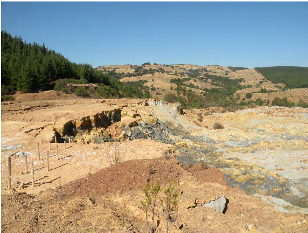
Figure 11.24. Upper Scarp of Failed Tailings Impoundment Looking Northeast ( 35.184679^{\circ} S, 71.759410^{\circ} W)
