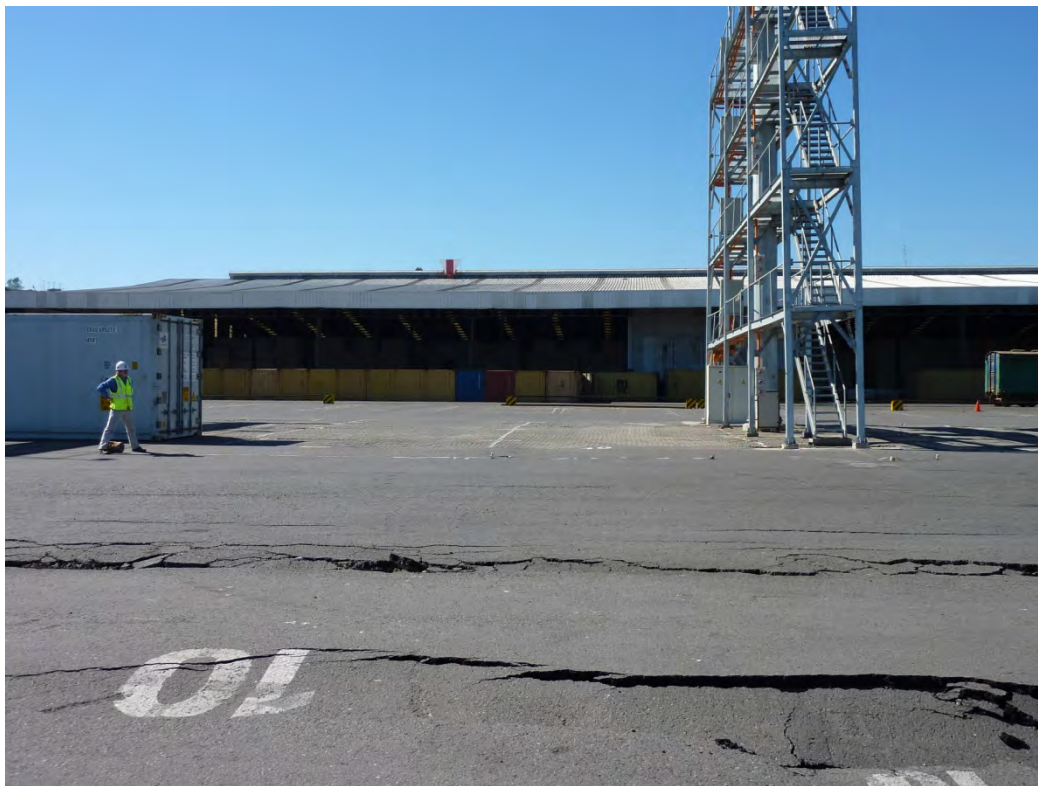
Figure 15.75 SASW line 2, and lateral spreading looking north, Port Coronel, April 14, 2010 (37.028874°S, 73.149768°W).
