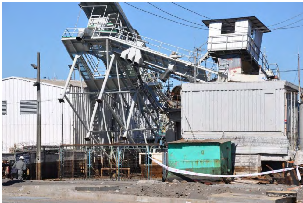
Figure 8.27. Damage to structures neighboring the fish packaging facility (S36.7267°, W73.1282°; 1200 hrs, 03/15/2010). Note the scum level at the base of the structure of approximately 1-2 m evidence of the water rise.
