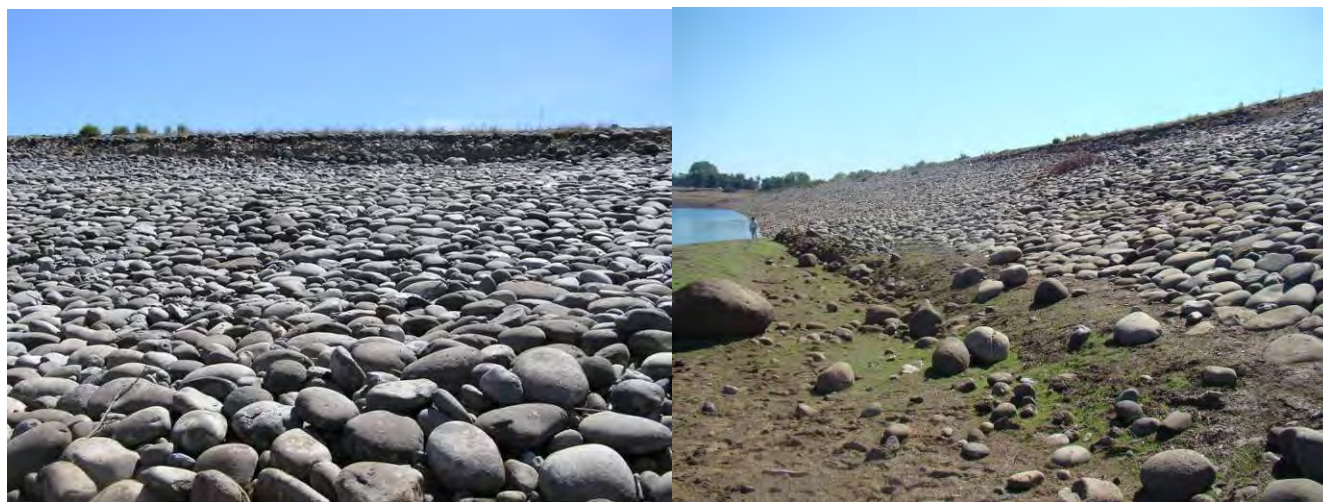
Figure 11.3. March 10, 2010. Slumping at Coihueco Dam Crest and Bulging at Dam Toe. (S36.636508°, W71.792505°)
