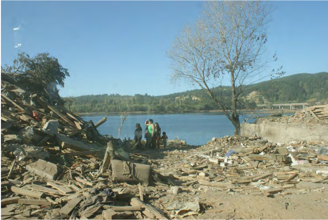
Figure 14.2. Constitución. Debris removal and road clearing still underway in the tsunami inundation zone along the Maule River. (S35.340323°, W72.396772°; 16:54 hours on 3/15/2010).
