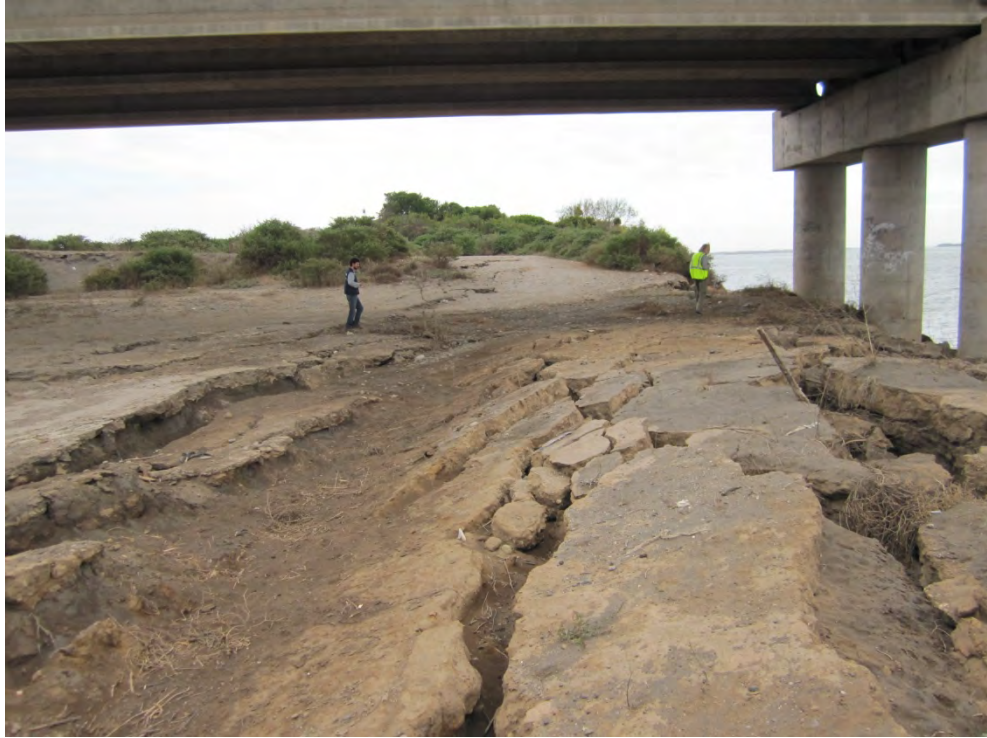
Figure 15.64 Lateral spreading on the south end of the bridge, Puente Mataquito, 35.050712°S,72.162258°W, April 16, 2010.
