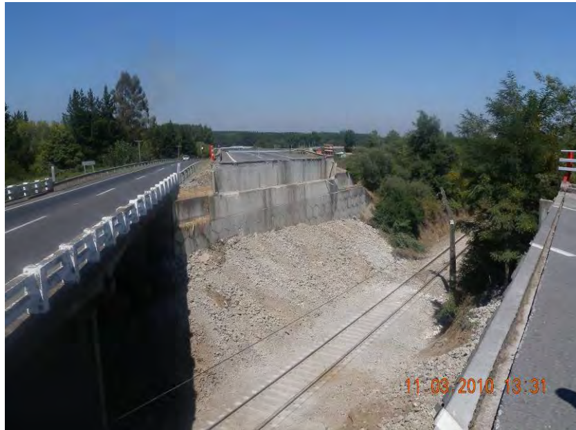
Figure 12.2. Reinforced Earth bridge abutments at a collapsed rail crossing on Route 5 north of Parral (36.0803°S, 71.788°W)
