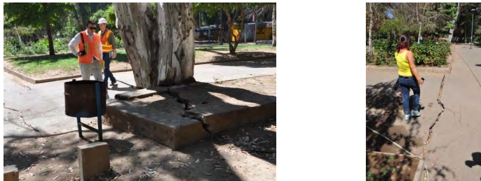
Figure 9.32. Ground failure in a park area near the shore of the Rio Claro in Talca (S35.419919°, W71.682289°; 1408 hrs on 3/18/2010), views looking north and south, for left and right images, respectively.
