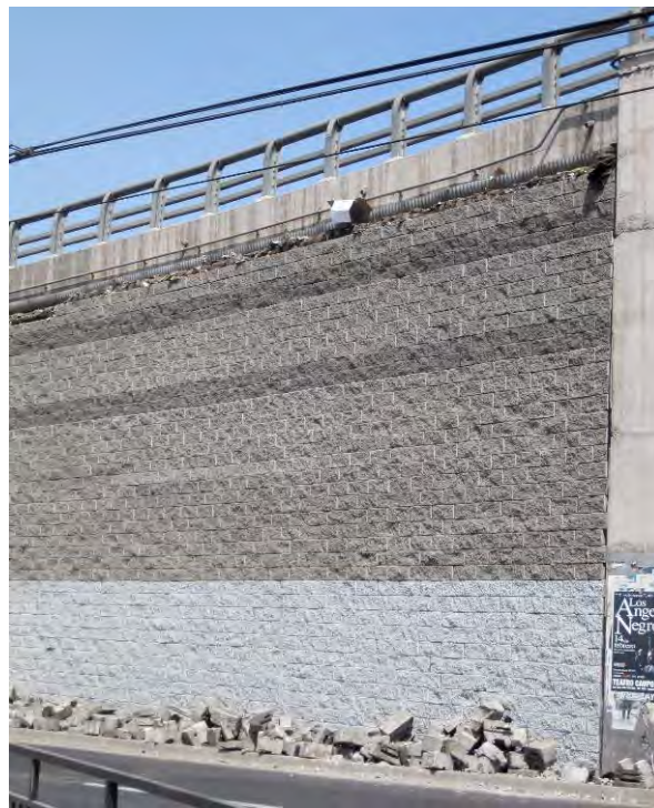
Figure 12.3. Block faced mechanically stabilized embankment, Intersection of Americo Vespucio Norte and Lo Echevers. (33°22'34.54"S, 70°44'52.83"W)
