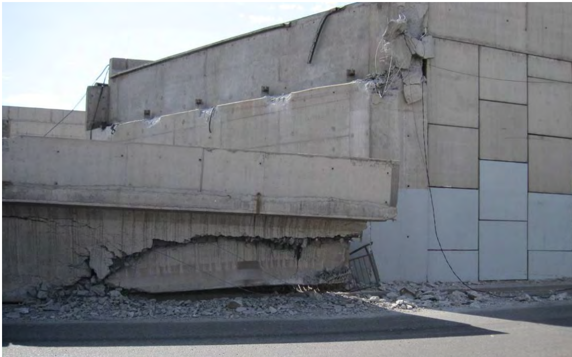
Figure 12.1. Intersection of Americo Vespucio Norte and Independencia. Abutment of a collapsed bridge. (33°21'57.83"S, 70°41'17.71"W)
