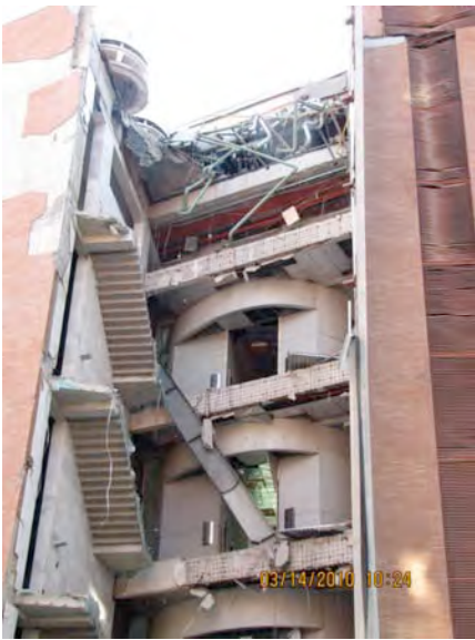
Figure 5.11. Site DA003 ( S33.387985^{\circ} W70.618815^{\circ} , 1015 hrs on 03/14/2010) 6-story commercial building. Damage of non-structural elements (glass windows, red brick façade) (Figures 11a,b) and emergency staircase (Figures 11c,d). Evidence of ground deformation (Figure 11e).
