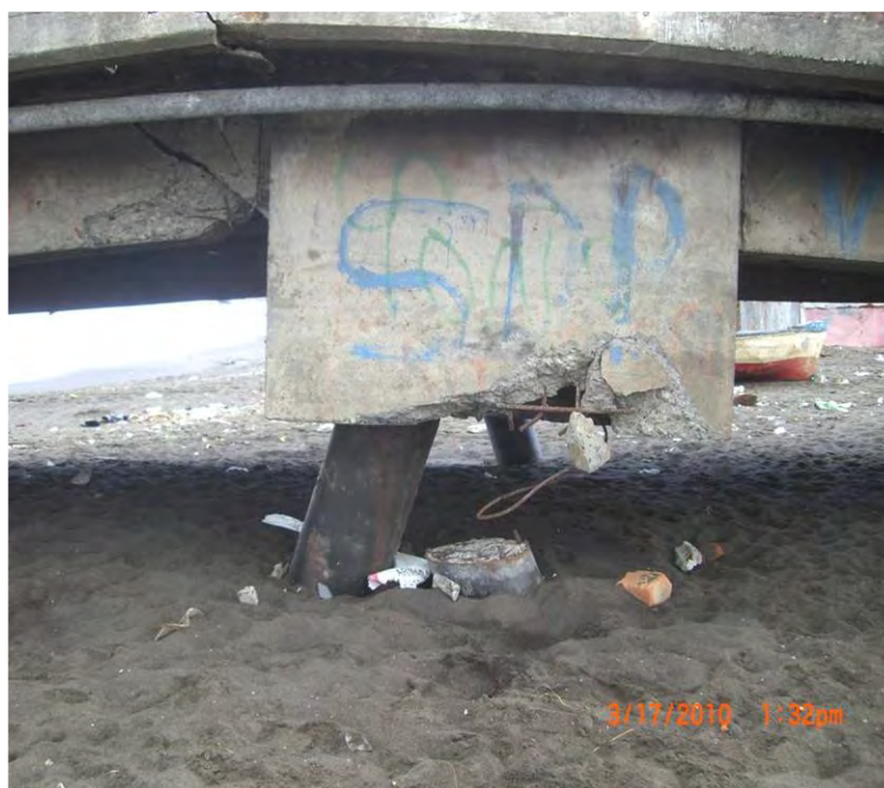
Figure 8.13. Photograph of pile cap with battered piles supporting pier at small fishermen's Port of Coronel showing pull out of trailing row piles (S37.024319°, W73.156210°; 1322 hrs, 03/17/2010).
