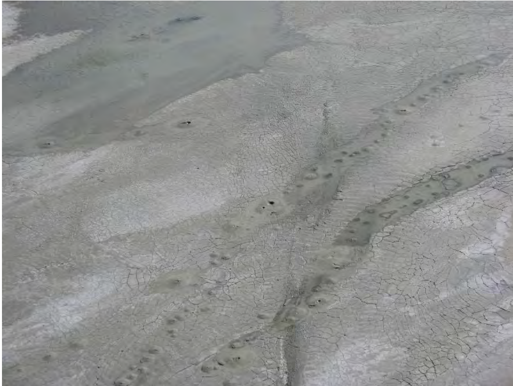
Figure 11.17. March 10, 2010 Sand Boils in Tailings Upstream of Caren Dam (S34.111476°, W71.141992°)
