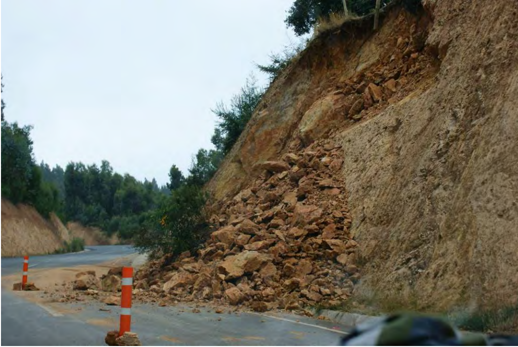
Figure 14.18. Lota Alto, Bio Bio region. Failures on the road cuts along one of two main highways leading to the Port of Coronel and surrounding coastal cities. (S37.047677°, W73.061597°; 15:30 hours on 3/16/2010)
