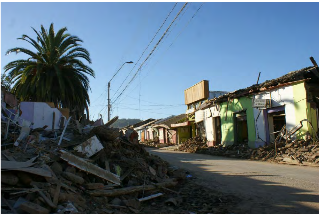
Figure 14.3. Constitución. Tsunami damage merges with shaking related damage in the older section of the city center with its many adobe and unreinforced masonry buildings. (S35.335383°, W72.410055°; 17:25 hours on 3/15/2010).
