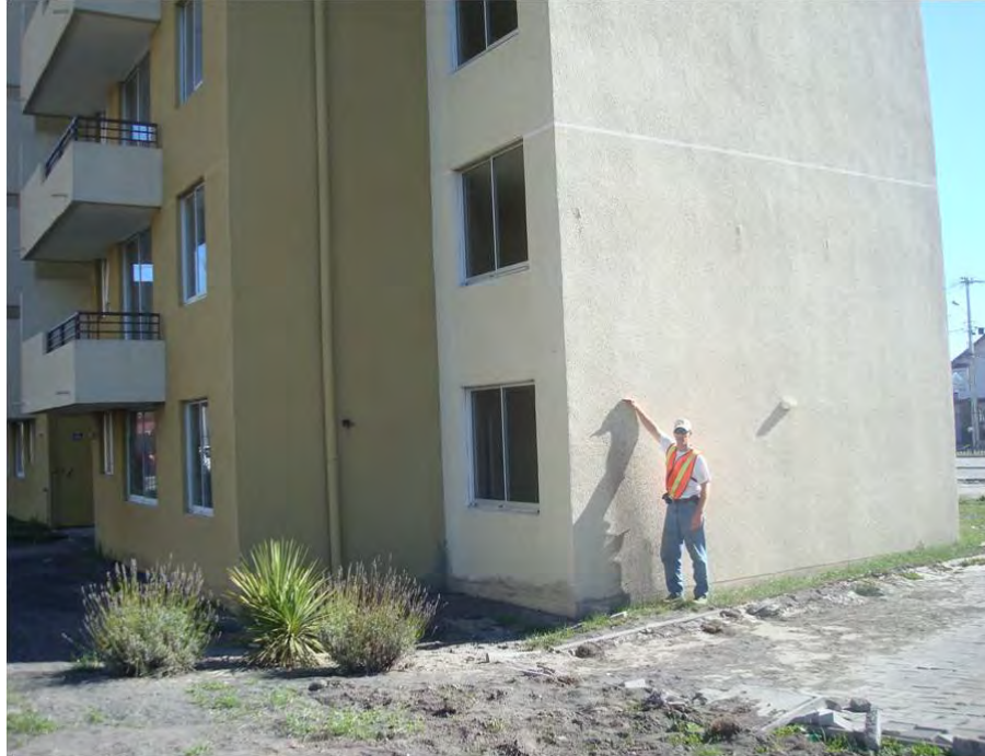
Figure 15.31. Height of ejecta sprayed onto wall of Riesco southwestern 8-story apartment building in Concepcion. Gray soil in foreground of photo also is sandy silt to silty sand ejecta, (36.79076°S, 73.08155°W; 25 March 2010; 16:50)
