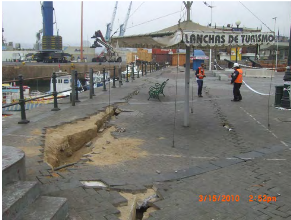
Figure 8.16. Photograph of lateral movement and vertical displacement of ground behind public dock at port of Valparaíso (S33.0375°, W71.6274°; 1452 hrs, 03/15/2010).
