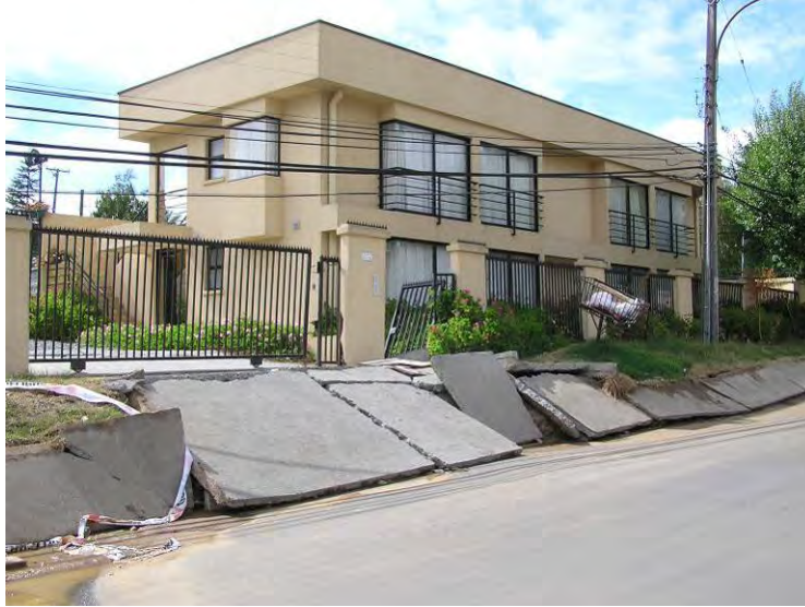
Figure 7.33. Apartment building underwent translation and tilt, but suffered no significant structural damage. (S 36.79167°, W 73.05721°; 1200 hrs on 03/17/10).
