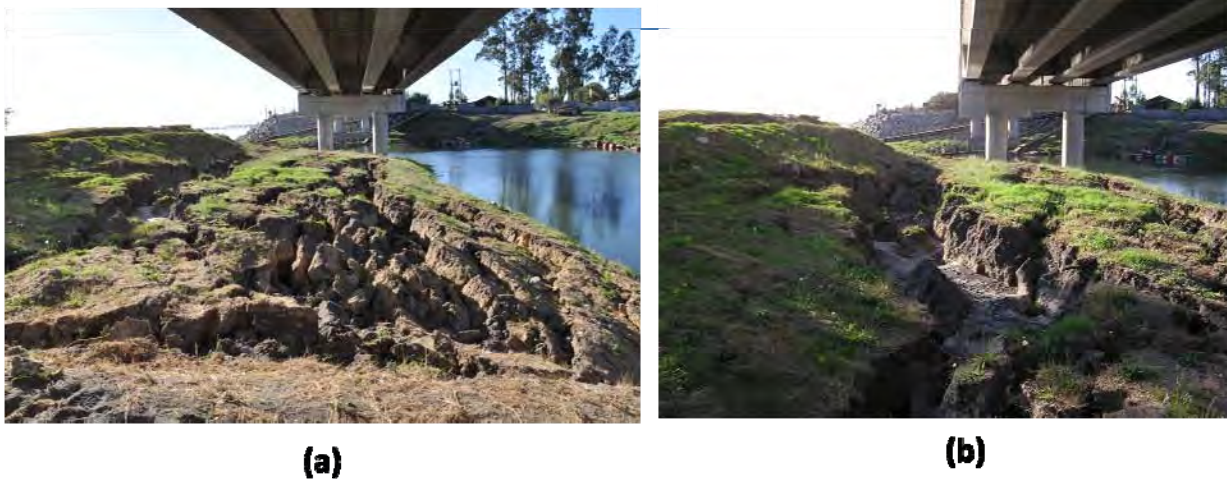
Figure 9.17. Ground failure at the La Mochita bridge, (a) looking north at bent #3 (S36.847389°, W73.055219°; 1831 hrs on 3/15/2010) and (b) looking north at bent #2 (S36.847495°, W73.055027°; 1835 hrs on 3/15/2010)
