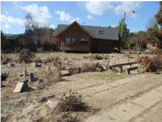
Photo 25 House that floated when tsunami came
