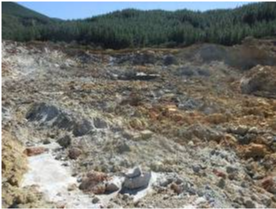
Photo 7 Tailing deposit after liquefaction
