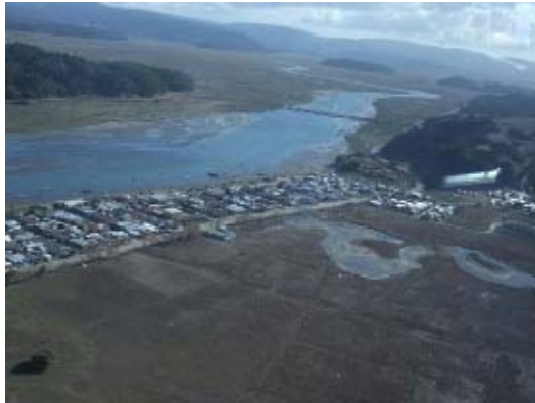
Photo 14 Peaty ground in and around Tubul
