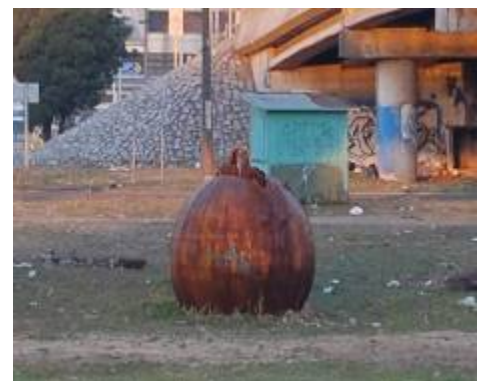
(Densification by dynamic compaction)
