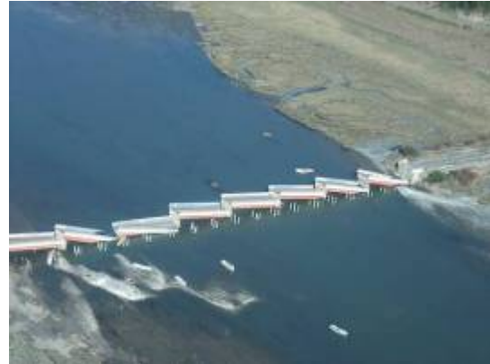
Photo 15 Collapsed bridge in Tubul
