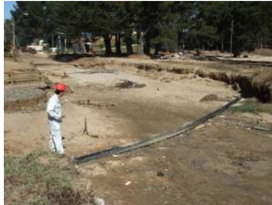
Photo 24 Exposure of buried lifeline after tsunami erosion
