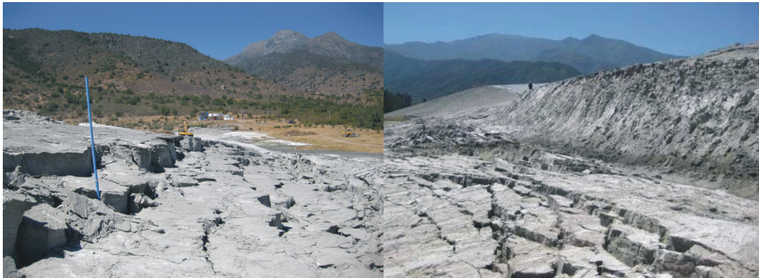
Fig. 11. Final situation after liquefaction of sand tailings dam, resulting from the earthquake of 27 February 2010, Maule Region, Chile.
