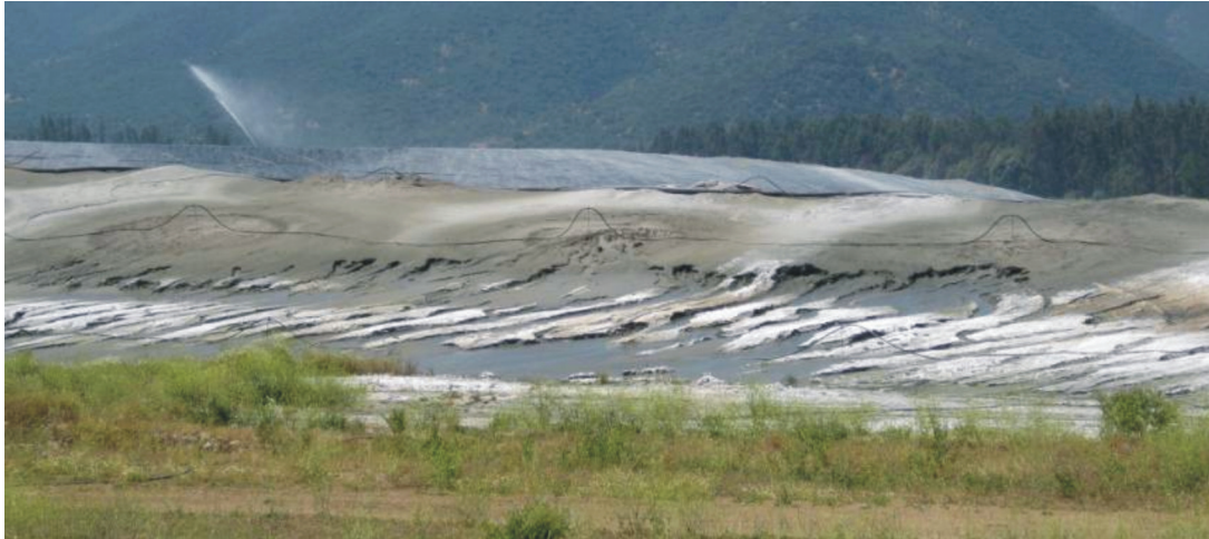
Fig. 11. Final situation after liquefaction of sand tailings dam, resulting from the earthquake of 27 February 2010, Maule Region, Chile.
