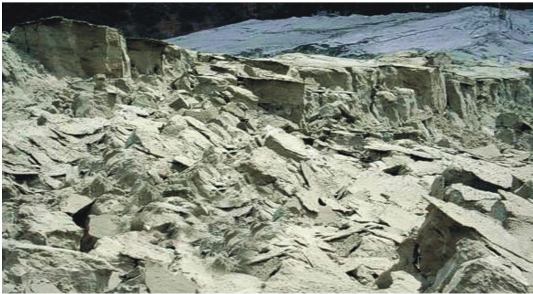
Fig. 6. Overtopping incident: (a) retaining dyke and basin of the sand tailings dam; (b) flow failure in downstream direction.
