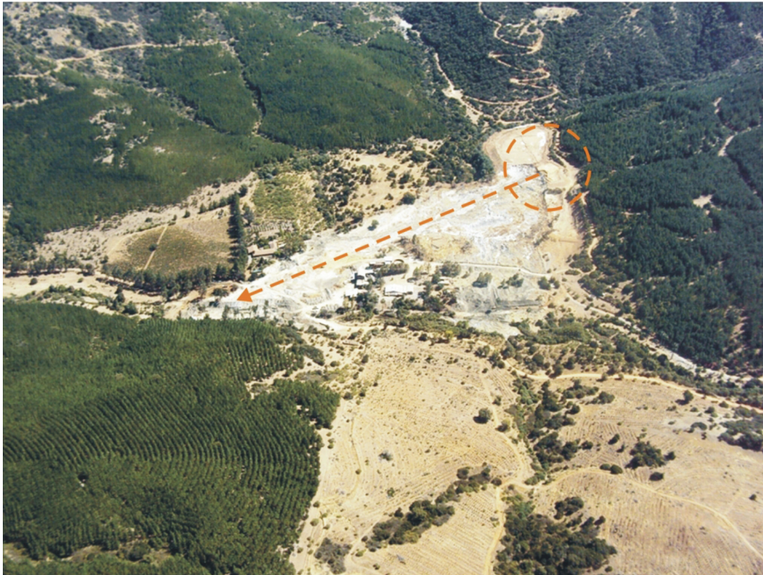
Fig. 8. Las Palmas sand tailings dam after the collapse generated by the 27 February 2010 earthquake.
