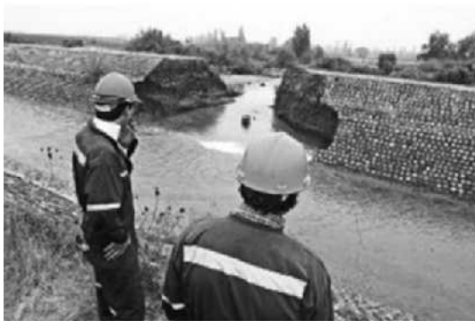
Figure 21. Earthen levee breach west of Colbún (S35.698672°, W71.487294°; photograph taken by Mr. Juan Carlos Romo of El Mercurio on 12 March 2010; http://diario.elmercurio.cl ).
