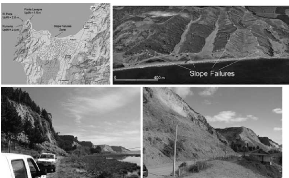
Figure 22. Massive slope failure occurred in Arauco area.
