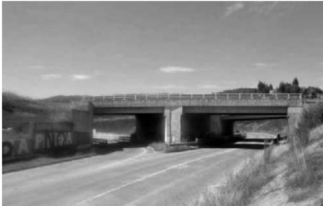
Figure 26. Multiple retaining structures for highway overpass structures south of Coronel.
