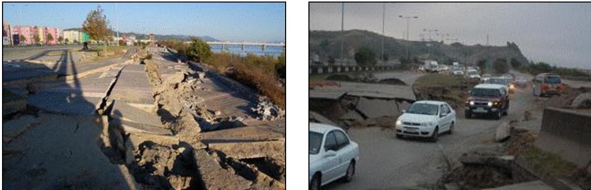
Fig. 13.- Cracks and settlements on right side of BioBio River caused by lateral spreading
