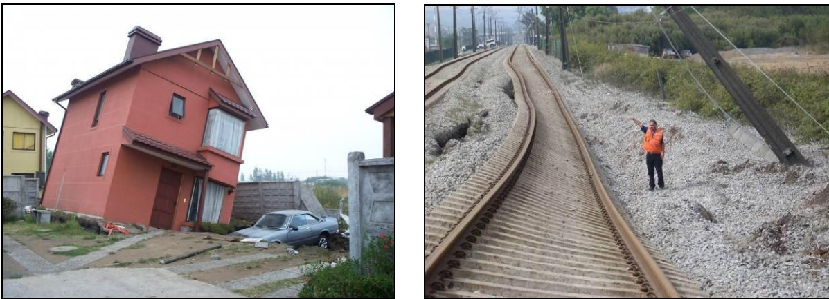
Fig. 11.- Liquefaction of flat areas. Condominium Brisas del Sol and railway near Concepción (EFE)
