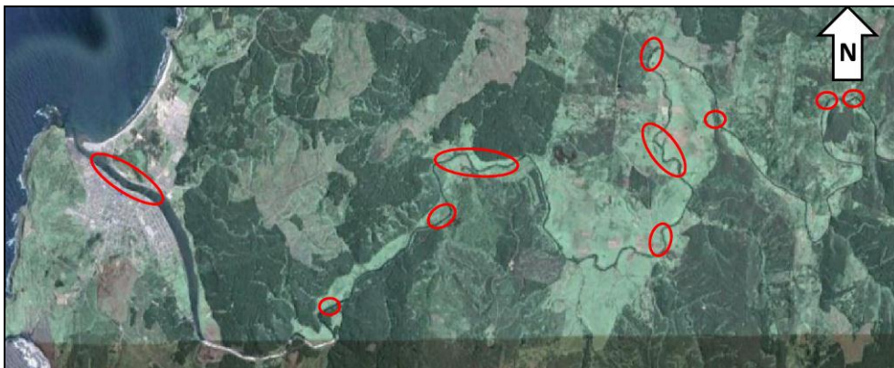
Fig. 12.- Lateral spreading observed along the Lebu River. Maule 2010 Chile Earthquake
