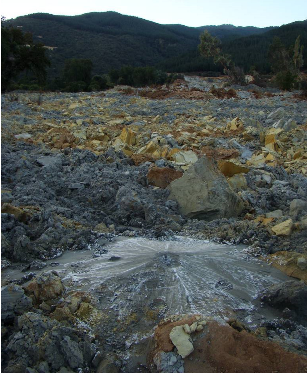
Figure 3.4 Sand-boil tailings along flow path (S35.18872, W71.75777) looking up towards the scarp is shown in Figures 3.2 and 3.3 (from GEER [2010]).
