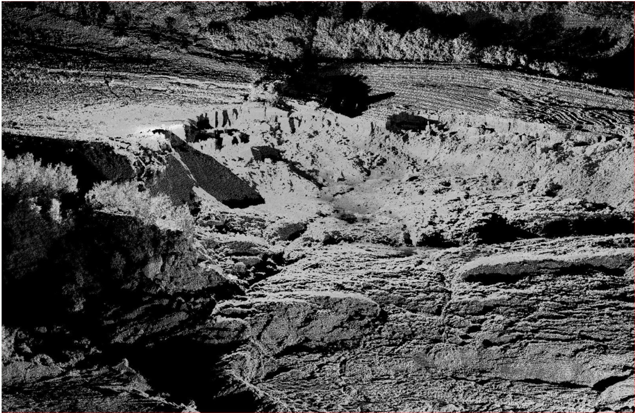
Figure 3.7 Detailed LIDAR of head scarp of Las Palmas tailings dam failure (from GEER [2010]).
