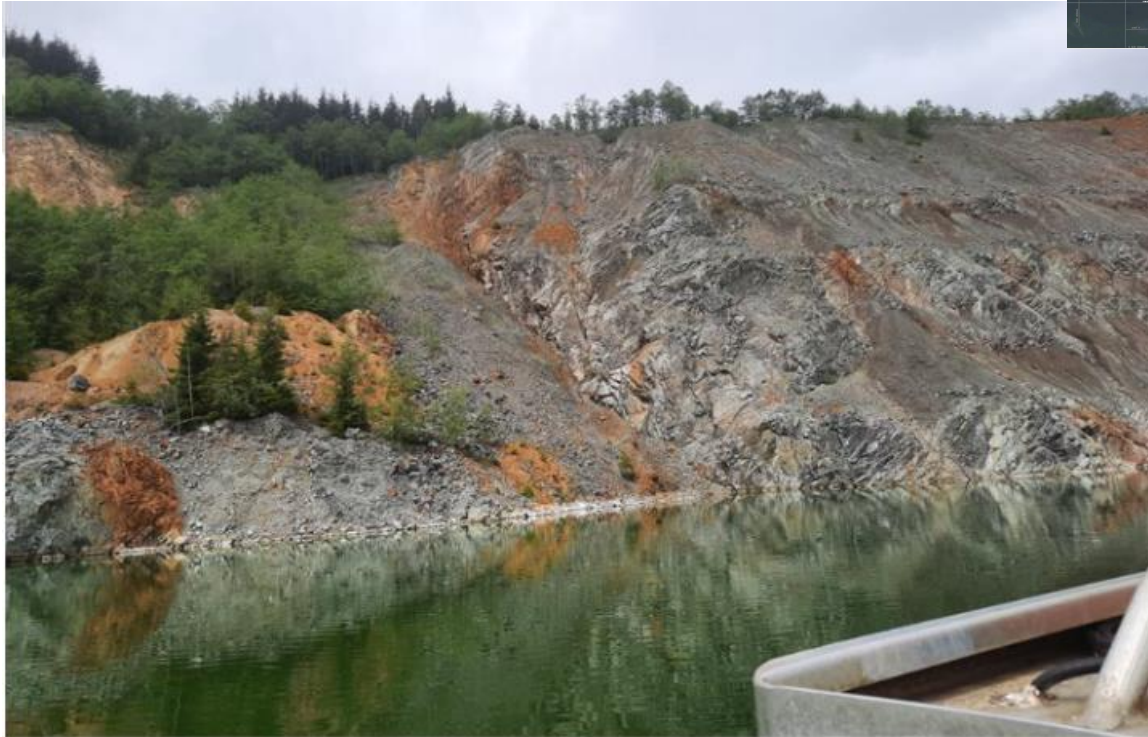
West slope movement (north end)
