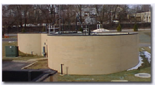
Conventional digesters (floating top)
