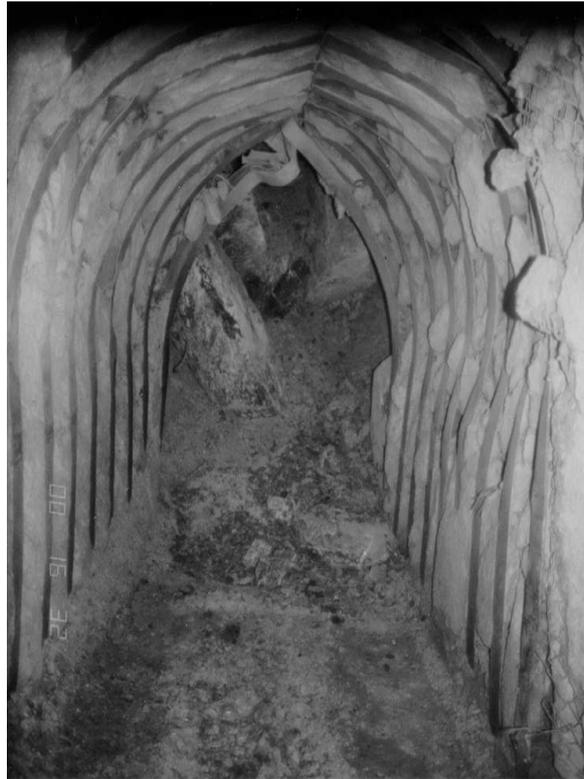
**Figure 6a : Buckling of arch legs.**
