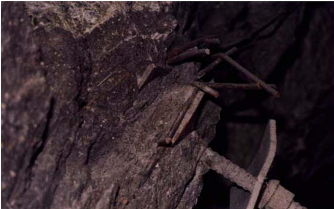
**Several layers of weld mesh reinforced shotcrete and a dwyidag bolt**
