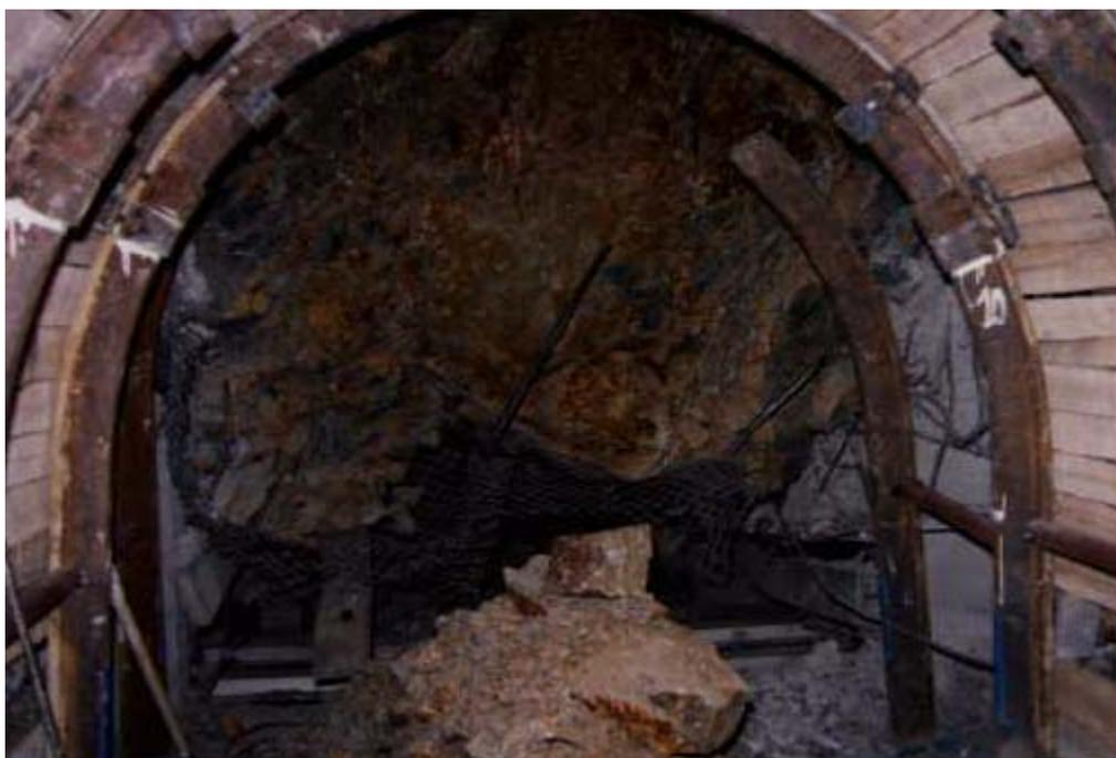
**A collapsed drift (squeezed) being rehabilitated with timber slats and arches**
