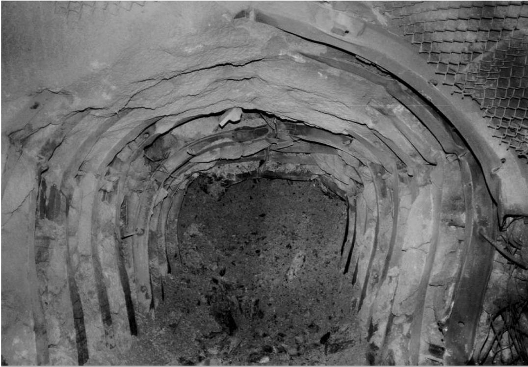
Figure 1 : If installed properly arches tolerated severe deformation without jeopardising the production.
