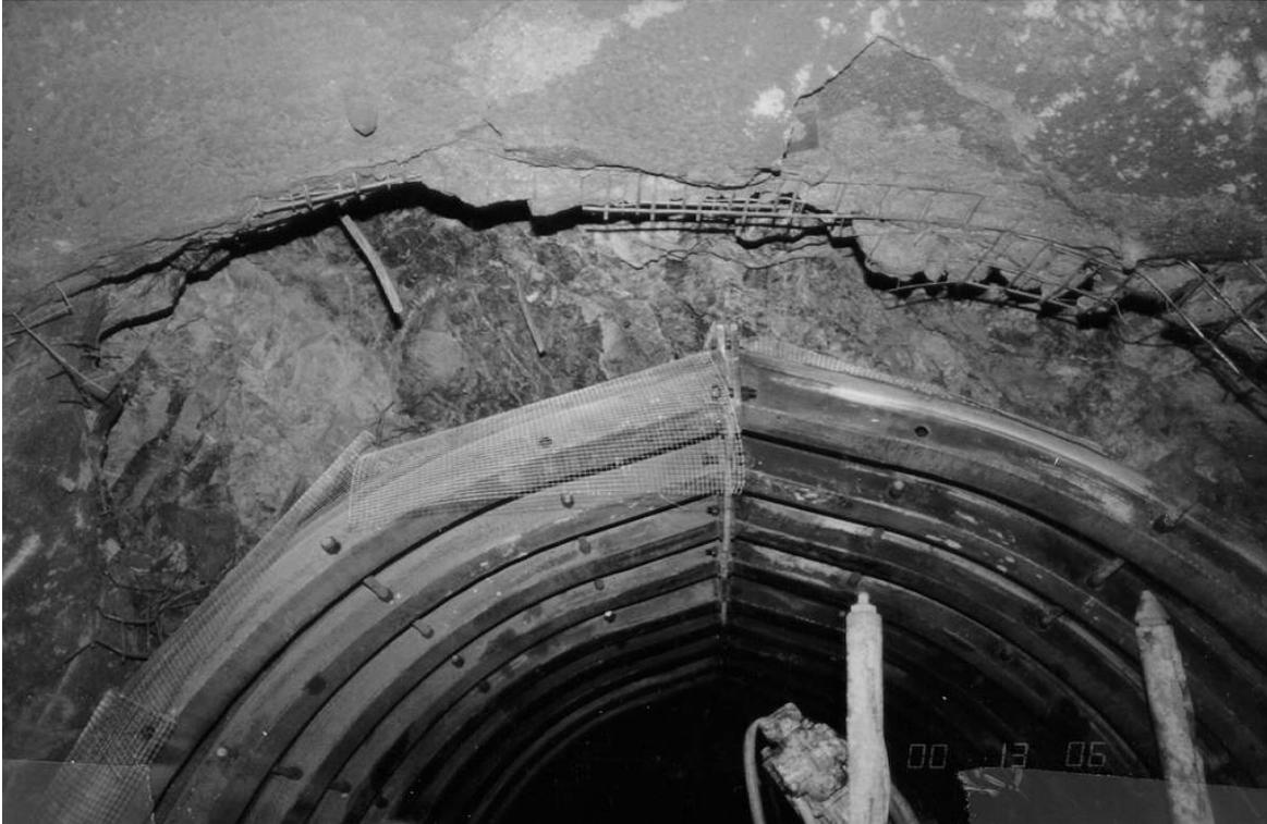
**Figure 10 : Initial reinforced shotcrete had to be slashed to increase the size of the tunnel in order to fit arches.**
