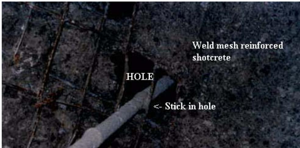
**Poor shotcreting of weld mesh**
