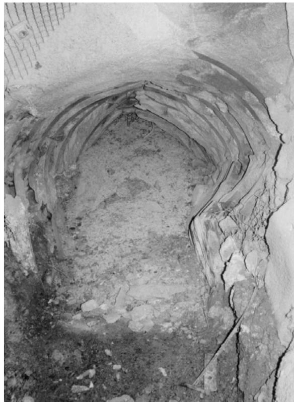
**Figure 6b : Buckling of arch legs.**
