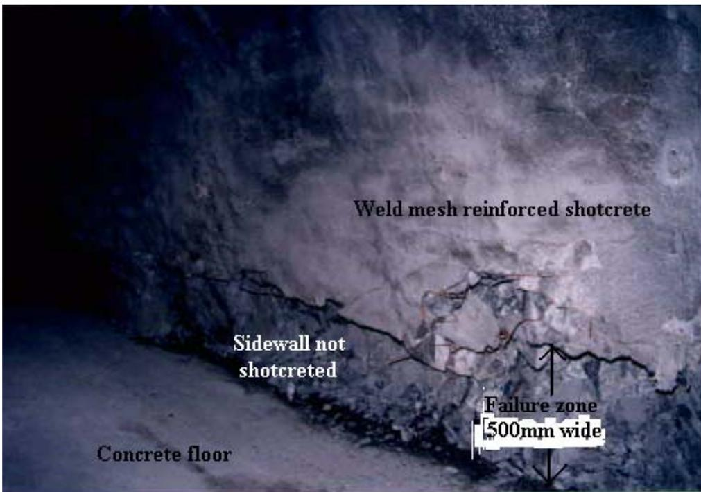
**Incomplete shotcreting results in failure 500mm into sidewall**
