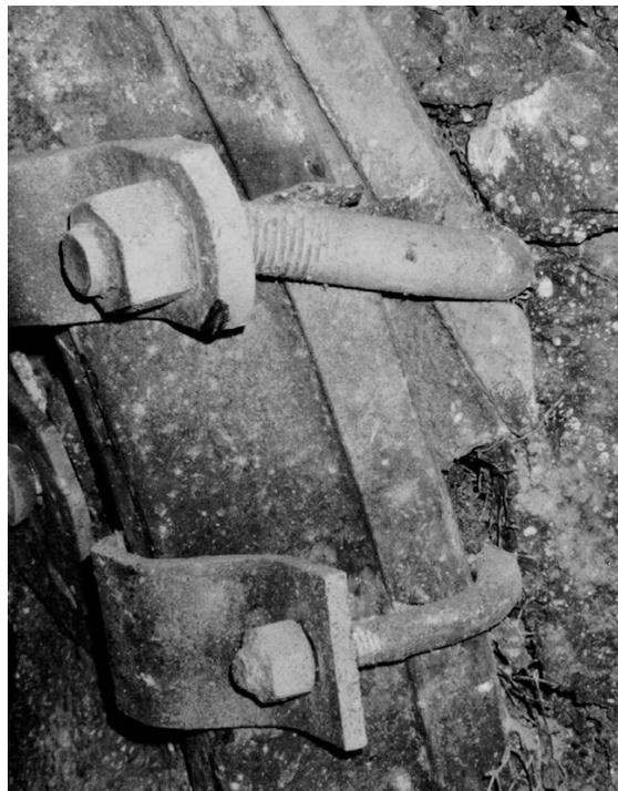
**Figure 10b : Failed ' U' clamp - yielding arch**
