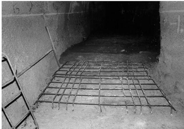
**Rebars in a grid and concreted in with 3m ropes into the floor**
