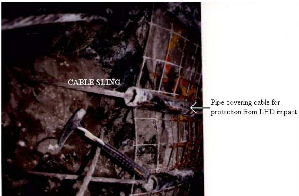
**Cable sling with pipe protection from LHD damage**
