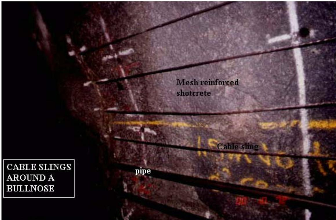
The length of the cable is kept as short as possible to limit elongation and thus provide more effective support. The cables are grouted into the rock mass for 3m. Not only does the cable provide excellent restraint to the rock surface, but it also contributes to the rock reinforcement.
