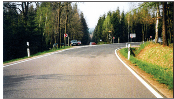
Figure HF-27 Example – Bad transition Intersection in horizontal curve
