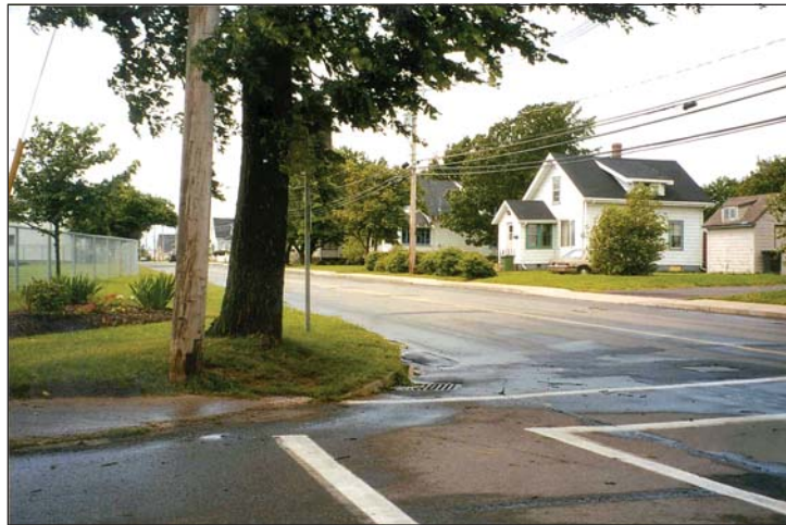
Visual obstruction in the corner of a conventional intersection.
