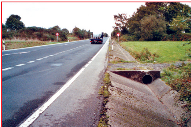
Hazardous drainage structure on a main rural highway (errant vehicle are directed on a vertical concrete structure)
