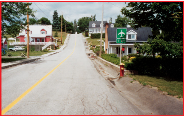
Hazardous drainage facility on a narrow and hilly road
