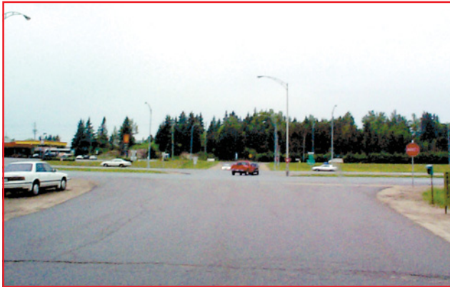
Excessive road width, leading to excessive speeds
