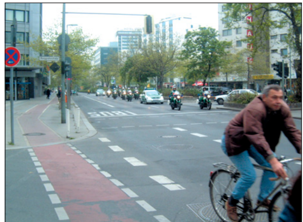
Urban arterials allowing proper separation of incompatible road users: wide and well-marked lanes, bicycle paths with different material and color and pedestrian traffic signals.
