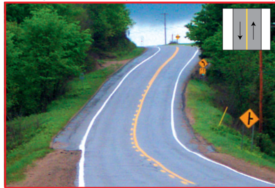
Due to the vertical curve, drivers may be surprised by the presence of the intersection and horizontal curve ahead
