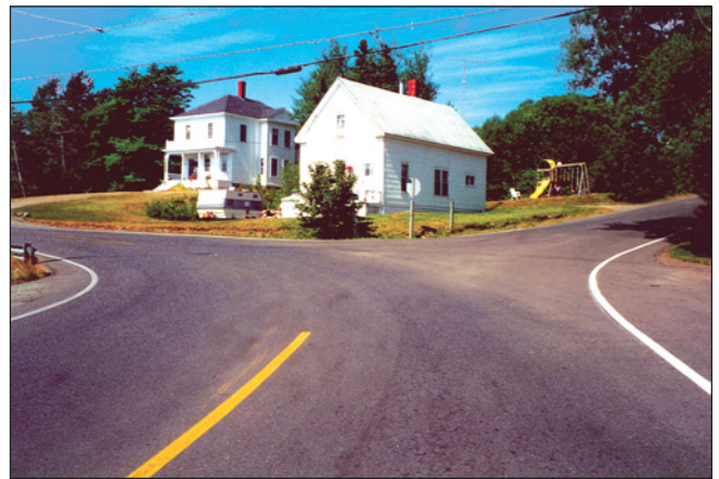
Y intersection that may cause hasardous manoeuvres (high speed turning manoeuvres, traffic conflicts).
