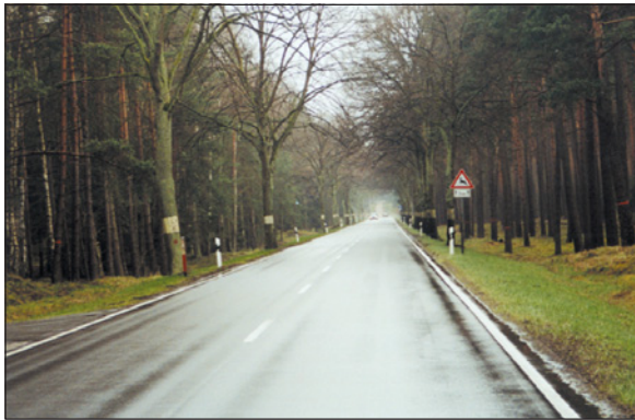
Figure HF-26 Example – Bad transition Intersection in horizontal curve
