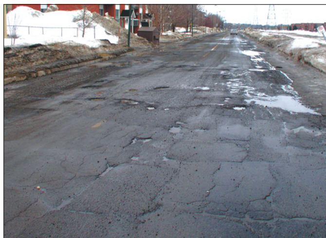
Severe deterioration of a road surface (combination of problems: cracking, potholes, depressions)
