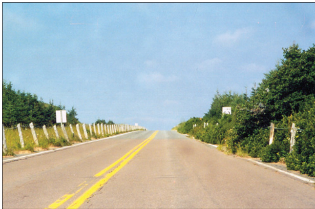
Inadequate maintenance (vegetation, guardrails)
