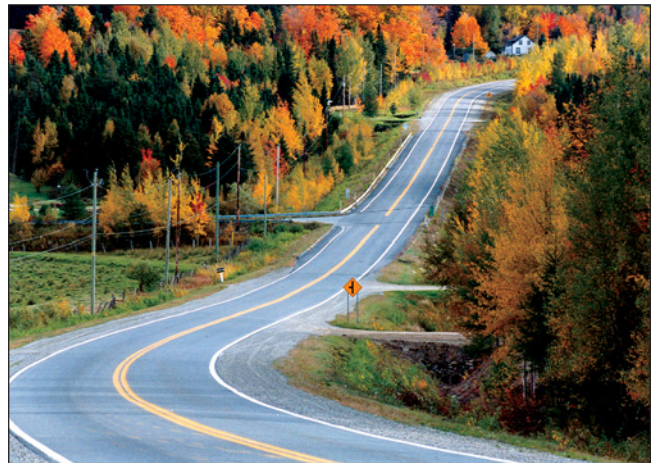
Hazardous combination: hill, intersection, accesses, horizontal curve.
