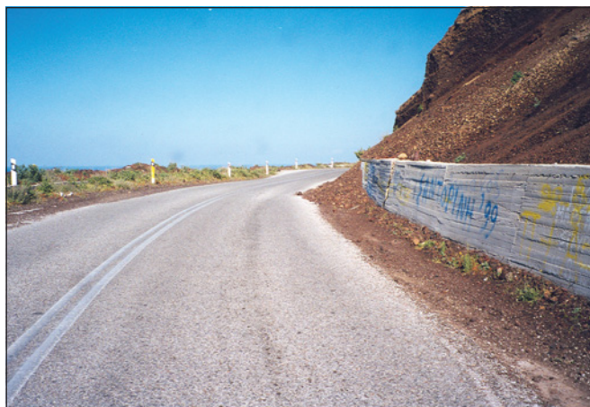
Debris on the road - The retaining wall is too short
