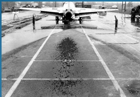
*Effect of jet blast on pavement*
