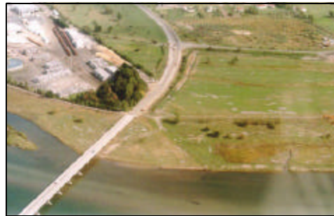
The Landing Road Bridge, after the 1987 New Zealand earthquake
