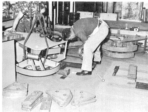
Fig. 3. Vibration Exciter Unit Being Installed in Laboratory
