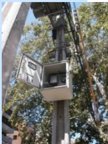
Ascom Head End installed in aerial transformer
