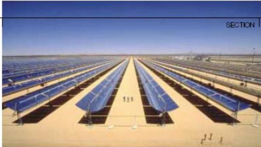
Figure 4 Parabolic trough concentrating solar collector field of the 150 MW (5 x 30 MW) steam cycle solar electricity generating systems at Kramer Junction, California (Source: KJC)
