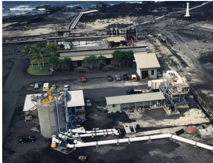
Figura 7.18. 210kW OC-OTEC Experimental Plant (1993-1998) in Hawaii (Source: Luis A. Vega, Ph.D. Project Director)
