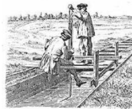
Figure 7. Technicians using a Pitot-Darcy tube (Darcy and Bazin, 1865).
