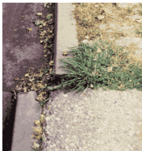
Left: Creeping along the Calaveras fault has bent the retaining wall and offset the sidewalk along 5th Street in Hollister, California (about 75 km south-southeast of San Jose). Right: Close-up of the offset of the curb. (Photographs by W. Jacquelyne Kious.)
