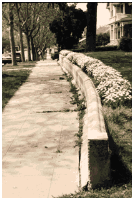
Left: Creeping along the Calaveras fault has bent the retaining wall and offset the sidewalk along 5th Street in Hollister, California (about 75 km south-southeast of San Jose). Right: Close-up of the offset of the curb. (Photographs by W. Jacquelyne Kious.)
