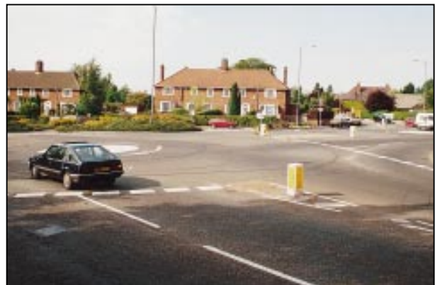
Photograph 39.3: Circulating carriageway made two-way and entry controlled by a mini-roundabout.
