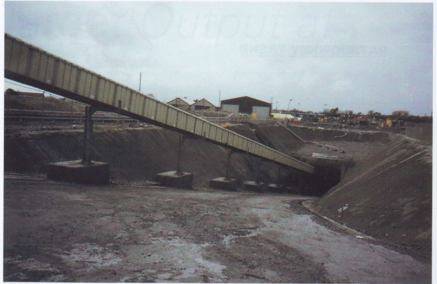
Lisheen mine decline and conveyor installation.
