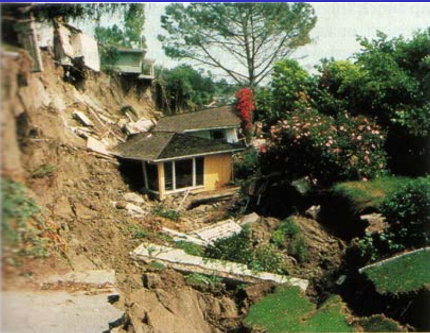
(A) This photograph shows the upper part of a landslide in California, where homes were displaced along the curved rupture surface of the slump block.
