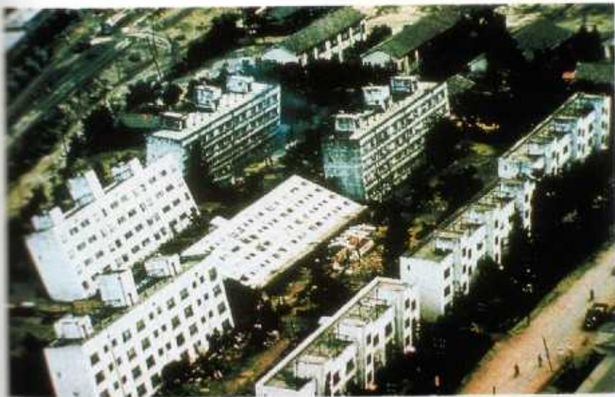
(A) Earthquake of June 16, 1964, Niigata, Japan. Apartment houses tilted by liquefaction. Poor foundations were partly responsible for this type of damage. About one-third of the city subsided as much as 2 m as a result of sand compaction. (Courtesy of USGS)
