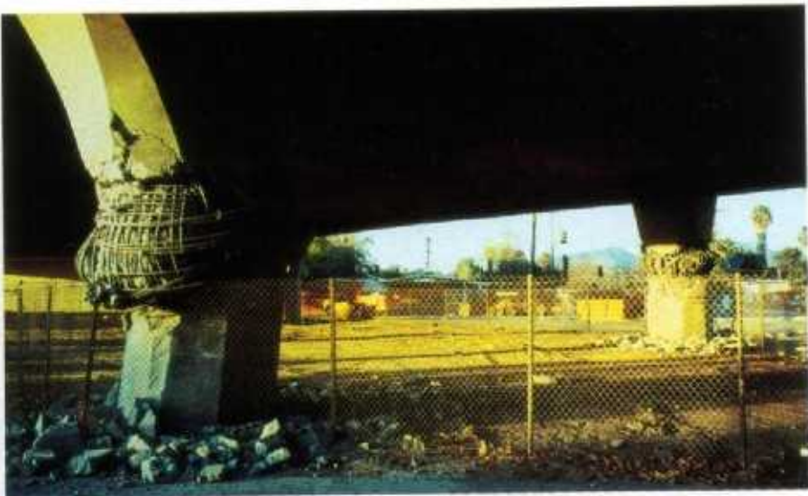
(B) Earthquake of January 1994, Northridge, California. Extensive damage to freeway overpasses occurred. (Photo by Geo-Tech Imagery)
