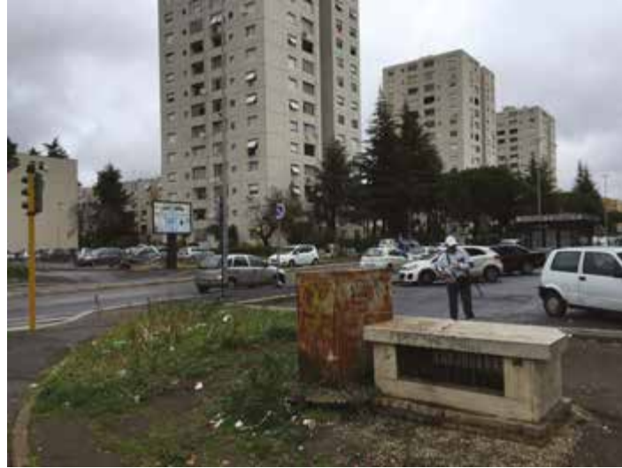
Figure 1. Typical example of one of the main roads of the district
