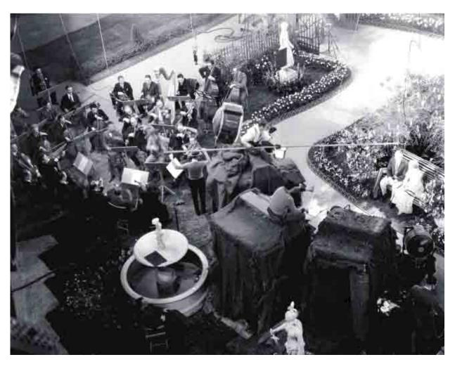
**82** This photograph, taken during the making of a Warner Bros. film, shows the coordination involved in early sound recording. Three large draped boxes house the cameras (bottom), a man holds a long boom over the actors' heads (far right) and a small orchestra plays.
