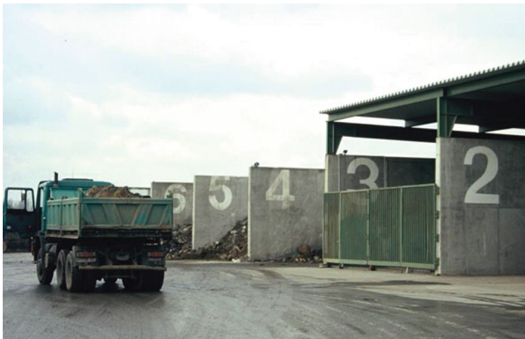
Fig. 6.1 Entrance area of a soil preparation plant exhibiting different boxes for soil storage before the preparation process begins and a sealed bottom to prevent leaching of contaminants
