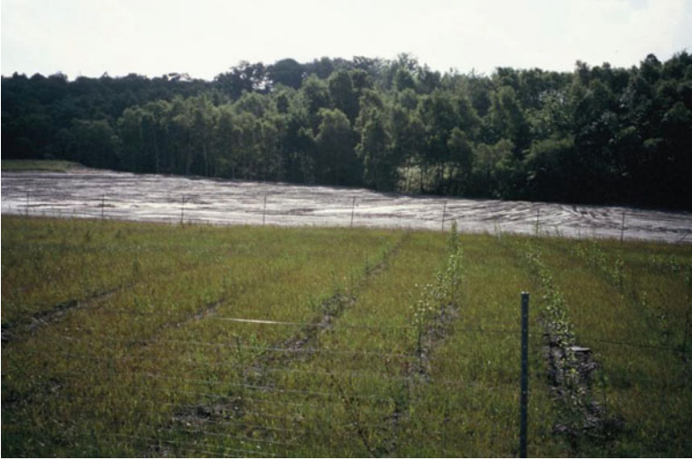
Fig. 3.15 Top of a mining waste heap showing narrow plantation of shrubs after the preparatory grass seed application in Osnabrück, Germany
