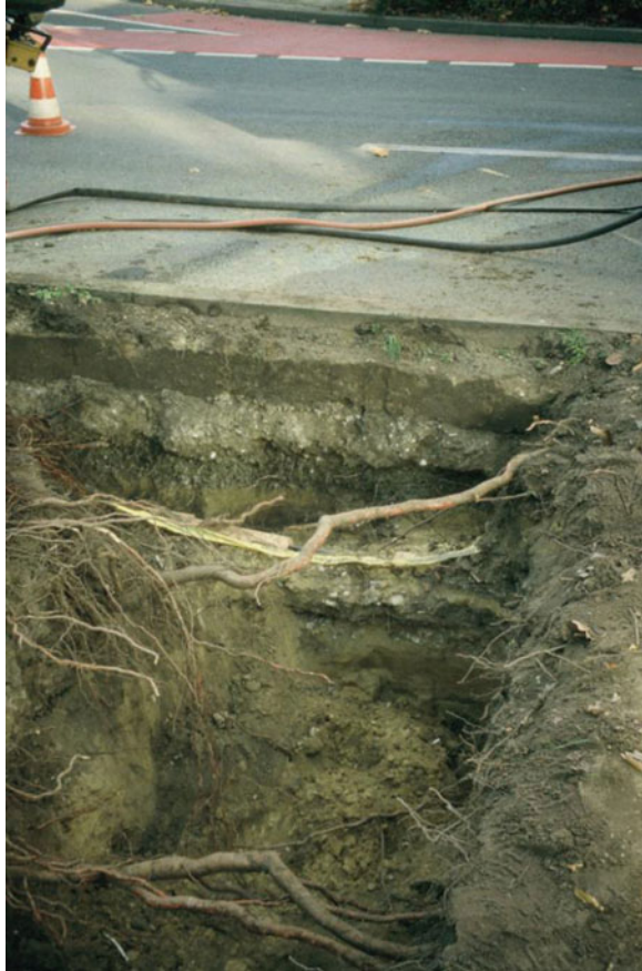
Fig. 4.9 Surviving tree roots after the vacuum excavator has removed the soil
