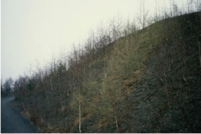
Fig. 3.13 Mining waste heap configuration with berms for erosion protection purposes in Osnabrück, Germany
