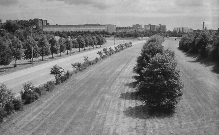
Fig. 2.3 De-sealed road in Munich, Germany
