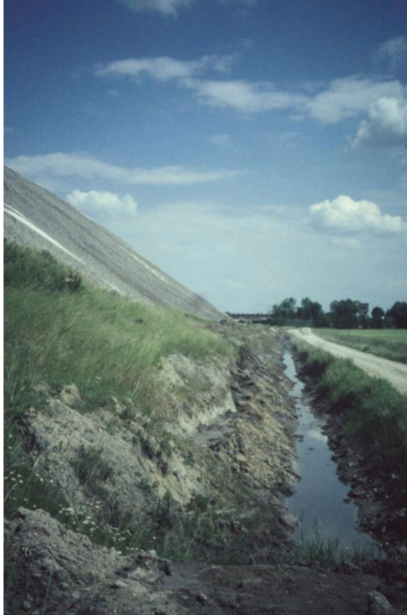
Fig. 3.18 Ditches to collect the salty runoff at the sides of the salt mining heap in the proximity of Hanover, Germany
