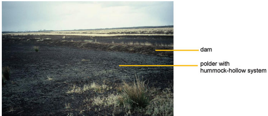
Fig. 3.40 Construction of polders interrupted by dams to prepare bog rehabilitation
