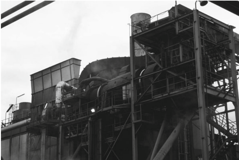
Fig. 6.25 Thermal treatment facility in Breda, The Netherlands
