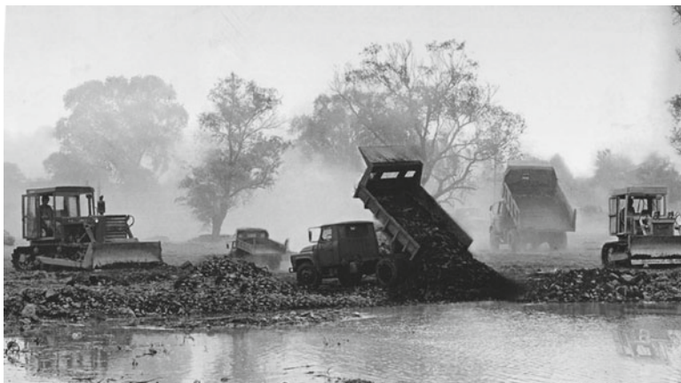
Fig. 3.34 Deposit of coal mining waste on subsided and flooded terrain in the Double H Region, China (From: Huainan Mining Industry (Group) CO., LTD.)
