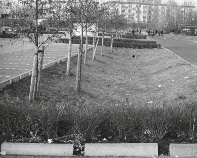
Fig. 2.4 Stormwater runoff storage system (swale) located between car park and market place
