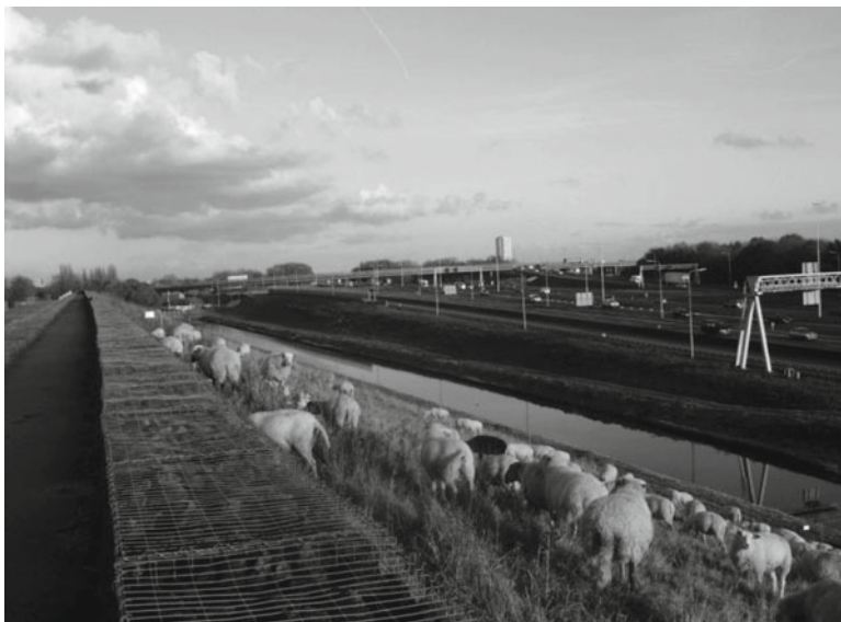
Fig. 5.15 Sound insulating wall filled with encapsulated contaminated substrates close to a motorway in Rotterdam, The Netherlands
