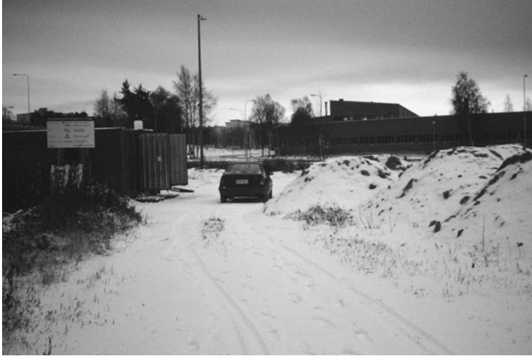
Fig. 6.21 Regeneration pits for the bioremediation of an oil-contaminated soil in cold climatic conditions in Oulu, Finland – the photograph was taken in November when the sun sets at 3 p.m. and the air temperature is -35^{\circ}\text{C}
