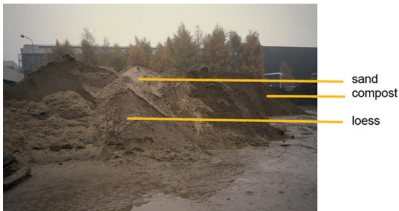
Fig. 4.11 Process of soil mixing for the supply of clean soil: piles of uncontaminated material divided into different texture classes (sand, loess, compost at the back)
