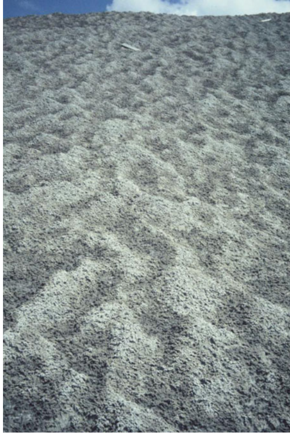
Fig. 3.17 Loose surface at the slope of a salt mining heap in proximity to Hanover, Germany
