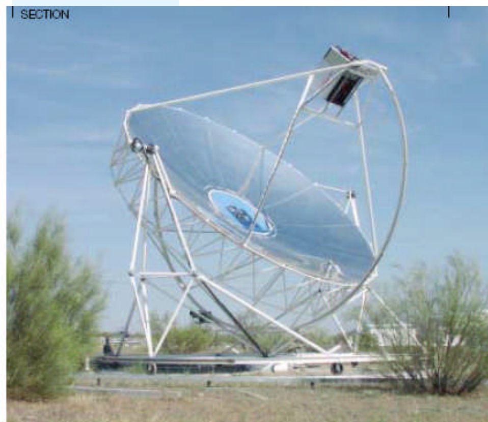
Figure 6 The EURO-DISH parabolic dish concentrator with a Stirling motor-generator in the focal point at the CIEMAT solarthermal test centre Plataforma Solar de Almería, Spain (Source: SBP)
