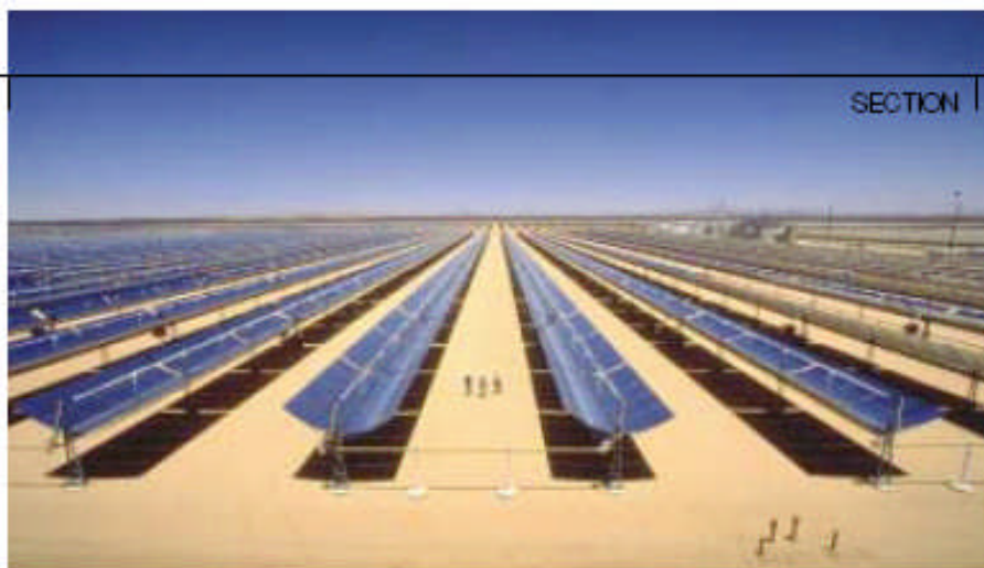
Figure 4 Parabolic trough concentrating solar collector field of the 150 MW ( 5 \times 30 MW) steam cycle solar electricity generating systems at Kramer Junction, California (Source: KJC)
