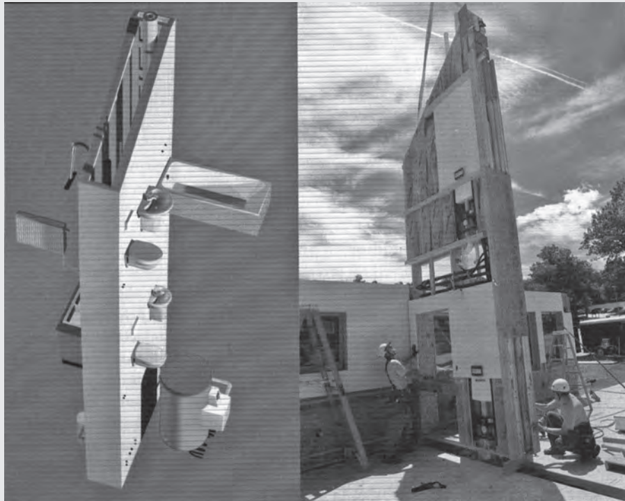
Figure 11.6 Bensonwood Homes separates different components of a building, prefabricating many assemblies in controlled environments. This also controls waste. Courtesy of Bensonwood Homes.
