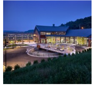
The Roundhouse at Hazelwood Green GBBN Architects
