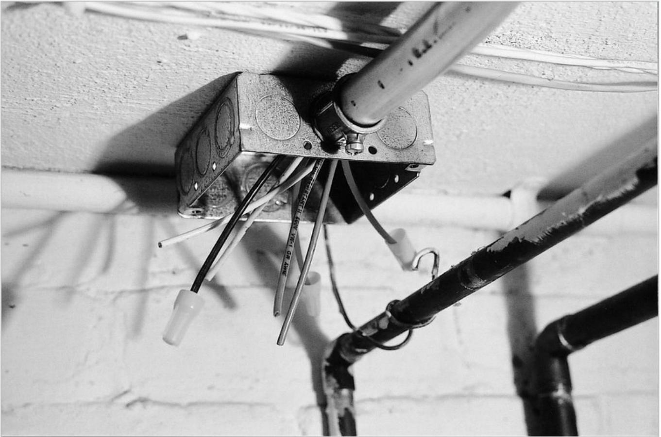
When leaving unfinished electrical wiring projects unattended, simple precautions, such as capping wires, turning off power, or adding warning tape, can prevent injuries.
