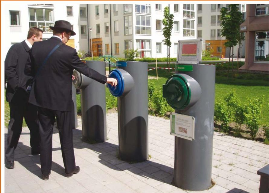
These are envac points at the Hammarby Sjöstad low-carbon housing development in Stockholm, Sweden. Waste is dropped in the inlets – a vacuum system sucks it to the collection terminal where it is sorted. It is a working prototype for a new and sustainable way of living. Image courtesy of Liz Bartlett.
