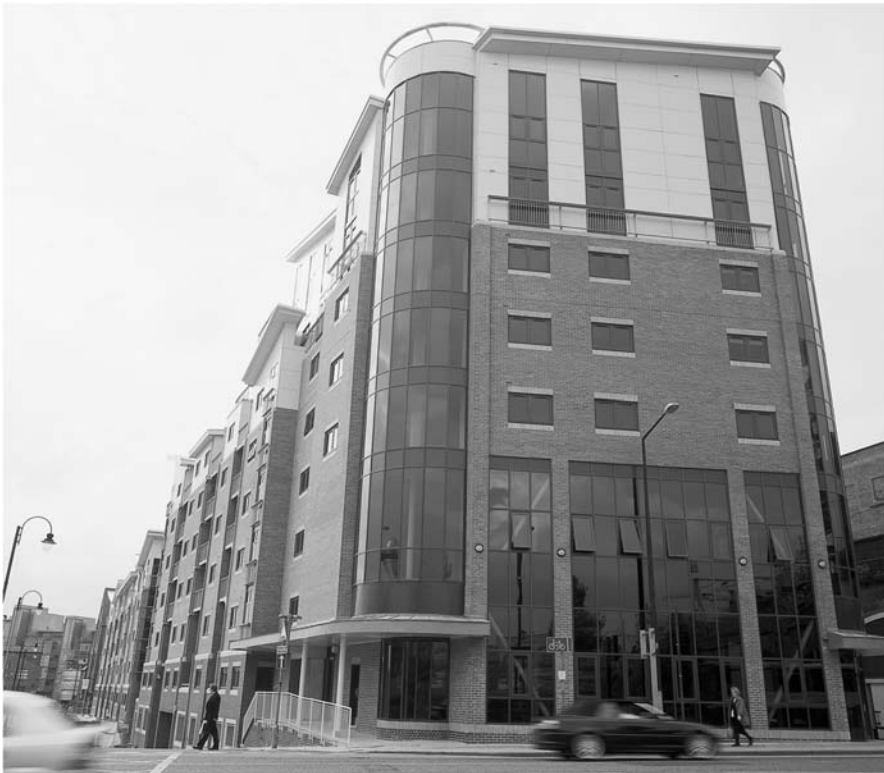
▲ B2 Front of the completed development
