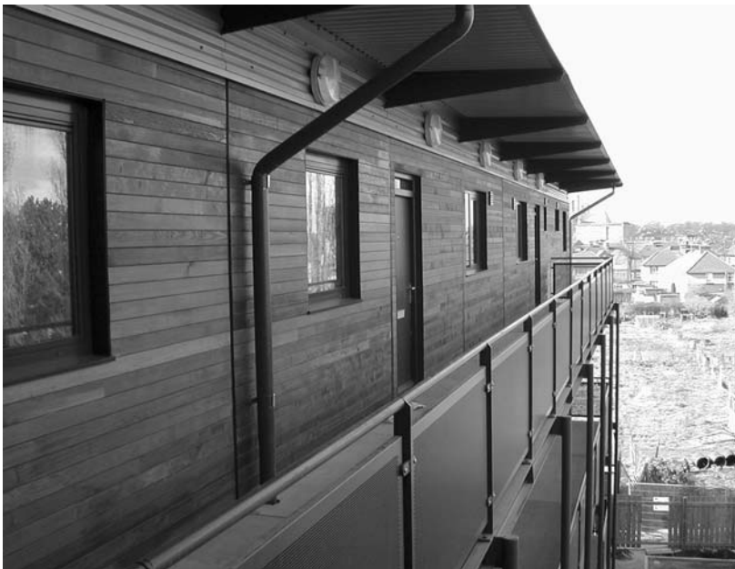
▲ 17 Access balcony passes kitchens and some bedrooms
