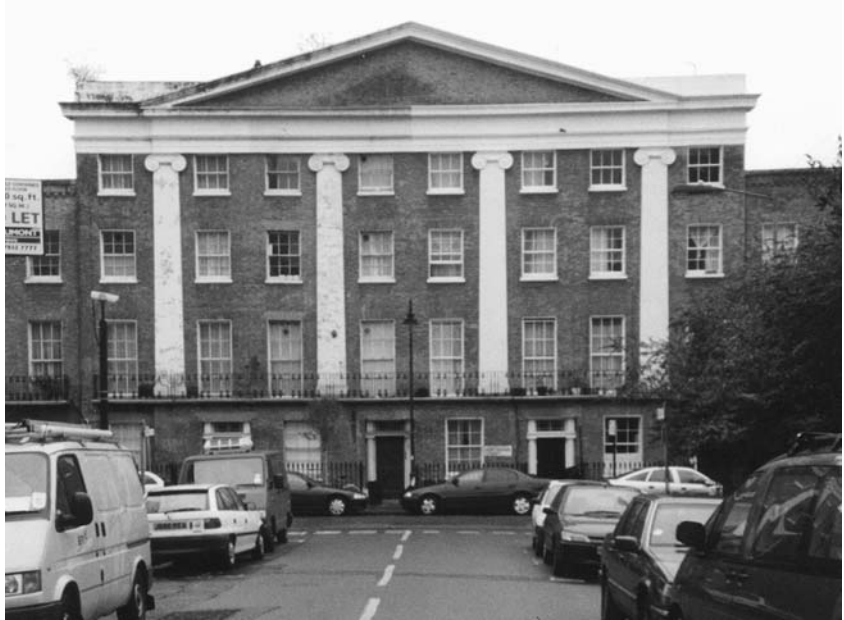
▲ 7.1 Northdown Street, London N1 – Classical formalism. Four houses are designed as one giant portico with each owner given care of a giant pilaster. Even then the entrances are not symmetrical
