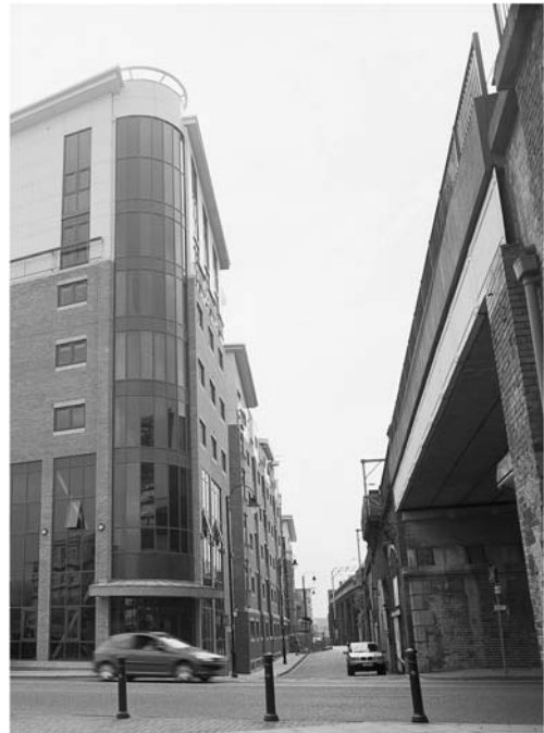
▲ B6 An elevated railway runs along the rear of the site
