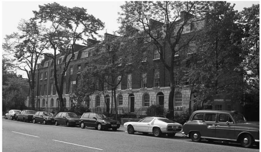
▲ 0.8 Old terraced housing renovated and converted
