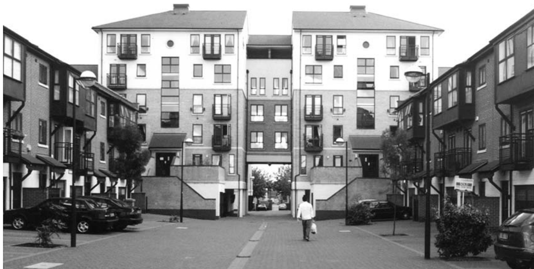
▲ C3 Court of private housing off dock front
