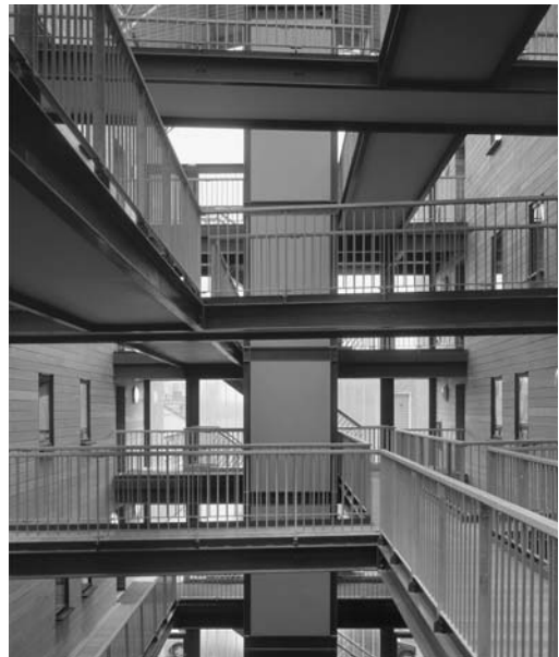
▲ F4 The central space, lift and stairs
