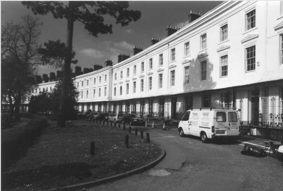
▲ 1.3 Regency housing in Lansdown Crescent
