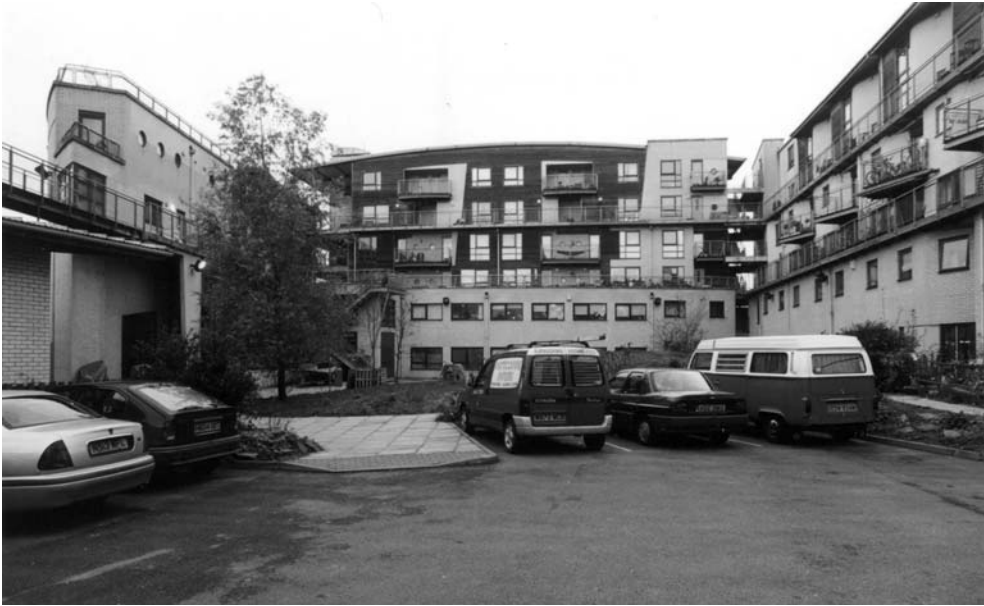
▲ D2 The central courtyard
