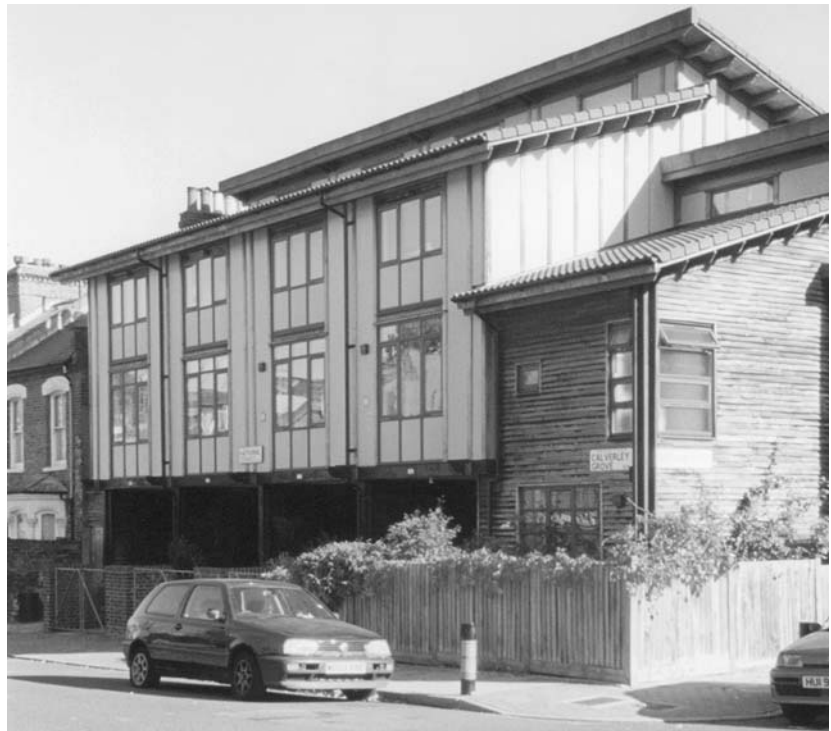
▲ 5.4 Timber-framed terraced houses in North London self-built by residents using the Segal system
