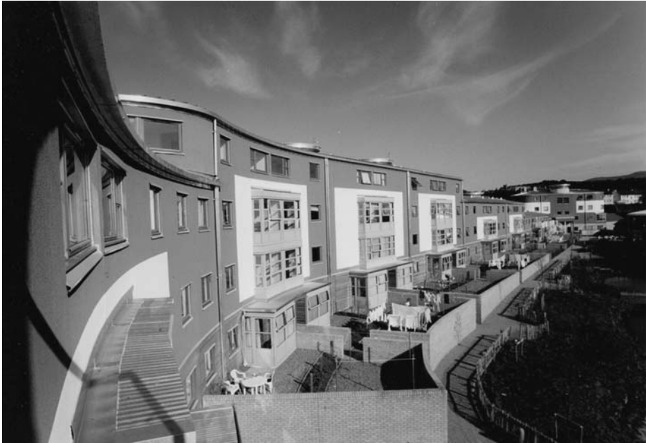
▲ G6 The central space, ponds on the right
