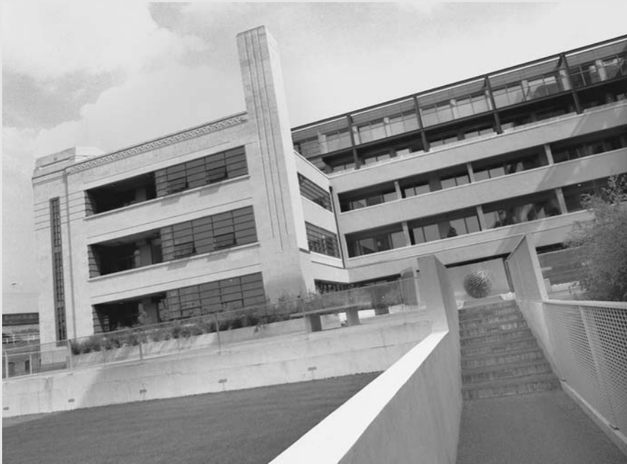
▲ 6.12 The completed project
