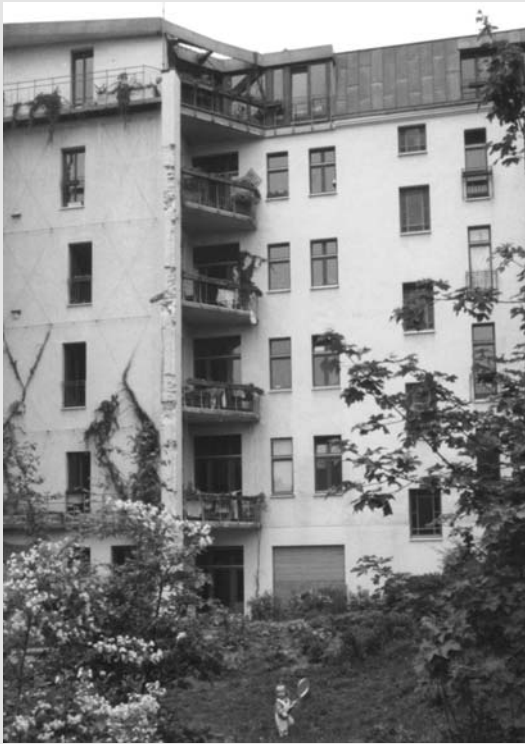
▲ 8.3 Existing housing renovated with courtyard opened up to give light and green space
