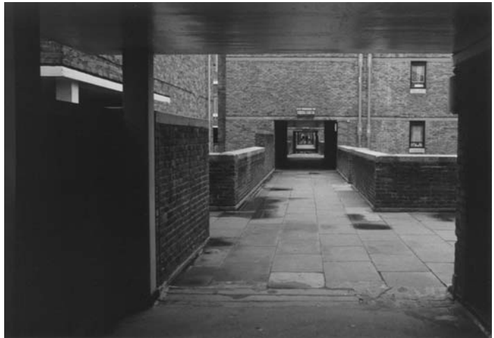
▲ 4.6 North Peckham Estate
