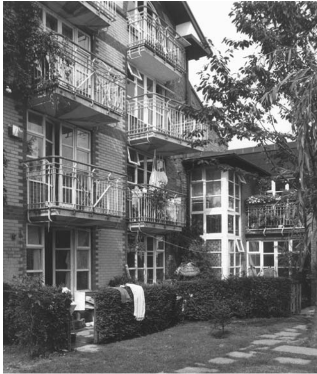
▲ 7.16 Bramley Co-op, West London. This co-op, founded on a squatters group, developed a mixture of family houses, shared houses and small flats for single people. At the centre of the scheme is a communal garden shared by all the residents
