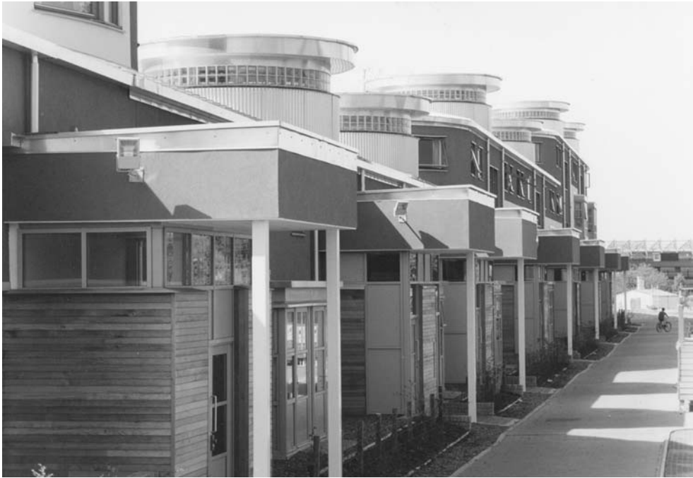
▲ G5 'Passive-stack' vent turrets to staircases
