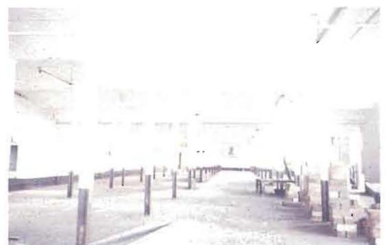
Ditherington Flax Mill, Shrewsbury, England, the world's first iron framed building, erected in 1797.
