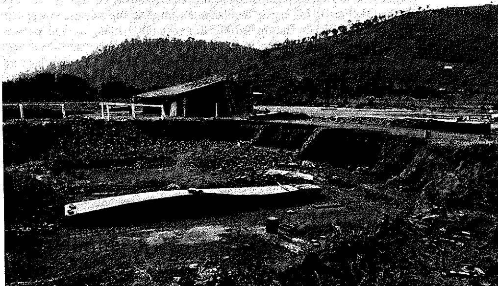
Figure 5.1 A brickyard in highland Guatemala. The plastic clay soils of the valley are excavated and mixed with water, then shaped in rectangular wooden molds to form bricks,
