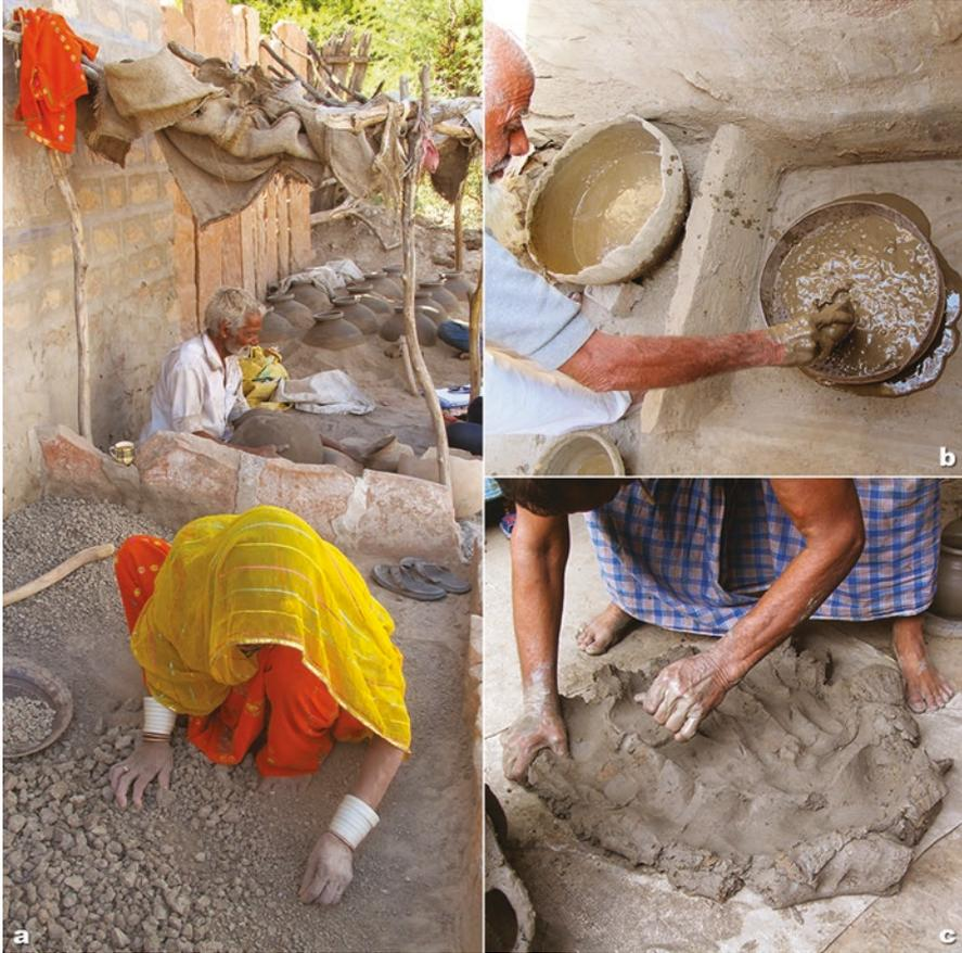
**Fig. 2.7** Removing coarse elements: (a) by hand during the course of fragmentation; (b) with a sieve on liquid clay; (c) by hand during kneading
