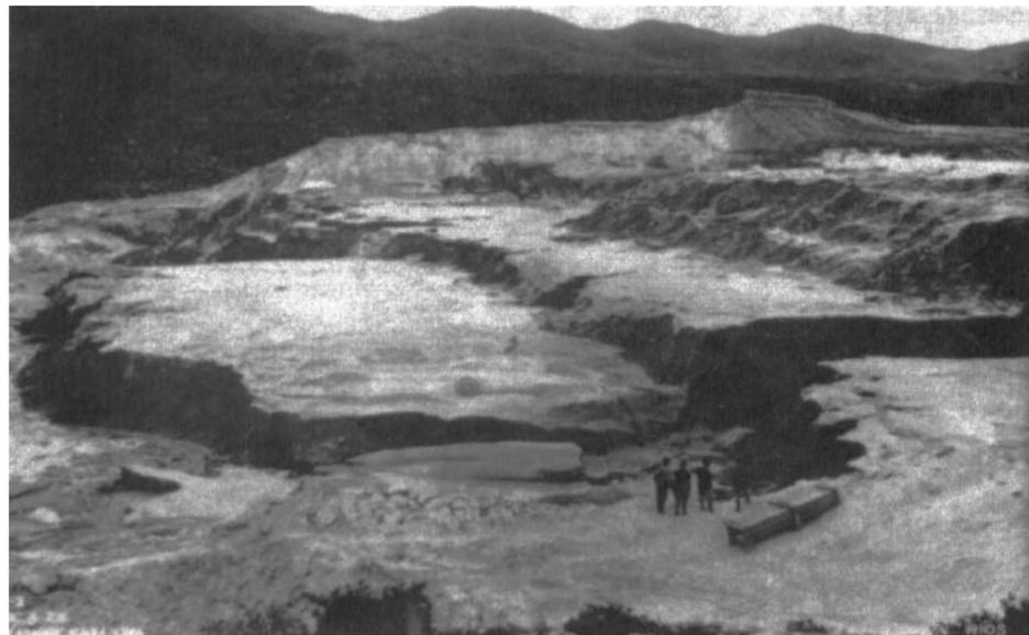
**Figure 3.** Collapse of Barahona Tailings Dam, Rancagua, El Teniente Mine, 1928 [16].
