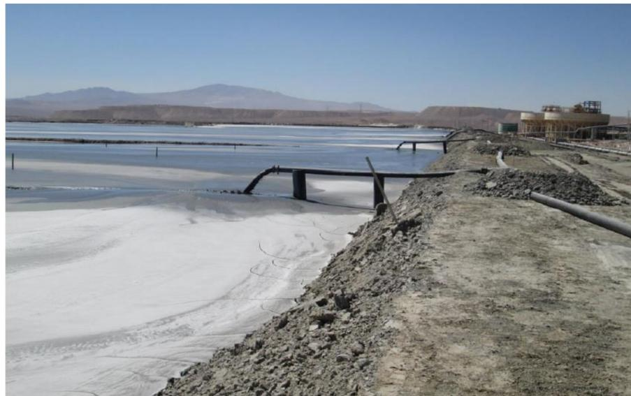
Figure 21. Centinela Tailings Storage Facility, Centinela Mine, thickened tailings technology [8].
