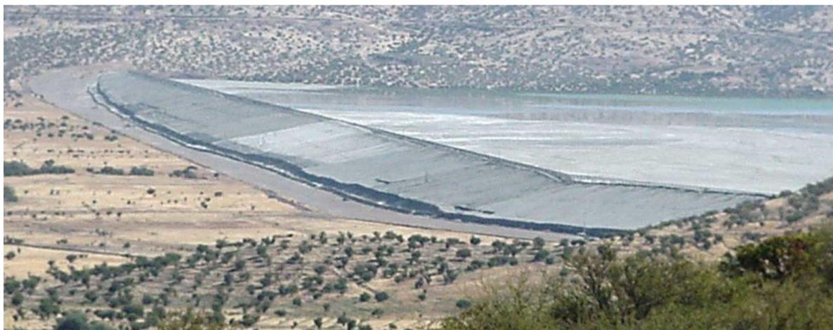
Figure 19. Ovejeria Tailings Dam, Andina Mine, conventional tailings technology [52].
