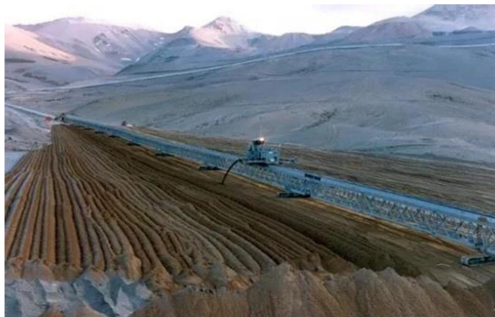
Figure 25. Rako Tailings Storage Facility, La Coipa Mine, filtered tailings technology [47].
