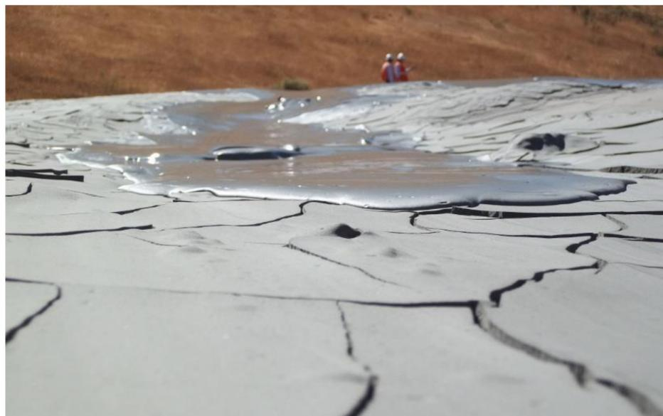
Figure 23. Chinchorro Tailings Storage Facility, Las Cenizas Mine, paste tailings technology [33].
