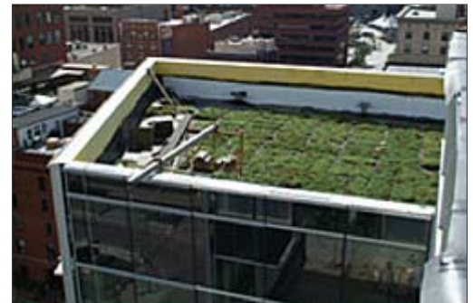
The building's modular green roof system is planted with sedum and will reduce storm water pollution, minimize heat-island effect, and absorb carbon dioxide.
