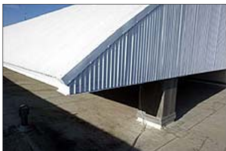
Curved Energy Star® white roof covering the mechanical systems and Energy Star® compliant reflective flat roof
