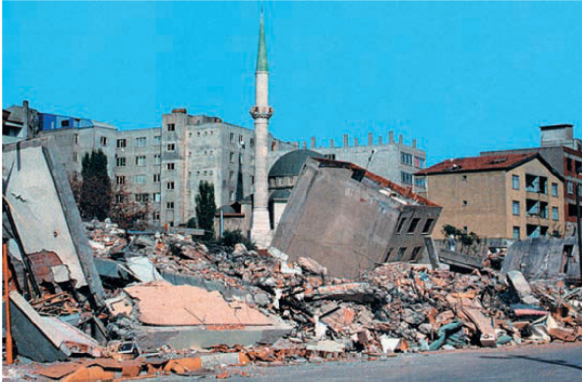
FIGURE 14.17 An earthquake near the town of Izmit in western Turkey in 1999 killed at least 50,000 people and injured an equal number. Poorly constructed buildings collapsed and trapped residents, while stronger structures nearby remained standing.
