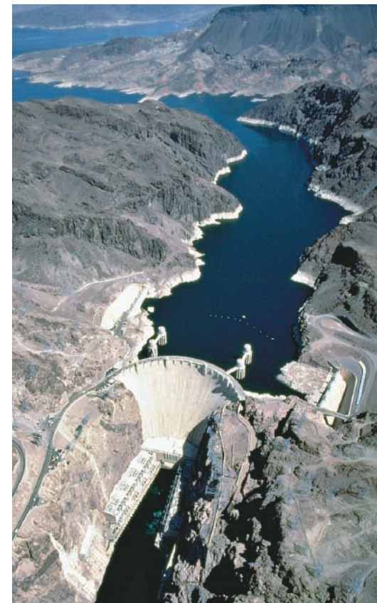
FIGURE 24.13 Hydroelectric power is produced by channeling dammed rivers through turbines inside dams such as this one. Hoover Dam impounds the Colorado River to form Lake Mead in Nevada and Arizona. (Lowell Georgia/Photo Researchers, Inc.)
