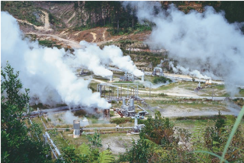
FIGURE 24.15 Geothermal energy stored in heated groundwater is extracted in facilities such as this one in New Zealand to generate electricity.
