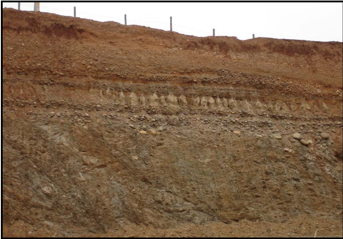
Figure 11. Huentelauquén road cut. From top to bottom: Soil of about 100 cm depth, diverse origin stratified deposit and Silurian Phyllites from the Choapa metamorphic complex
